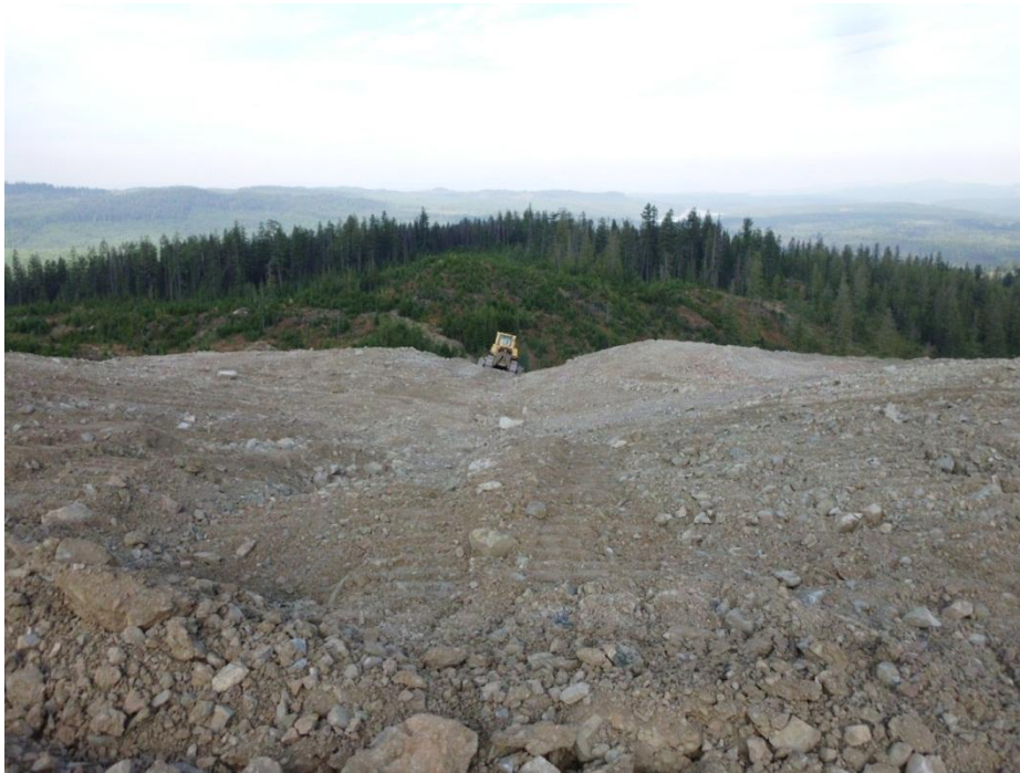
Figure 1. Creation of a swale on the NBD
