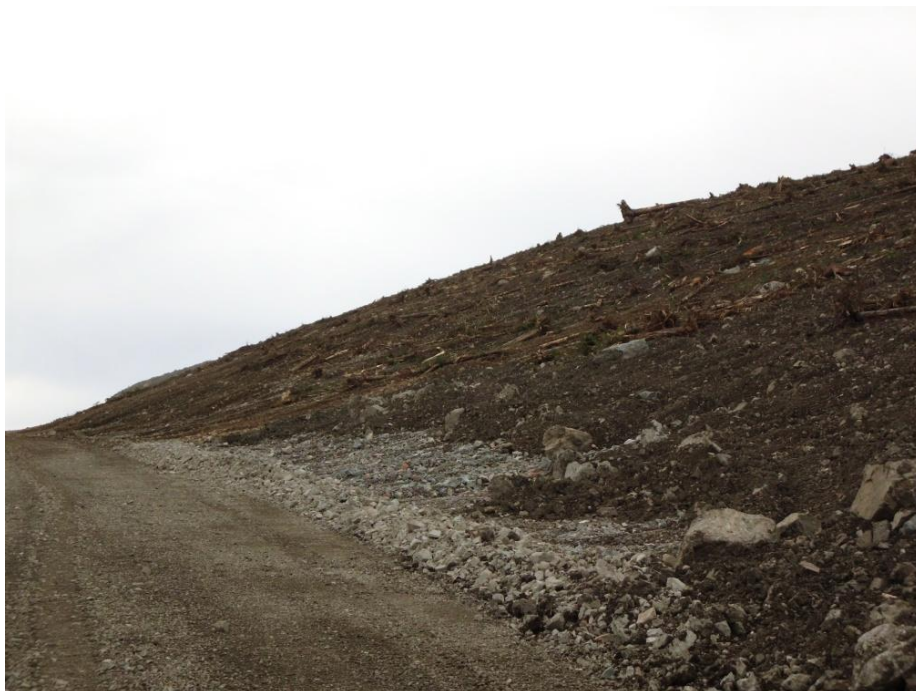
Figure 3: Coarse Woody Debris placed on North Bell Dump
