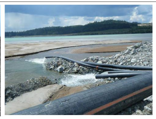
Photo 15: Perimeter seepage pond discharge into the TSF.
