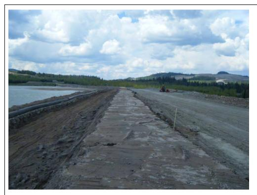
Photo 13: Looking northwest along the perimeter embankment (Zones U, S, F, T and C from left to right).
