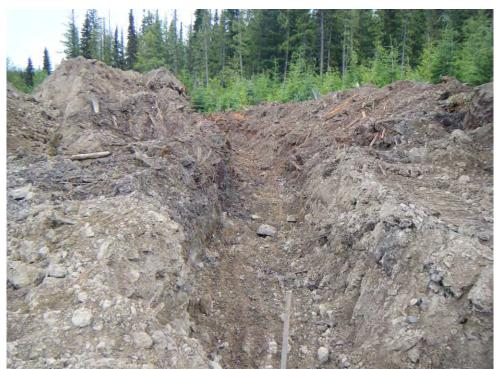
Photo 1: Relocation of the diversion trench near corner 4.
