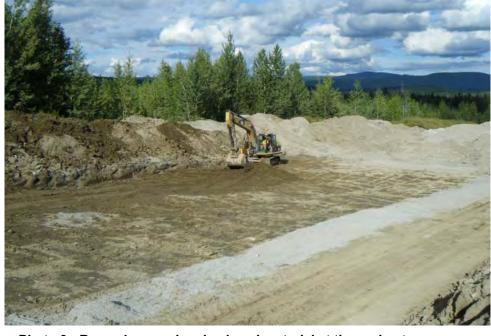
Photo 9: Removing previously placed material at the perimeter embankment to expose competent native till.
