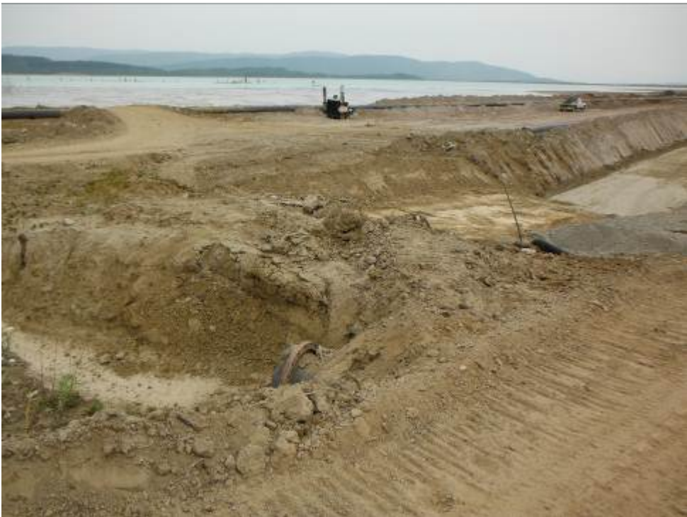
Photo 2: South embankment abutment tie-in
