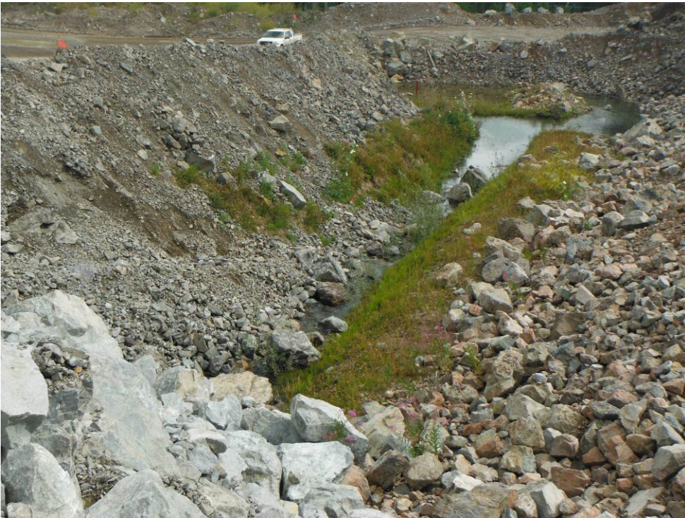
Photo 13: Perimeter drain discharge as impacted by haul road connection.
