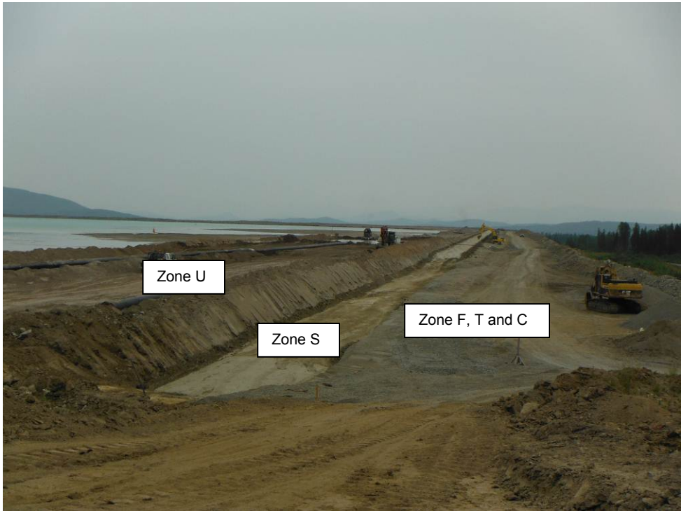
Photo 1: South embankment fill placement near corner 4.
