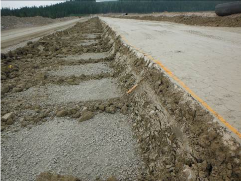
Photo 4: Compacted and trimmed Zone S (glacial till) along South embankment
