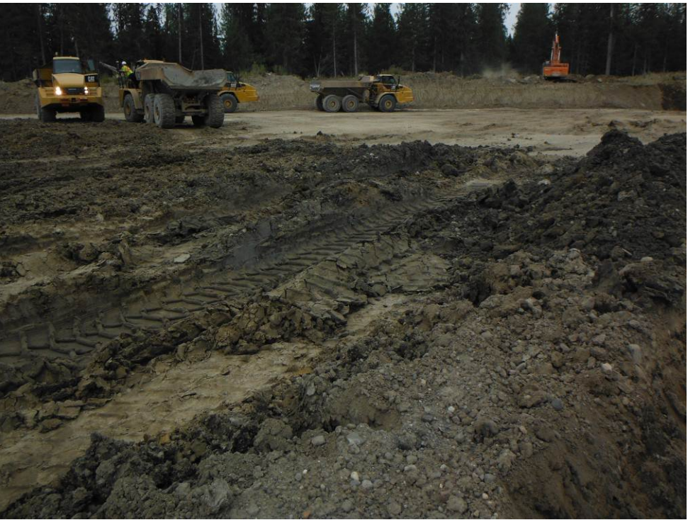
Photo 20: 'Punchy' GLU material, unsuitable for use as Zone S core.
