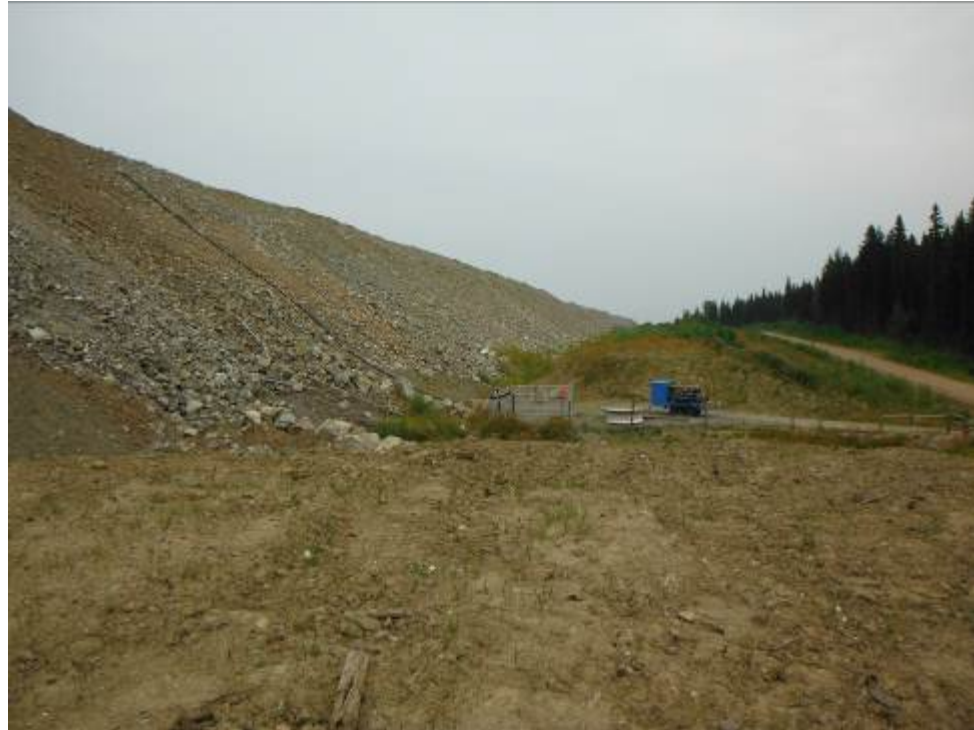
Photo 6: South embankment Zone C (downstream shell), looking west. Drain pumpback to impoundment shown.
