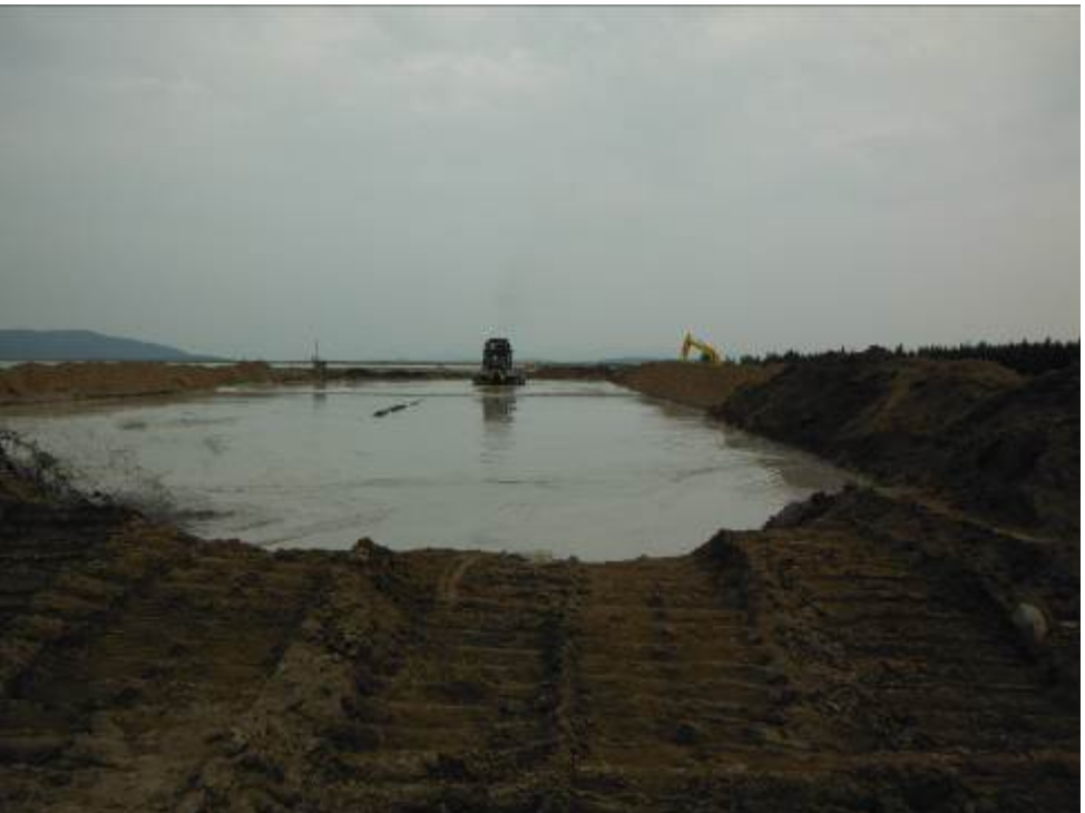
Photo 3: Zone U sand cell construction along South embankment.
