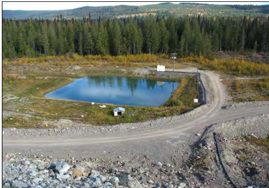
PHOTO 2 – Perimeter Embankment Seepage Collection and Recycle Pond.
