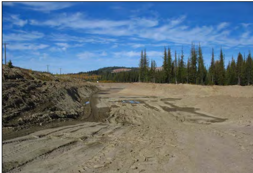
PHOTO 4 – Glacial Till borrow Downstream of Perimeter Embankment.
