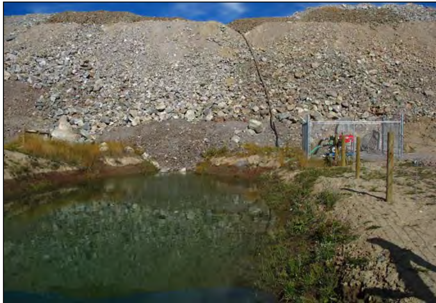
PHOTO 14 – South Embankment Seepage Collection and Recycle Pond.
