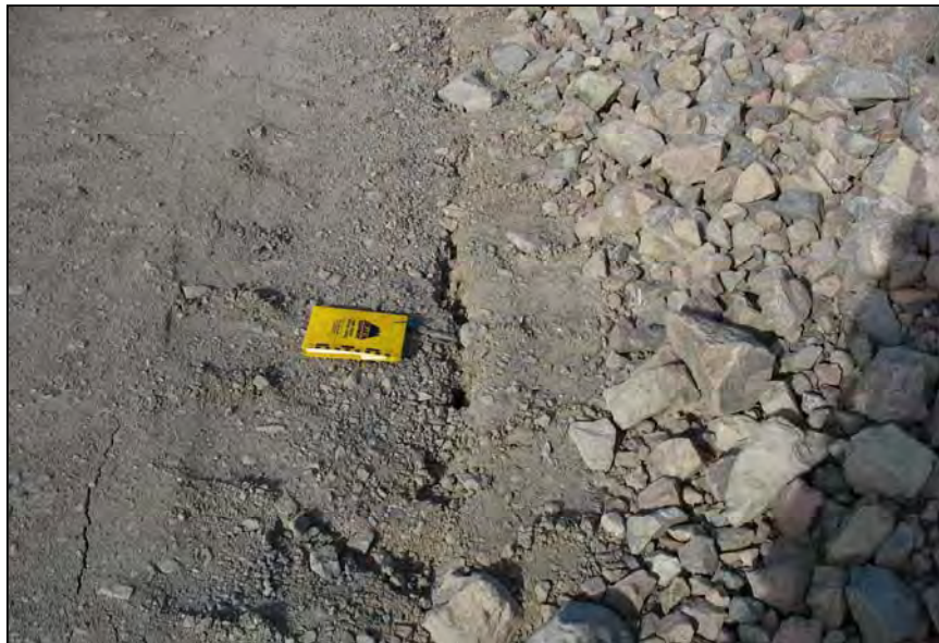
PHOTO 6 – Tension Crack at the Perimeter Embankment.
