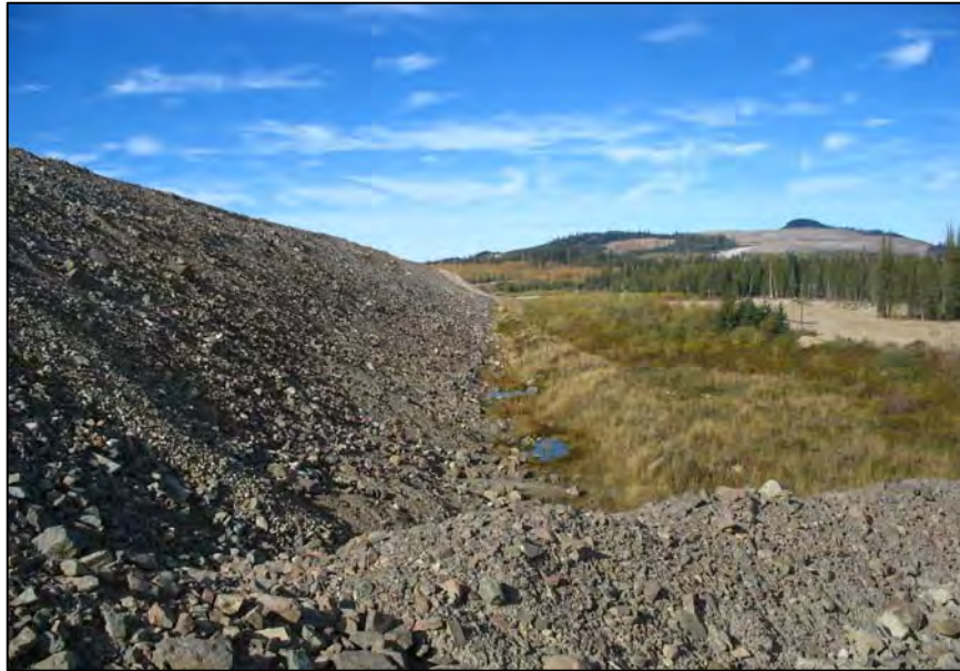
PHOTO 7 – Downstream Slope of Perimeter Embankment.
