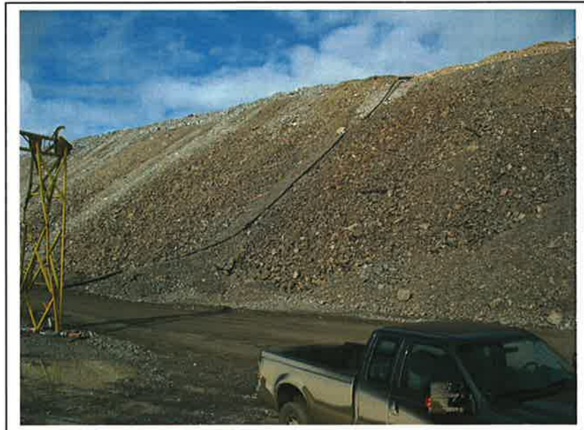
PHOTO 6 – Main Embankment Seepage Pond Return Pipe
