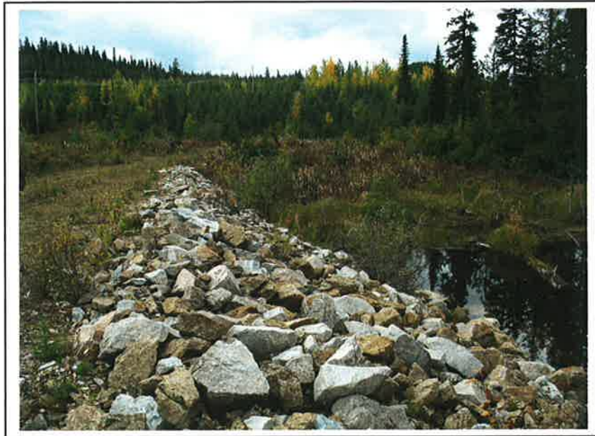
PHOTO 17 – South Bootjack Dam
