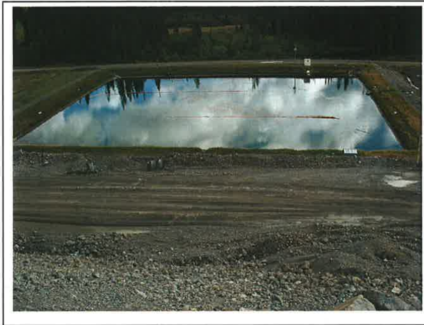
PHOTO 5 – Main Embankment Seepage Pond
