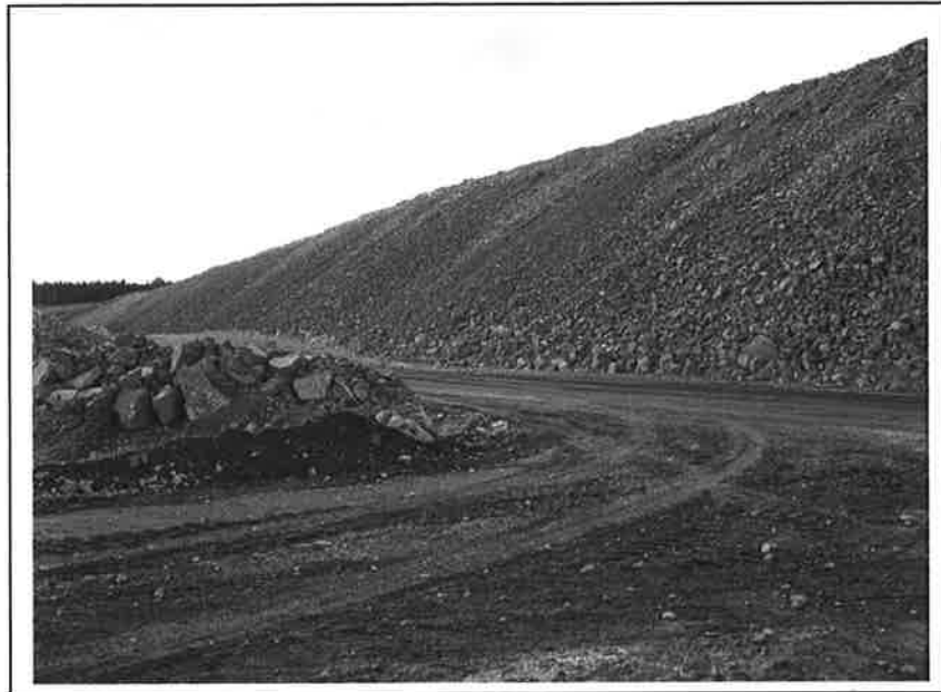
PHOTO 7 – Main Embankment looking west
