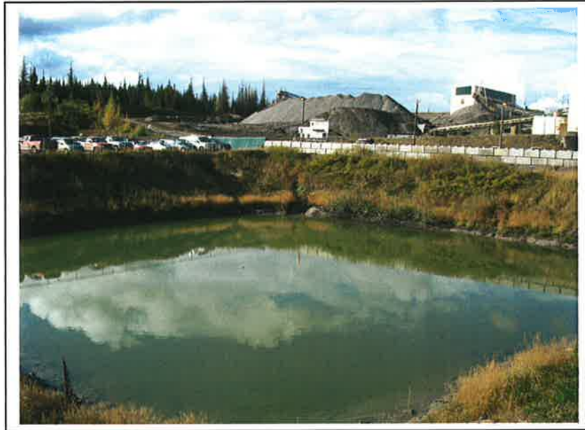
PHOTO 13 – Mill Site Sump
