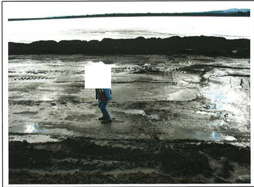
PHOTO 11 – Recently completed Sand Cell
