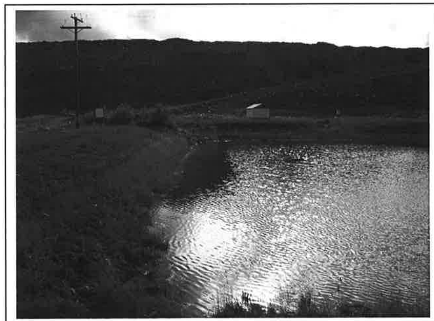
PHOTO 8 – Perimeter Embankment looking south, showing access ramp to PE seepage pond
