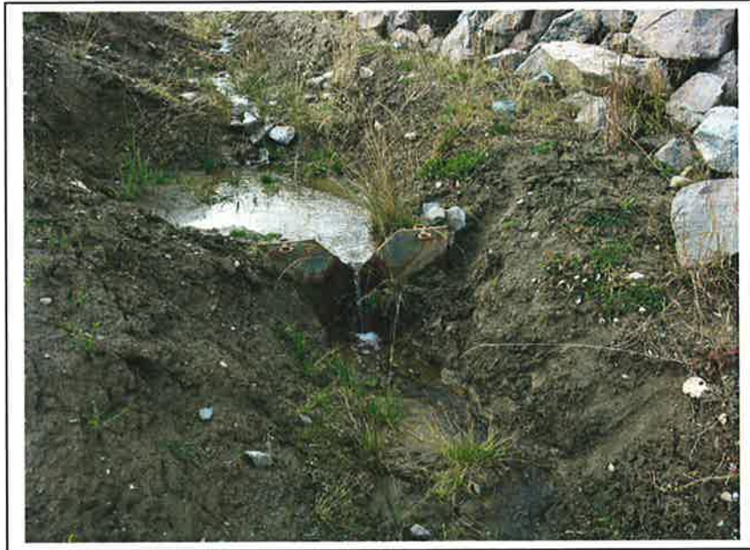
PHOTO 3 – Main Embankment Foundation Drain flows from the ME/SE Corner.
