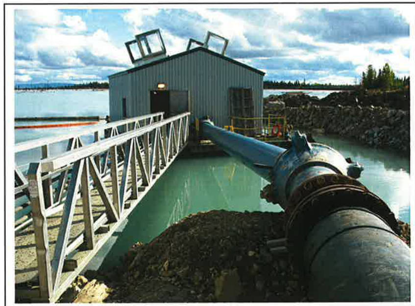
PHOTO 12 – Pump barge and reclaim pipeline
