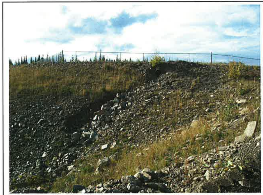
PHOTO 14 – Mill Site Sump Emergency overflow
