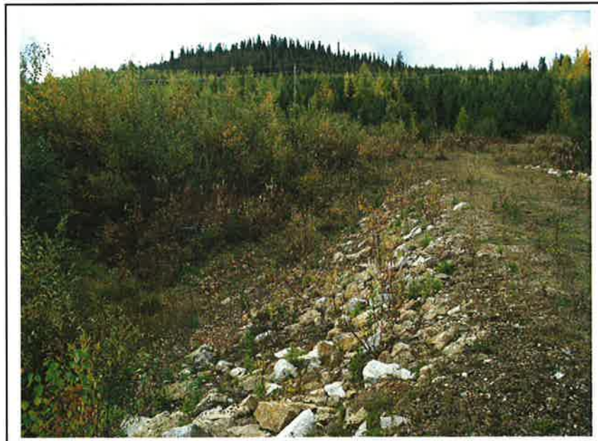
PHOTO 18 – South Bootjack Dam
