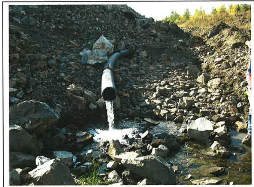
PHOTO 4 – Perimeter Embankment Toe Drain flow running clear
