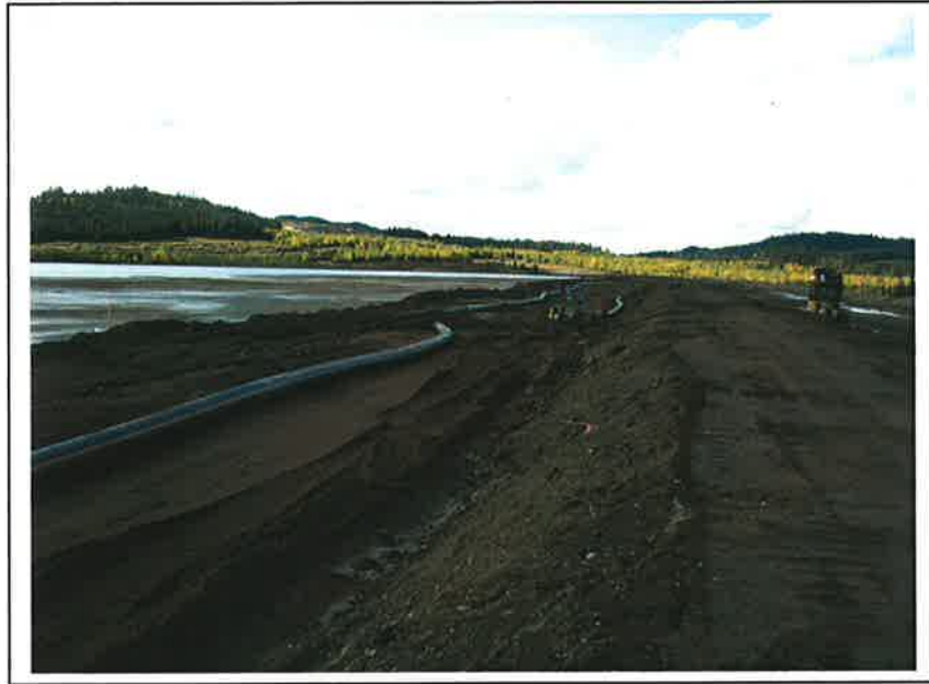
PHOTO 9 – Perimeter Embankment Zones U and S. The Zone U on the left was constructed using tailings sand cells.
