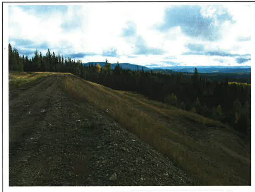
PHOTO 16 – Southeast Sediment Pond Downstream Slope
