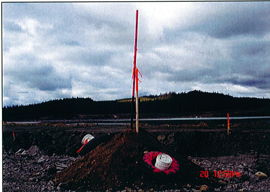
PHOTO 10 – Buckets and fluorescent poles act as protective measures to prevent damage to the new piezometers
