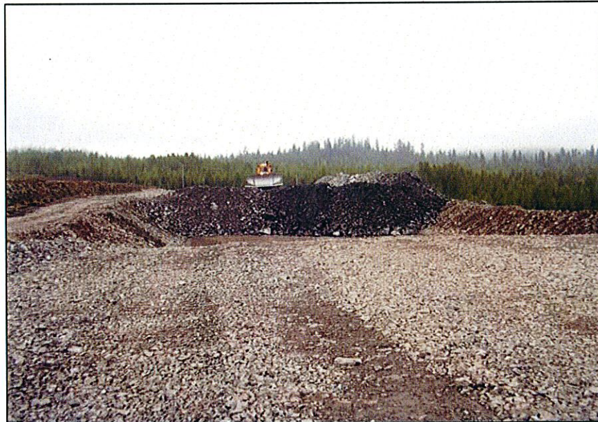
PHOTO 50 – Placement of Zone C in three meter lifts along the Perimeter Embankment.
