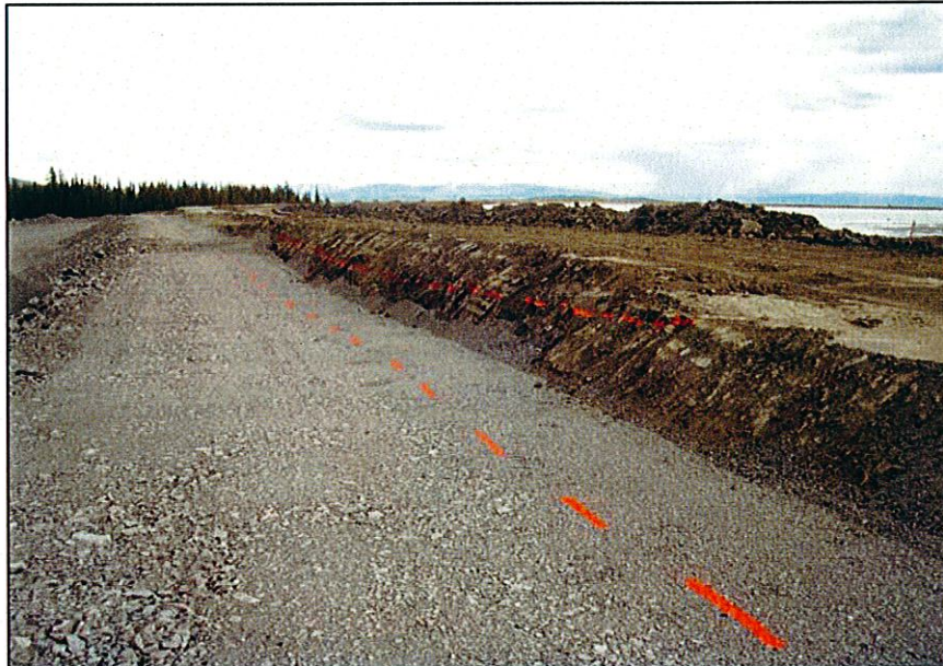
PHOTO 52 – Markings showing the 'hoe' operator exactly where to place the Zone F material against the Perimeter Embankment
