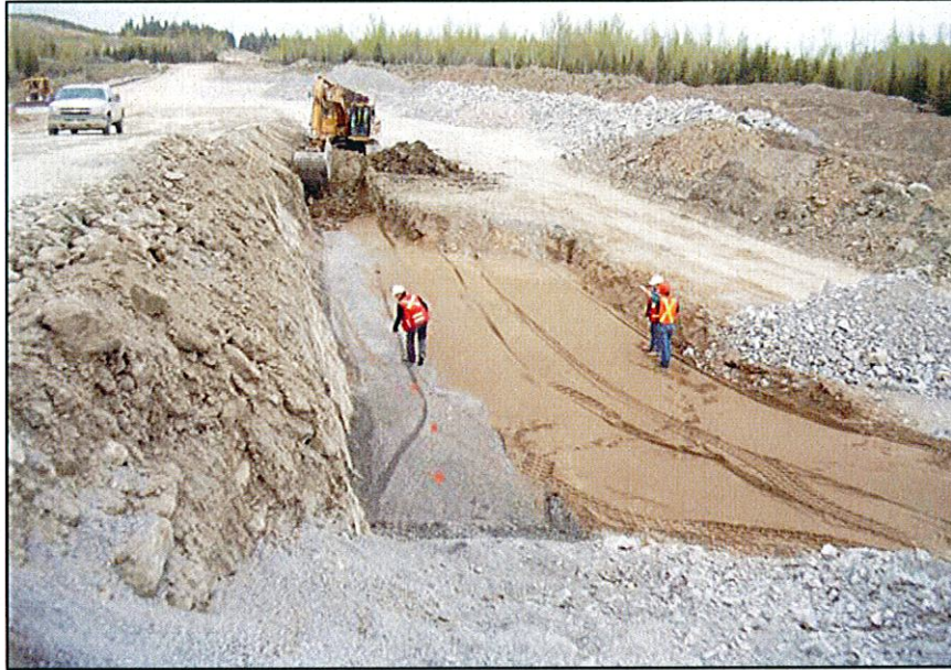
PHOTO 51 – Excavating to 'competent till' north end of the Perimeter Embankment. The area downstream of the Zone F region was excavated to original ground, and Zone FT was placed overtop, after which Zone T was placed.
