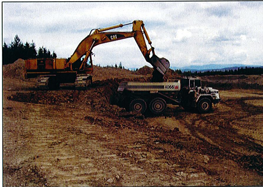
PHOTO 38 – Loading till from Borrow Area No. 4
