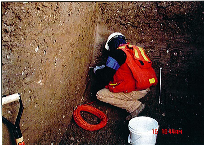
PHOTO 6 –Piezometer Installation
