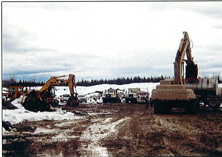
PHOTO 32 – Base of contractor Lake Excavating Ltd.
