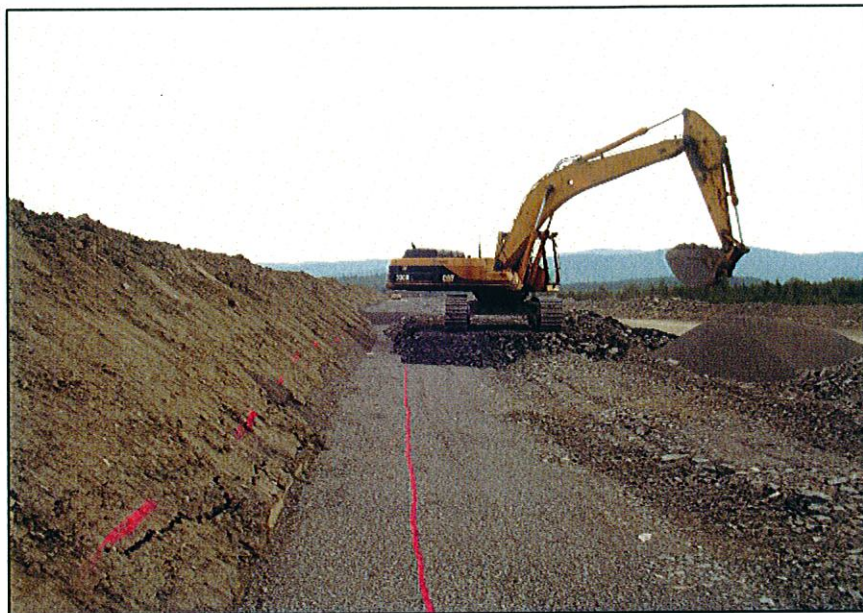
PHOTO 45 – Placing Zone T material along the South Embankment, leaving a one meter section for the Zone F.
