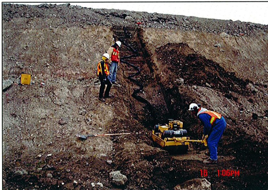
PHOTO 8 – Piezometer Installation in the South Embankment
