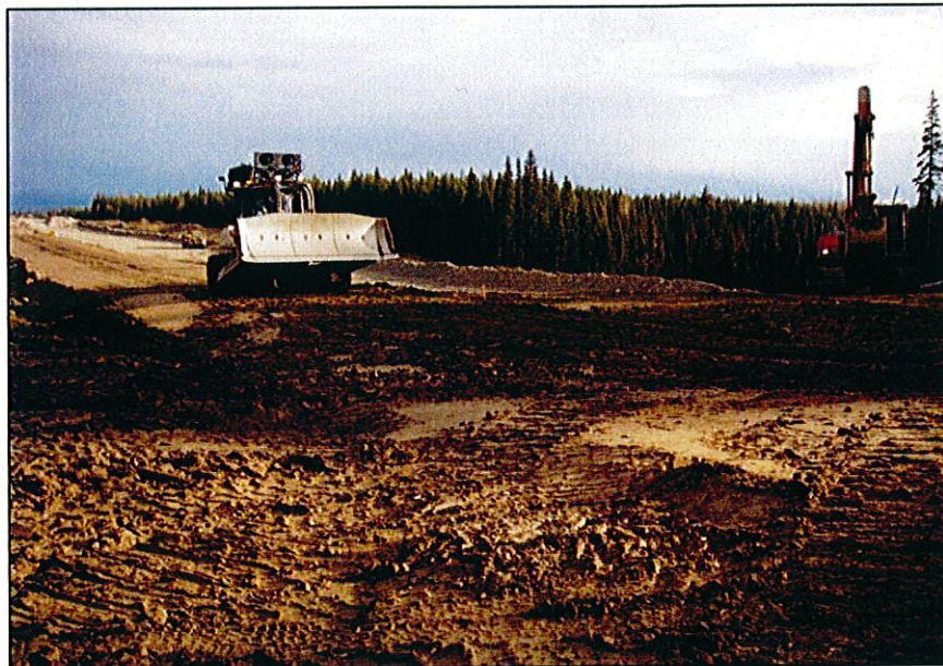
PHOTO 47 – Placement of Zone S material on the South Embankment, the last section to be brought up to elevation 951 m with Zone S.
