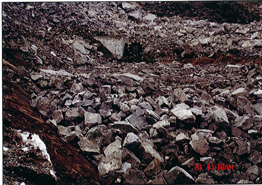
PHOTO 21 – The discharge point of the steel pipe
