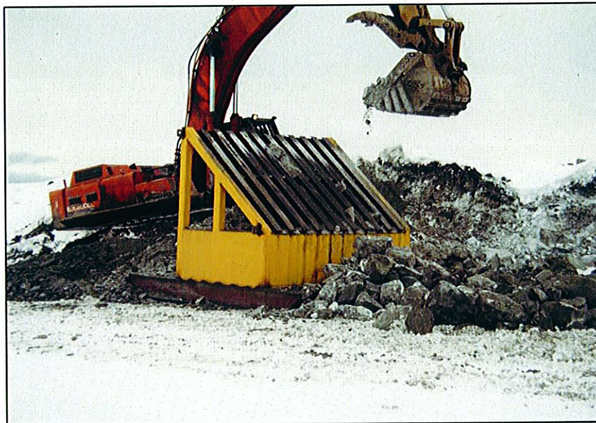
PHOTO 22 – Using the 'Grizzly' to filter the Zone T material, removing rocks greater than six inches in diameter
