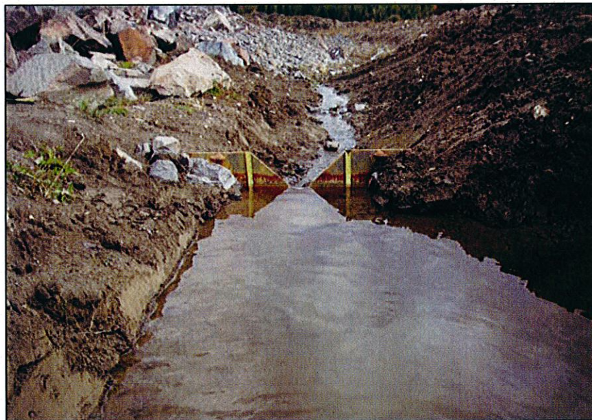
PHOTO 34 – Tape measures installed at the Main-South Embankment corner weir to provide an efficient means of determining the height above the V-notch.
