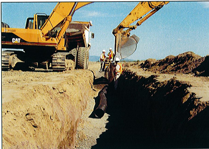
PHOTO 14 – Zone F backfill around the upstream toe drain
