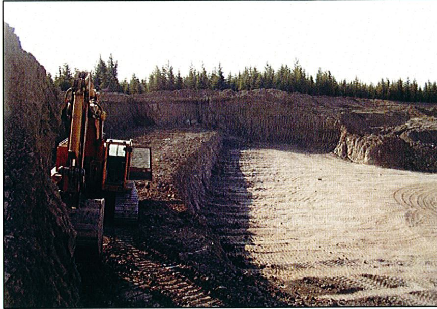
PHOTO 37 – Taking till from Borrow Area No. 3
