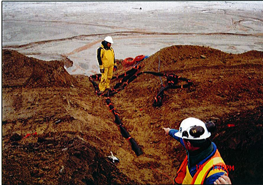
PHOTO 7 – Tailings Piezometer Installation in the Perimeter Embankment
