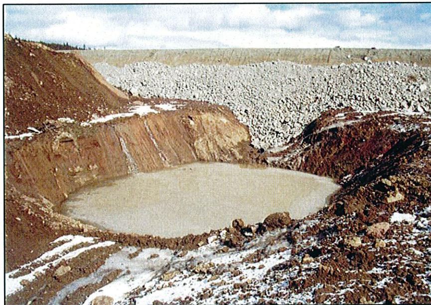
PHOTO 28 – Larger view of South Embankment sump.
