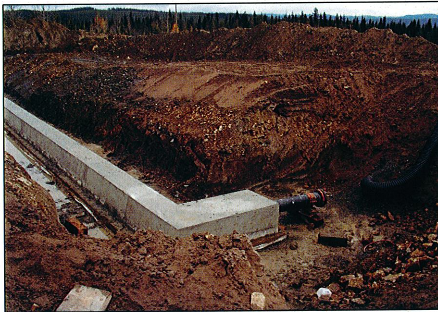
PHOTO 20 – The upstream toe drain and steel pipe prior to connection
