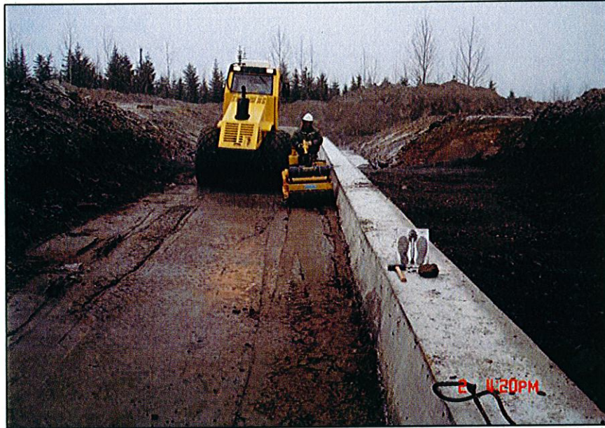
PHOTO 19 – Using the smaller packer to compact the Zone S right up against the encasement, and the 10-tonne vibrating drum roller for the remaining area
