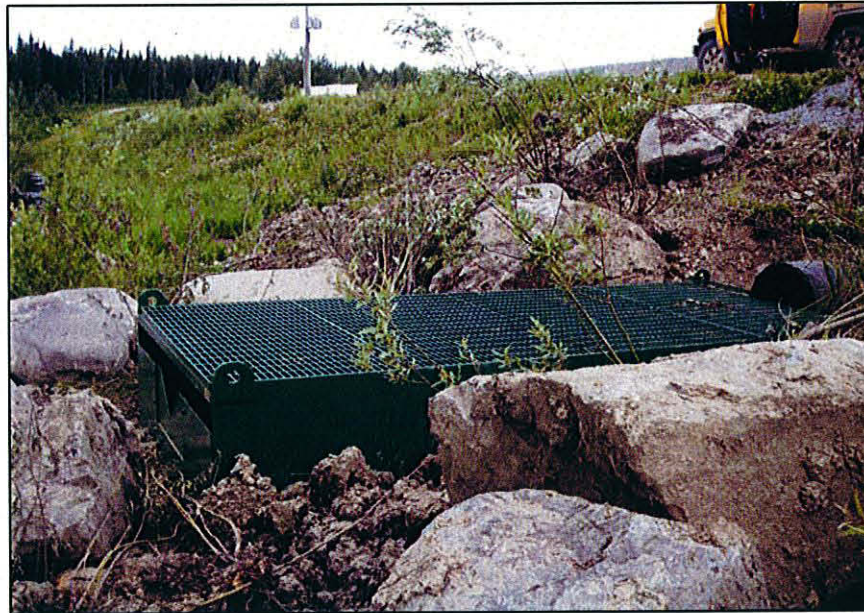
PHOTO 36 – The level weir box backfilled with Zone F and Zone S.
