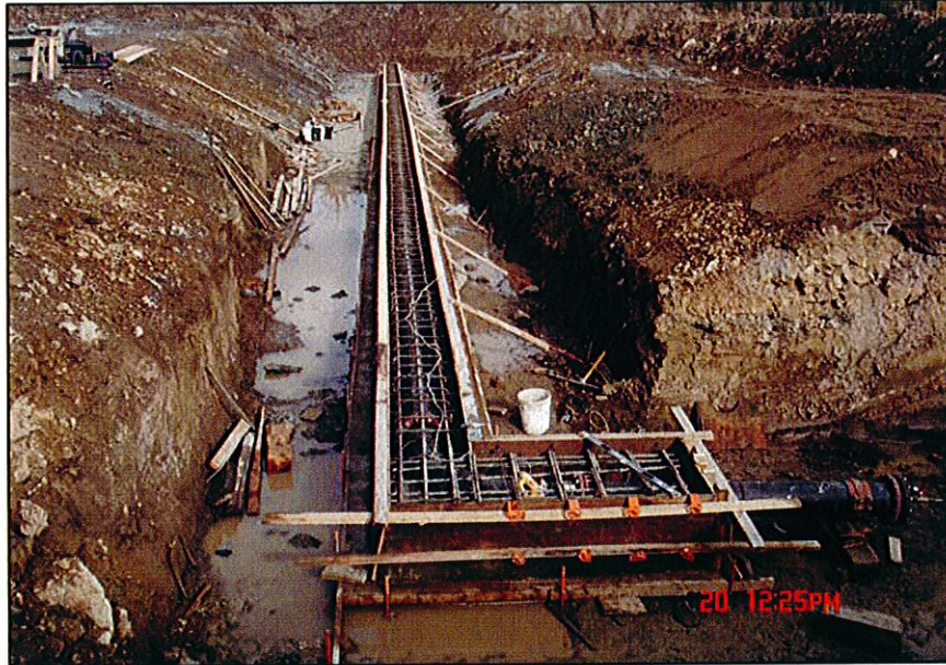
PHOTO 17 – Completed formwork with rebar, ready for concrete pour
