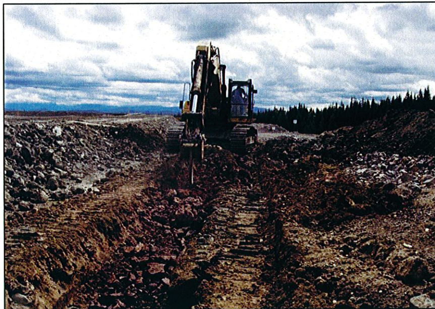
PHOTO 40 – Excavating a ditch for the South Embankment foundation drain
