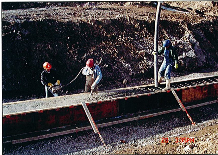
PHOTO 18 – Pouring the concrete to form the encasement
