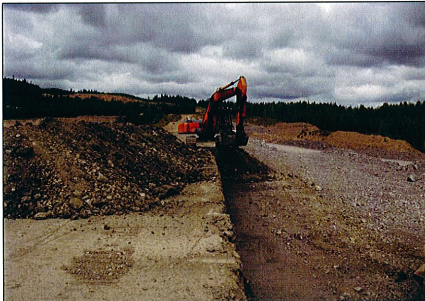
PHOTO 44 – Excavating to competent till for Zone F to be placed against.
