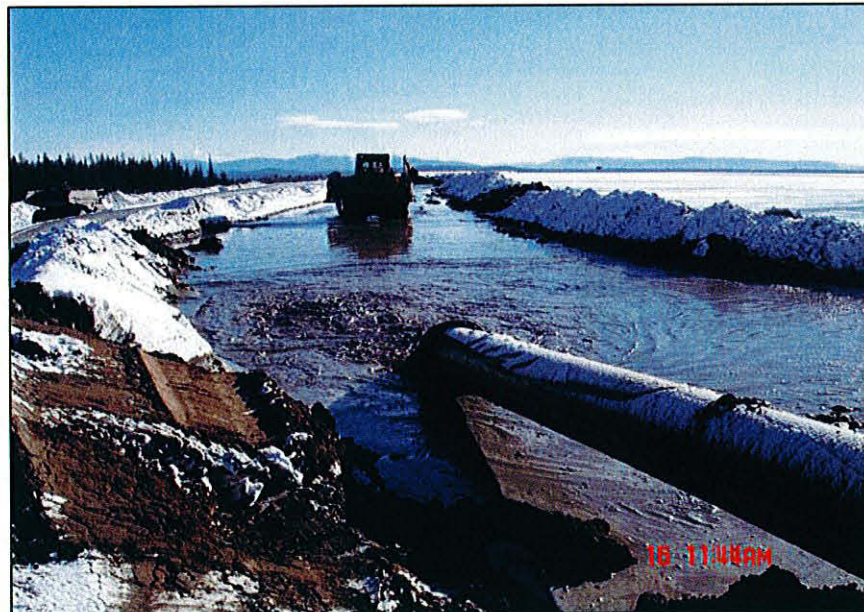
PHOTO 4 – Sand cell production along the Perimeter Embankment
