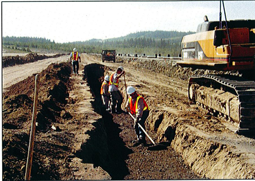
PHOTO 13 – Contractors leveling the Zone F material prior to placement of the Perimeter Embankment Upstream Toe Drain
