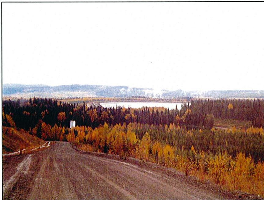
PHOTO 54 – The Mount Polley Tailings Storage Facility.
