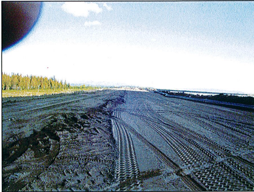
PHOTO 17 – Completed sand cell on the Perimeter Embankment.
