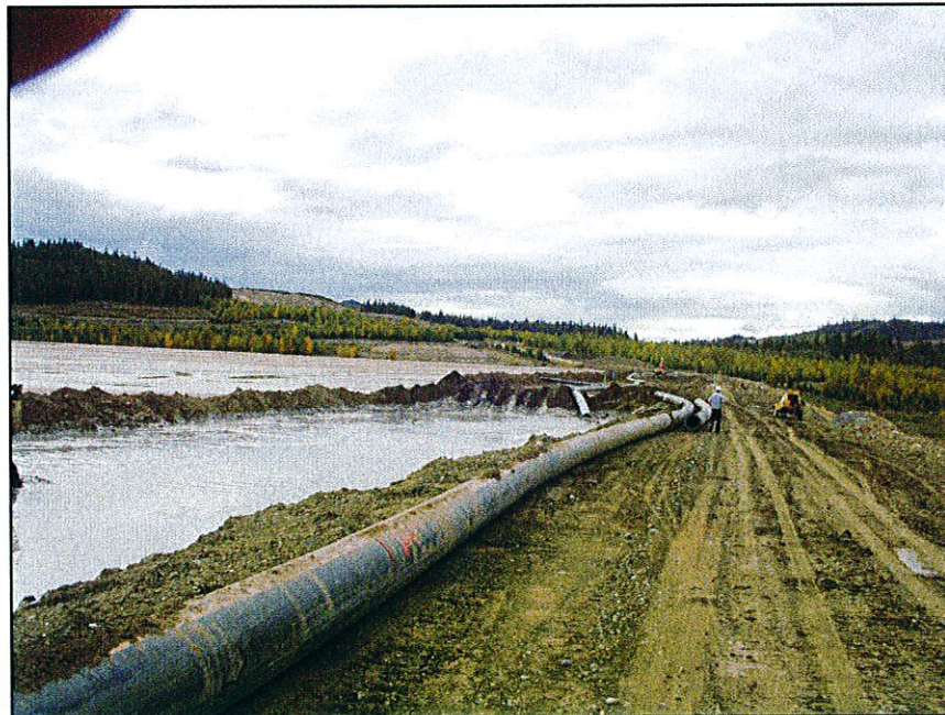
PHOTO 16 – Sand cell on the Perimeter Embankment. Tailings are discharged at the far end and exit into the TSF through culverts installed at the opposite end of the cell.
