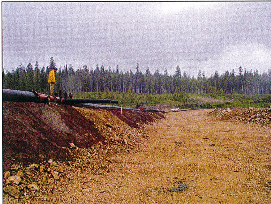
PHOTO 8 – South Embankment sand cell.
