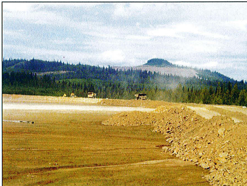
PHOTO 29 – Perimeter Embankment looking up towards the mine.
