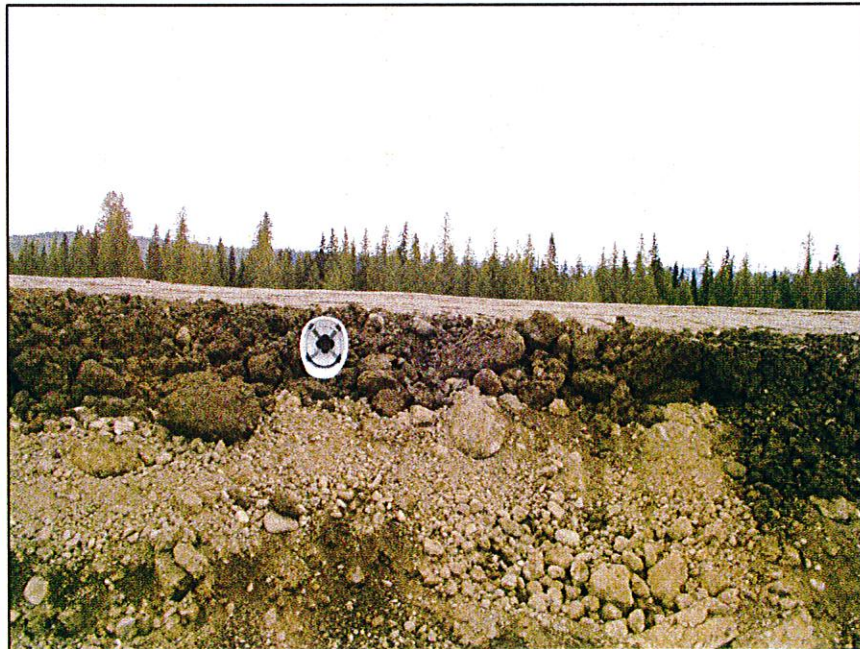
PHOTO 26 – 0.3 m lift of Zone S placed on the Perimeter Embankment.
