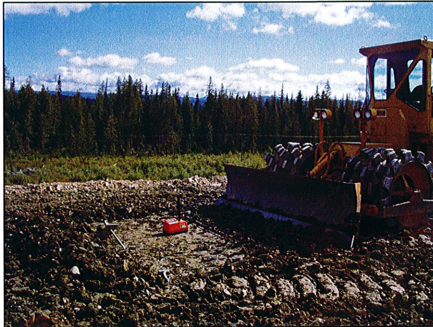
PHOTO 23 – Nuclear densometer testing on the Perimeter Embankment.
