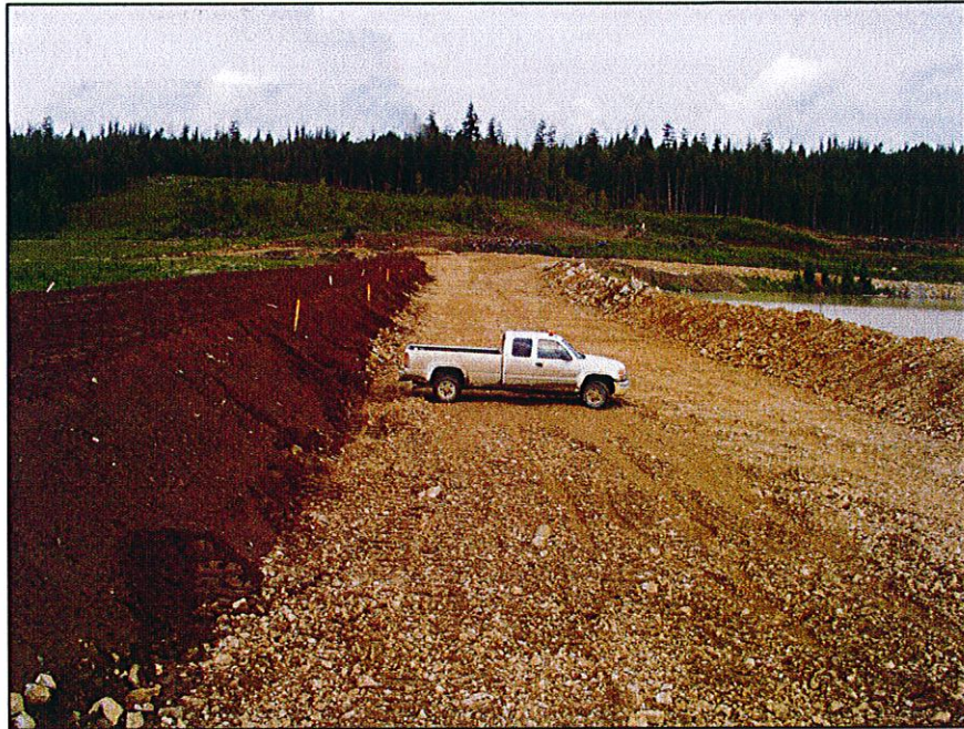
PHOTO 7 – South Embankment after the Stage 4 CBL was placed.
