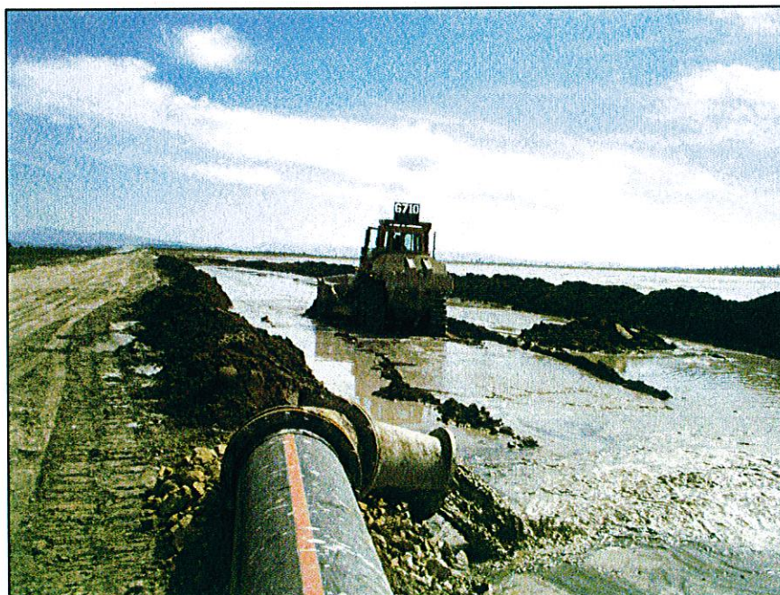
PHOTO 14 – Sand cell on the Perimeter Embankment.
