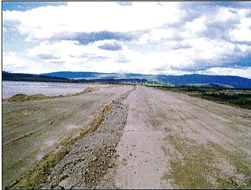
PHOTO 31 – Completed Zone U and Zone S lift on the Main Embankment.
