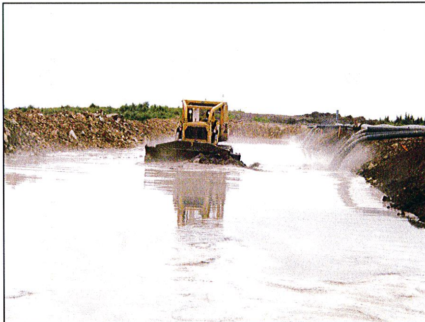
PHOTO 10 – Using a dozer in the sand cell at the South Embankment to distribute and compact the tailings sand.
