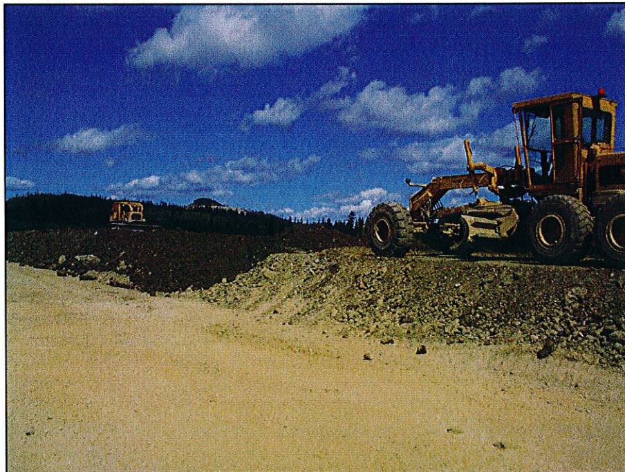
PHOTO 22 – Placing till on the Perimeter Embankment.
