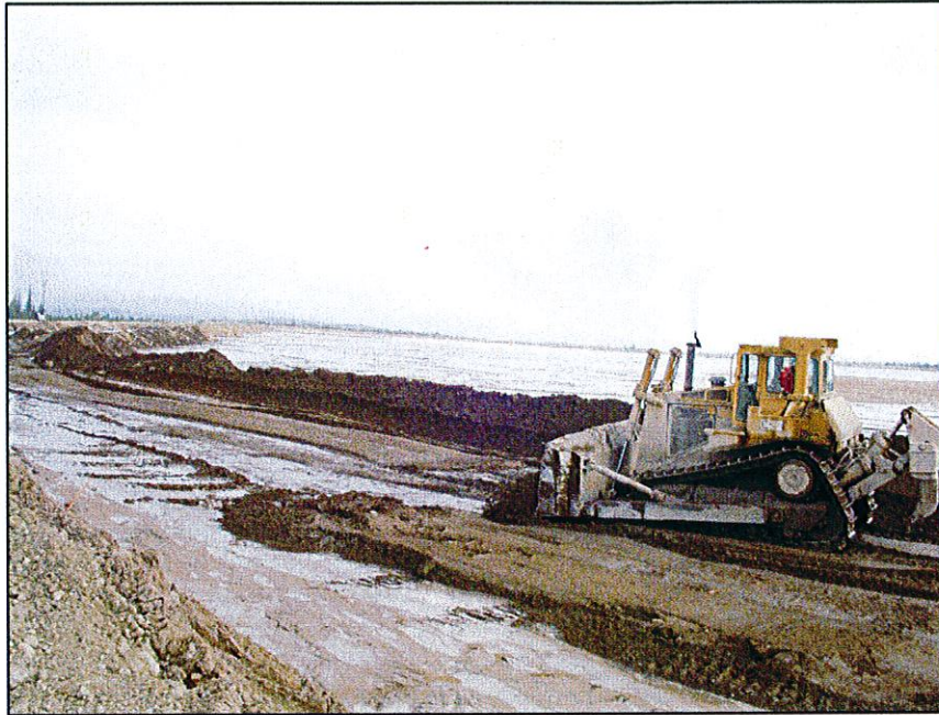
PHOTO 15 – Sand Cell on the Perimeter Embankment.
