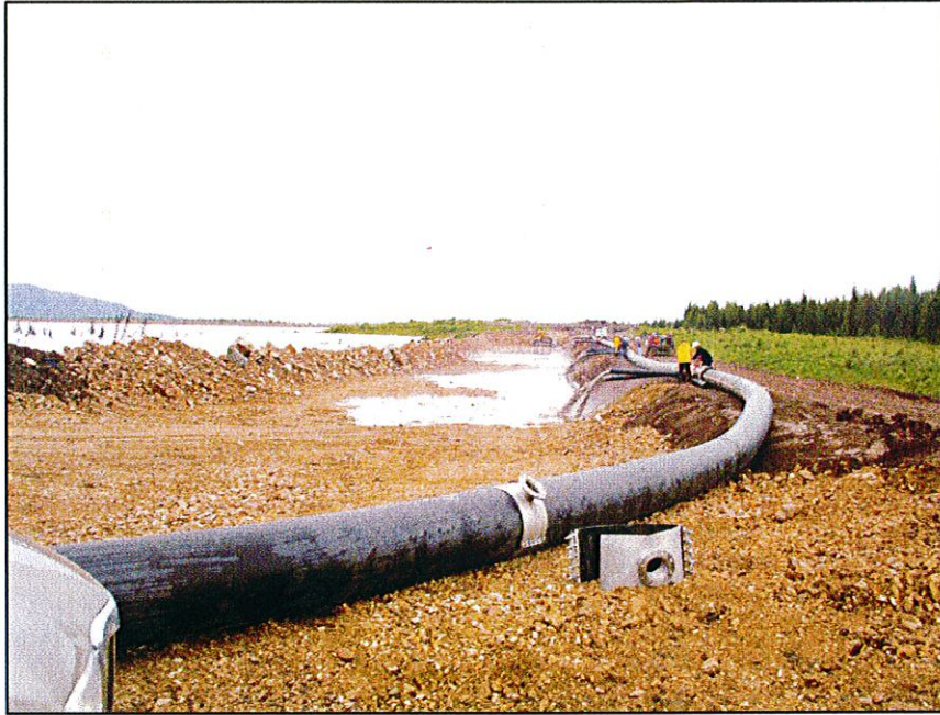
PHOTO 9 – Spigoting tailings into the sand cell at the South Embankment.
