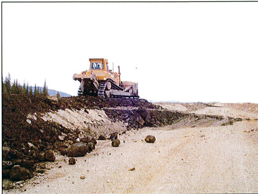
PHOTO 27 –Till ramps were set up to minimize the traffic on the Zone S material with the 777 haul trucks.
