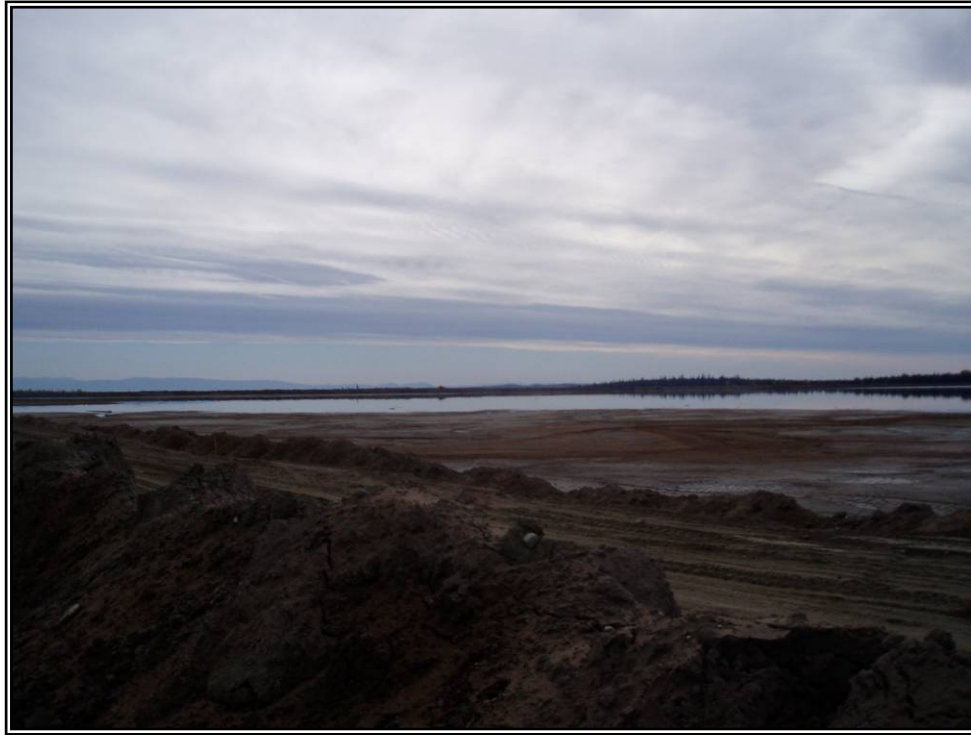
Photo 19: Tailings Pond from Northwest end of Perimeter Embankment
