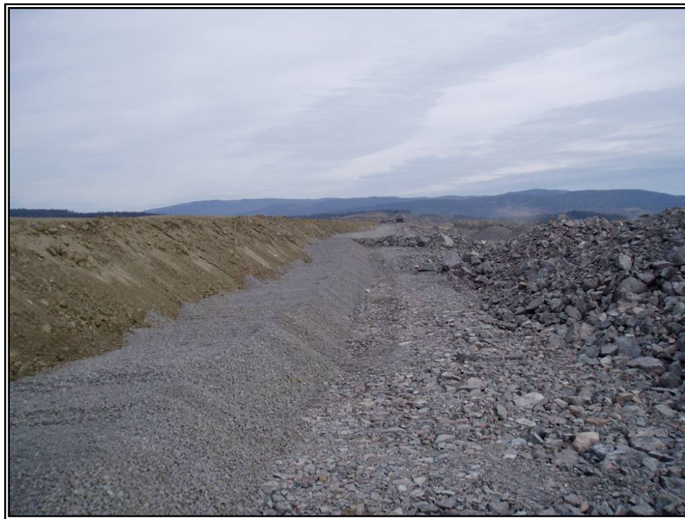
Photo 6: Zones of Main Embankment Dam
