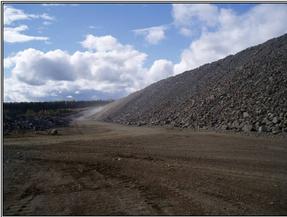
Photo 2: Main Embankment Shell – Looking Southwest
