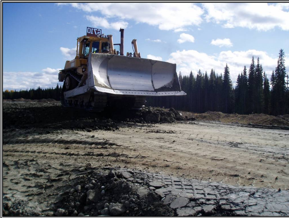
Photo 13: Compacted Till – South Embankment
