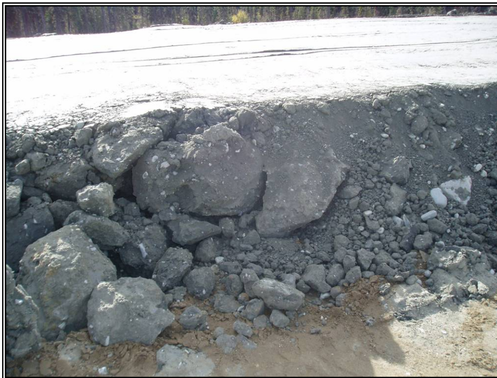
Photo 14: Compacted Till – South Embankment
