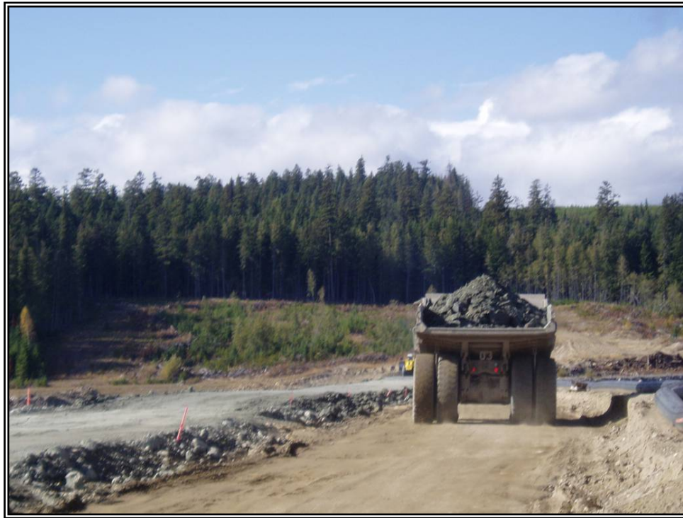
Photo 11: Till Haulage on South Embankment
