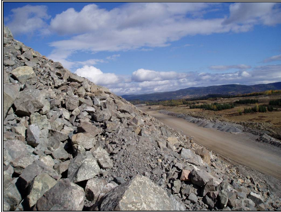
Photo 3: Nature of Main Embankment Rockfill
