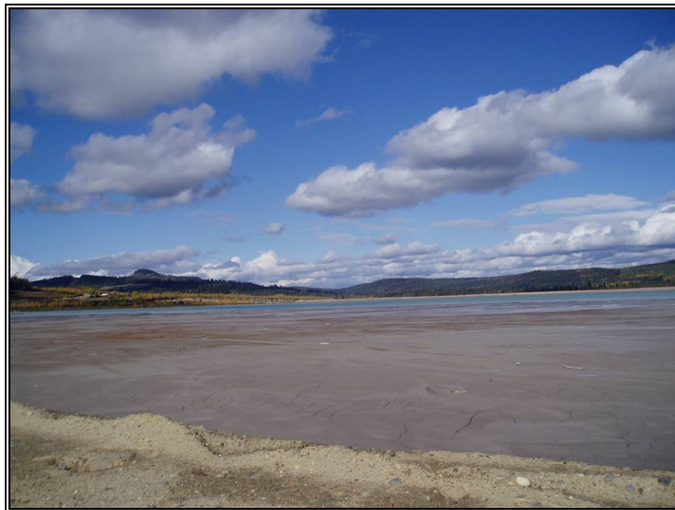
Photo 18: Minor Beach Development along Portion of Main Embankment
