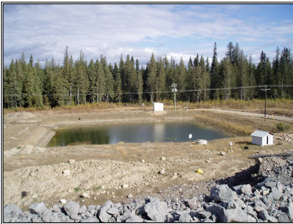
Photo 4: Main Embankment Seepage Collection
