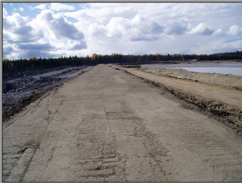
Photo 8: Main Embankment Compacted Core
