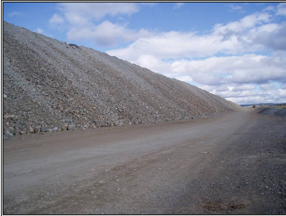
Photo 1: Main Embankment Shell – Looking Northeast
