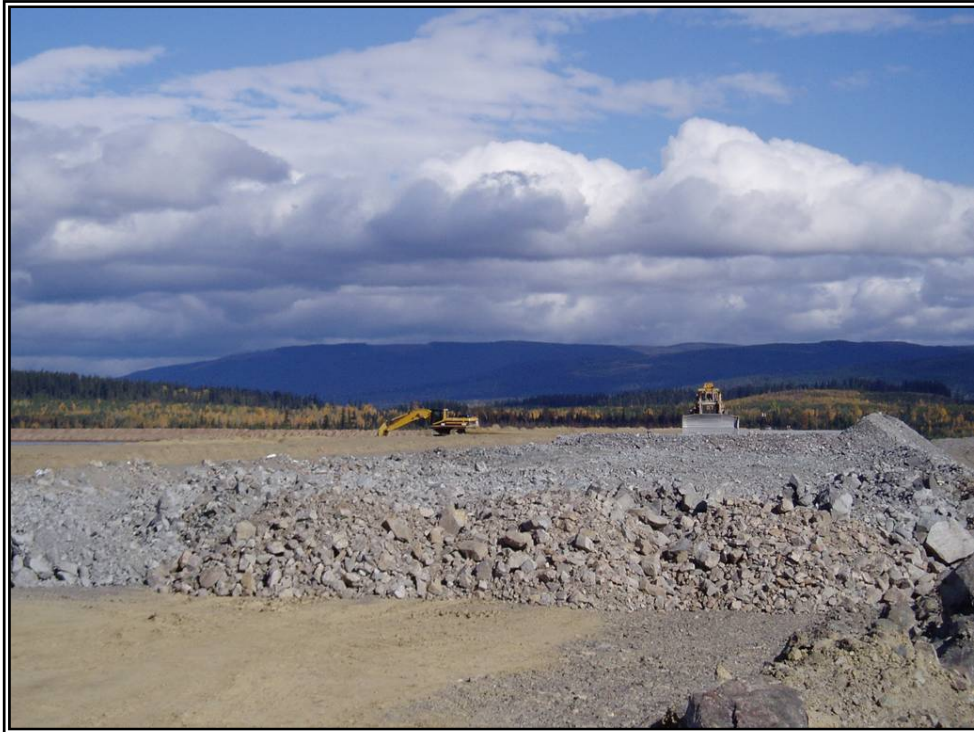
Photo 5: Construction on Main Embankment
