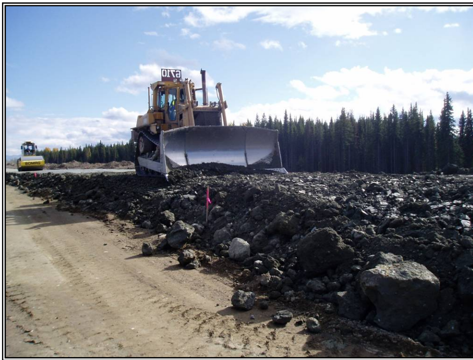
Photo 12: Placement of Till Core – South Embankment
