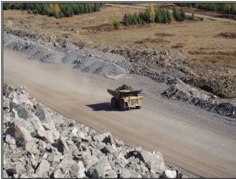
Photo 10: Haulage of Till from Borrow
