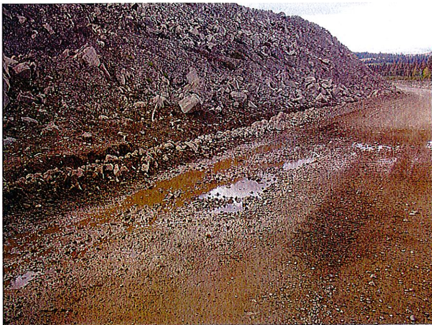
PHOTO 5: Minor seep at the Perimeter Embankment. Seepage routed to the Perimeter Embankment Seepage Collection Pond.
