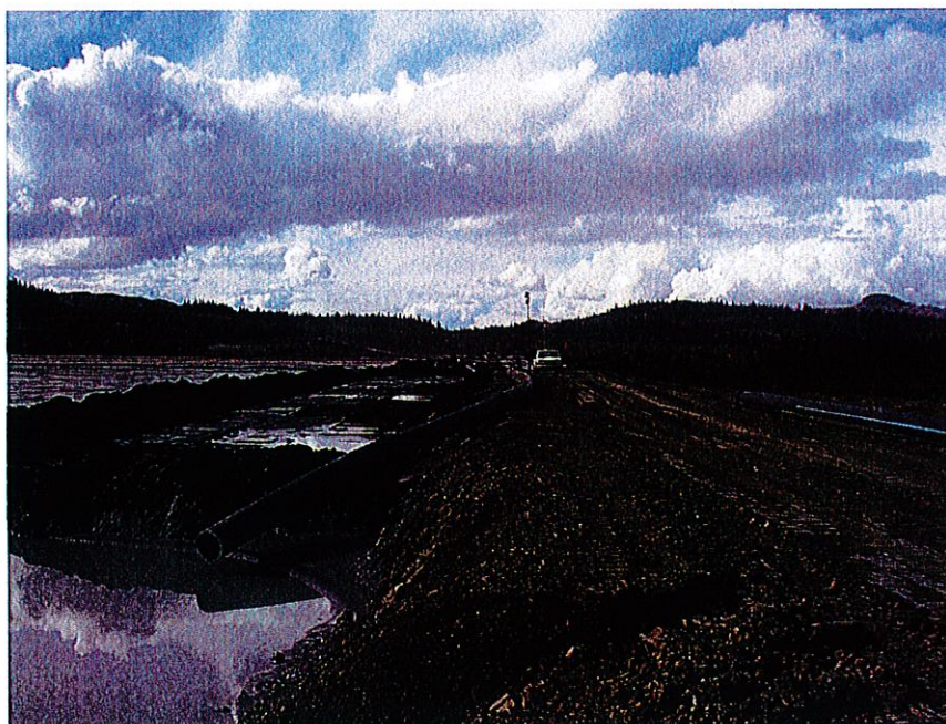
PHOTO 8: Perimeter Embankment. Construction of Zone U using the coarse tailings sand.
