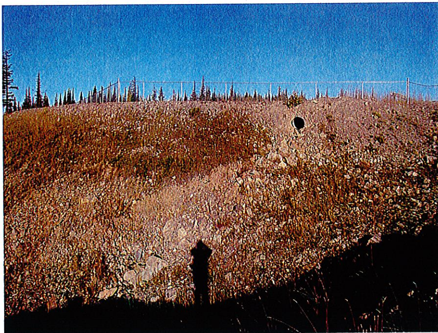
PHOTO 4: Millsite Sump Spillway showing signs of erosion
