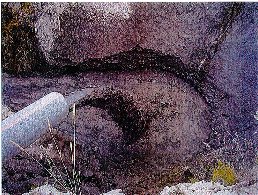
PHOTO 7: Single point discharge into the TSF at the knife gate valve located at the west end of the Perimeter Embankment.
