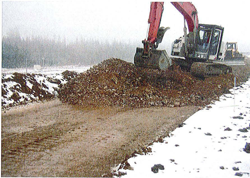
PHOTO 7 – Spreading rockfill/Zone T material with excavator.
