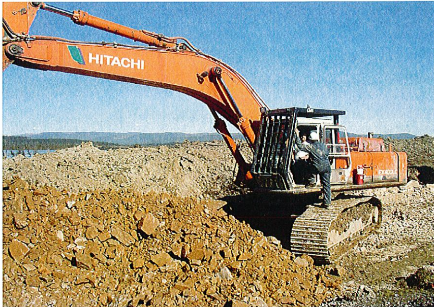
PHOTO 3 – Rockfill and Zone T placement with Hitachi Excavator.
