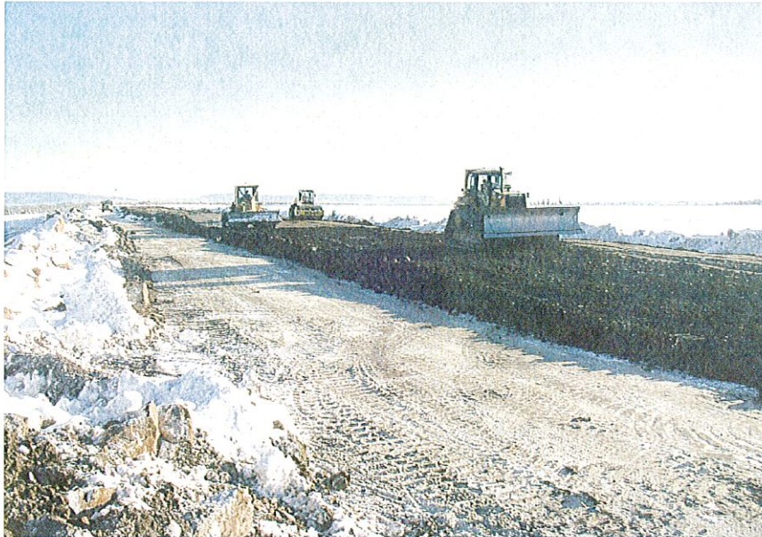
PHOTO 21 – Spreading and compaction of Zone S material during cold weather.
