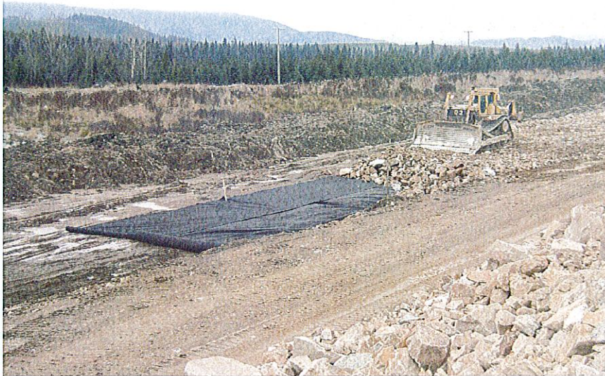
PHOTO 9 – Geotextile placement at the perimeter embankment.
