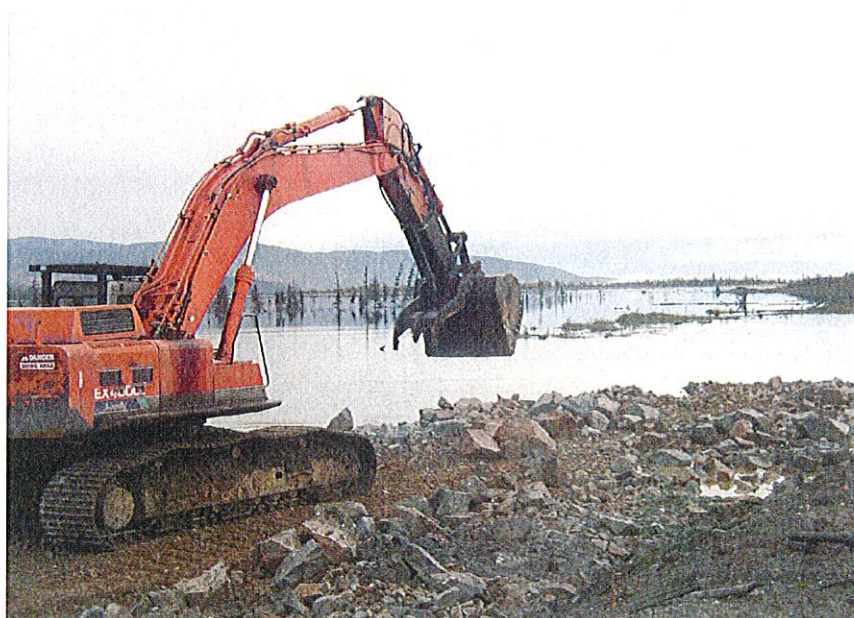
PHOTO 12 – Rockfill placement and spreading using excavator at the south embankment.
