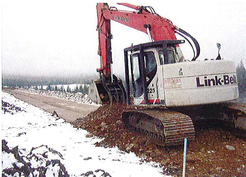
PHOTO 6 – Spreading Zone T material with excavator at Main Embankment.
