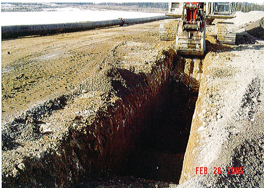
PHOTO 25 – Trenching for Zone F material at the perimeter embankment.
