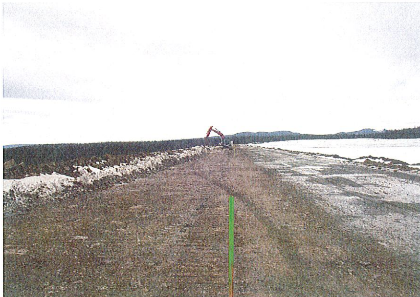
PHOTO 24 – Surveying for Zone F trench by surveying crew before excavating.
