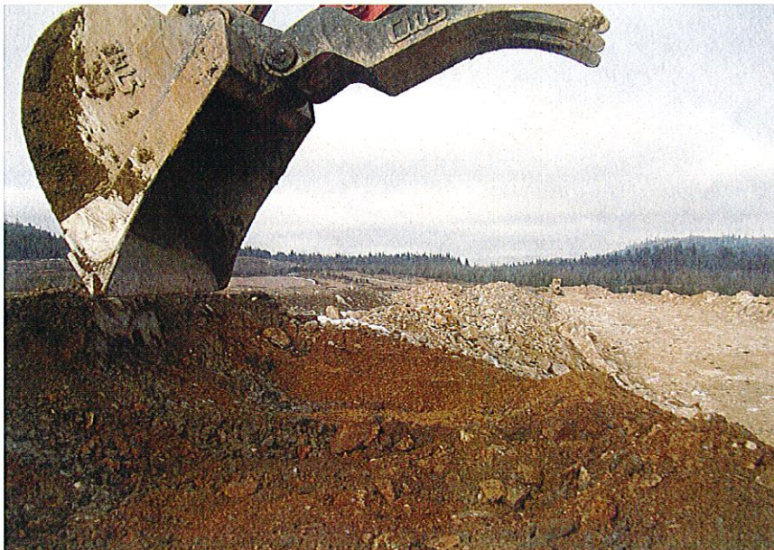
PHOTO 10 – Spreading Zone T material.
