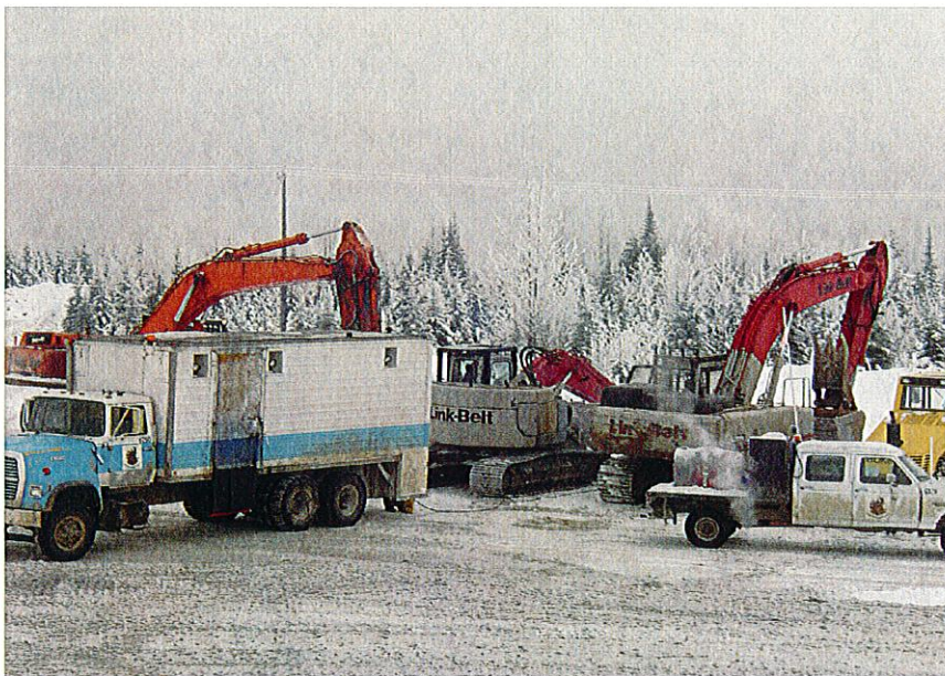
PHOTO 22 – Maintenance of construction machinery.
