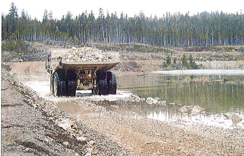
PHOTO 1 – Hauling rockfill to the south embankment by a 777 Cat Truck.
