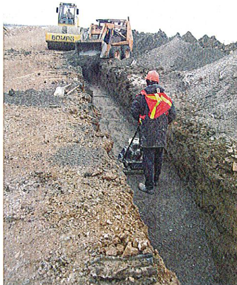
PHOTO 18 – Placement and compaction of Zone F material.
