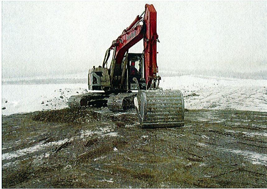
PHOTO 23 – Foundation preparation/snow removal using excavator before placing next Zone S lift.
