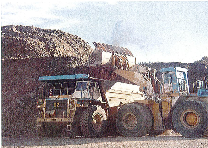
PHOTO 4 – Loading of 777 Cat Truck with loader at rock borrow area.
