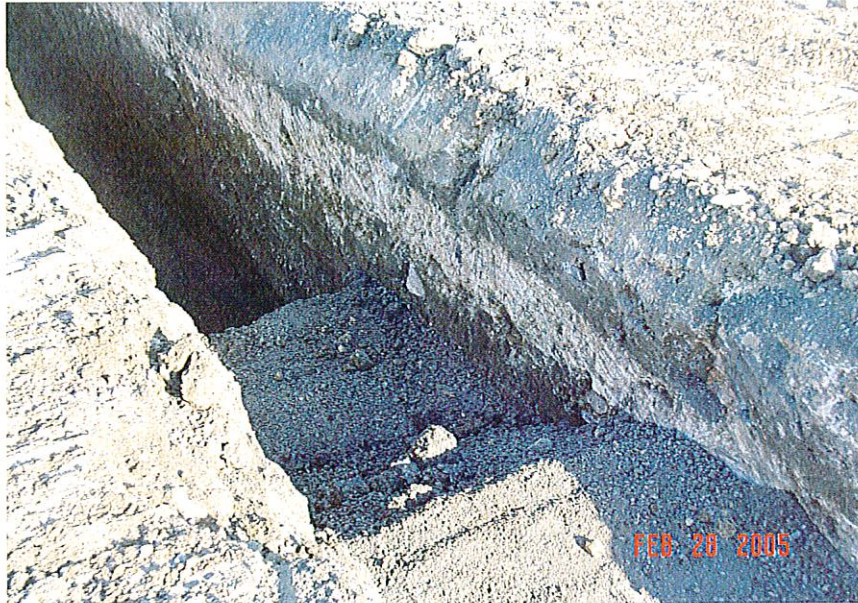
PHOTO 29 – Compacted Zone F materials using excavator.
