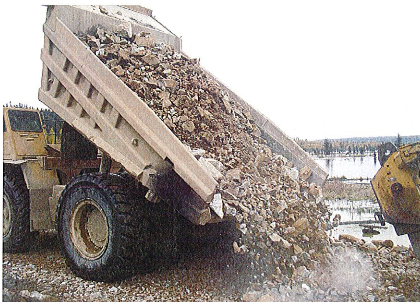
PHOTO 2 – Dumping rockfill at the south embankment.
