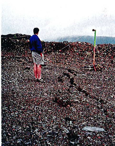
PHOTO 10: Tension cracks along east side of Waste Dump
