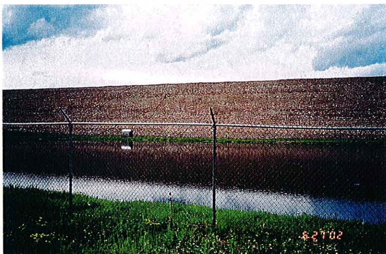
PHOTO 3: Main Embankment and Seepage Collection Pond
