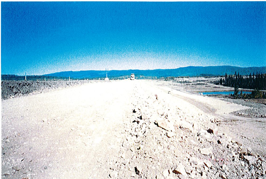
September 2000 - Main Embankment construction
