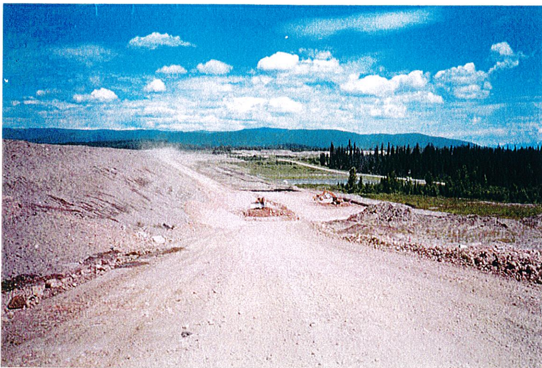
August 2000 - Downstream buttress construction - Main Embankment
