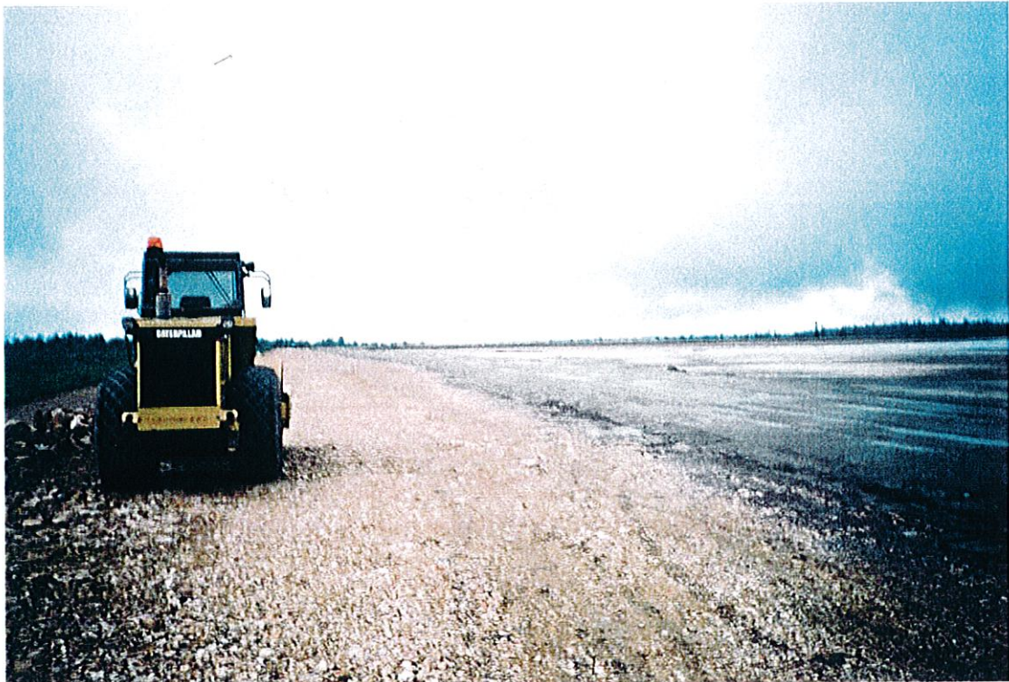
July 2001 - Perimeter Embankment at El. 942.5 m
