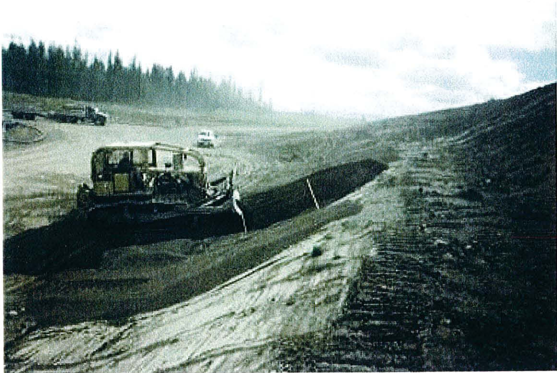
June 2001 - Perimeter Embankment Zone F construction
