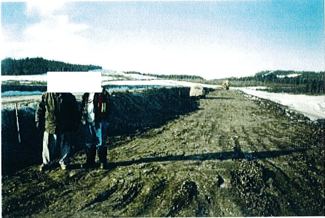
January 2001 - Perimeter Embankment Zone S construction
