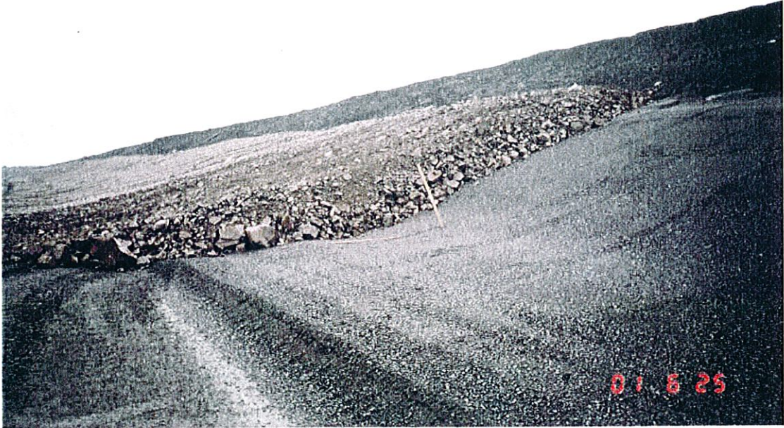
June 2001 - Perimeter Embankment Zone T construction
