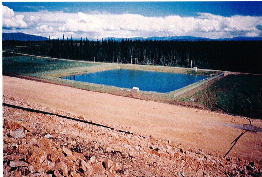
PHOTO 4: Main Embankment Seepage Collection Pond from Main Embankment Crest- Looking South
