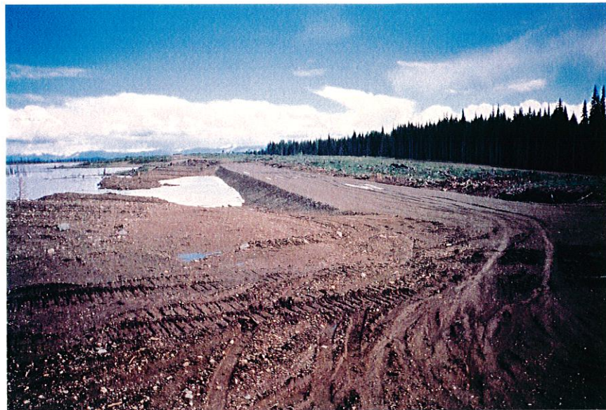
PHOTO 5: South Embankment from Right Abutment – Looking East
