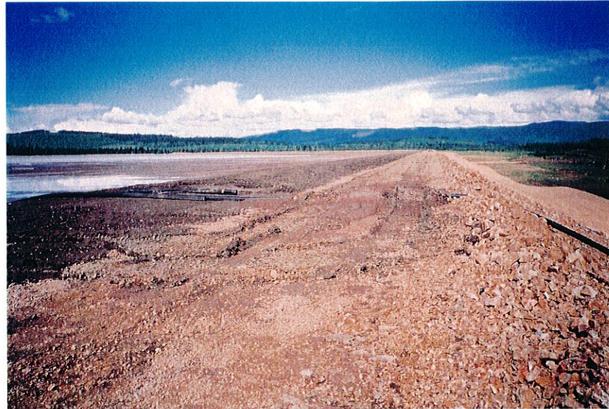
PHOTO 3: Main Embankment from Right Abutment – Looking East
