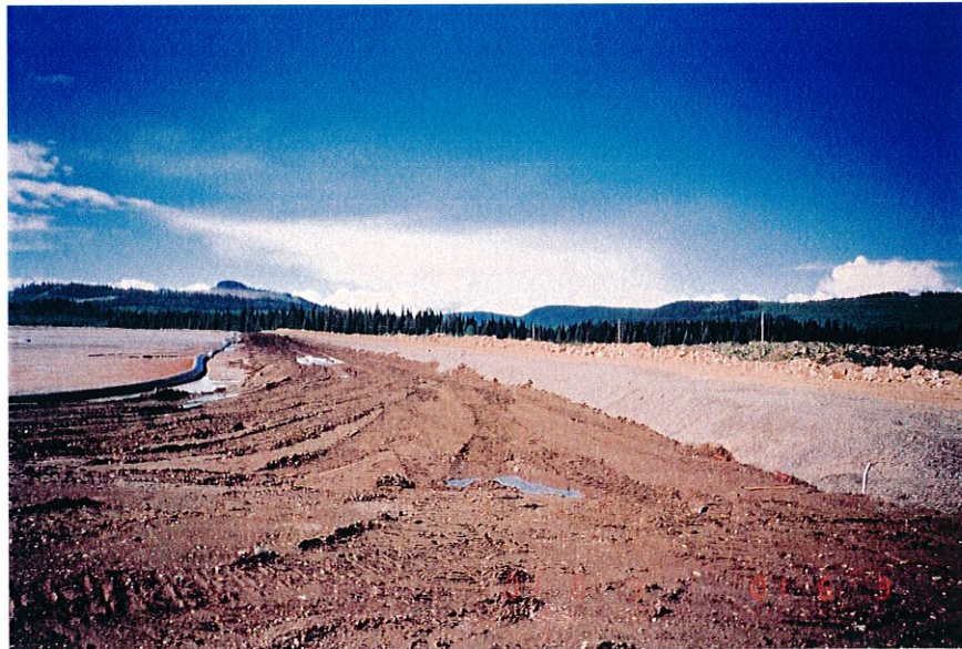
PHOTO 2 – Perimeter Embankment from Main Embankment – Looking North
