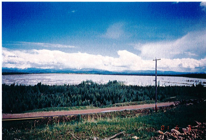
PHOTO 7: Reclaim Line and Tailings Impoundment – Looking East
