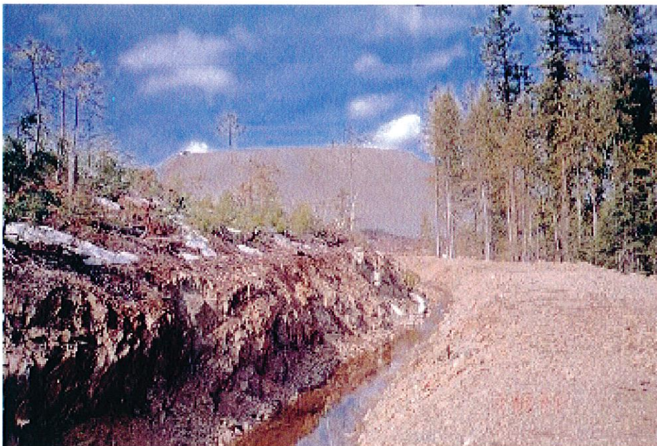
Photo No. 13: Runoff collection ditch leading to the Southeast Sediment Pond. Mine waste dump in background.
