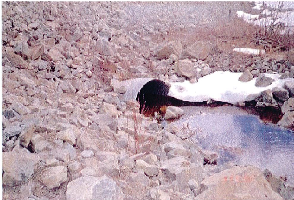
Photo No. 10: Bootjack Creek Culvert, upstream end.
