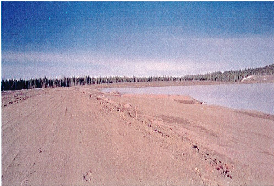
Photo No. 2: Main Embankment, view looking west from the left abutment.
