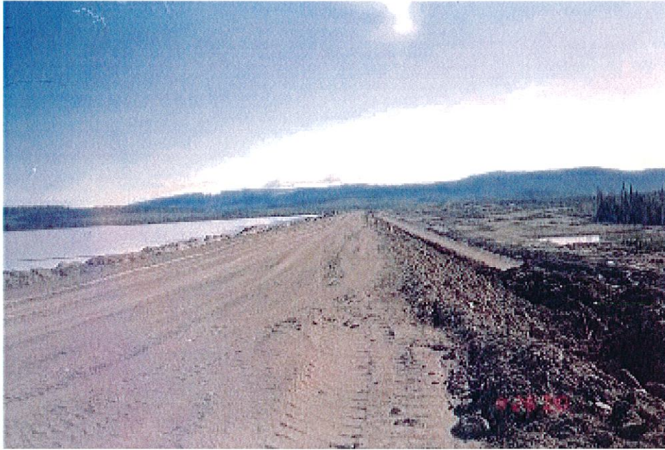
Photo No. 1: Main Embankment, view looking east from the right abutment.
