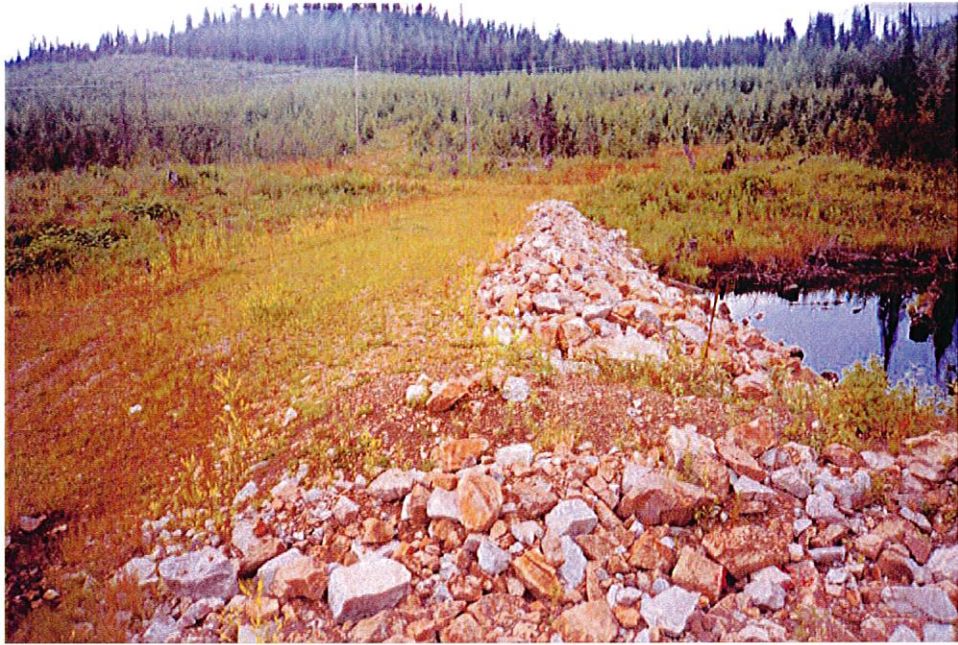
Photo No. 17: South Bootjack Dam, upstream slope.
