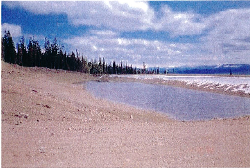
Photo No. 14: Southeast Sediment Pond, looking east.
