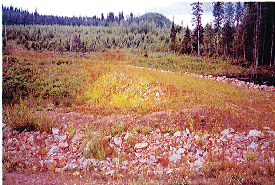
Photo No. 17: South Bootjack Dam, downstream slope with spillway in foreground.
