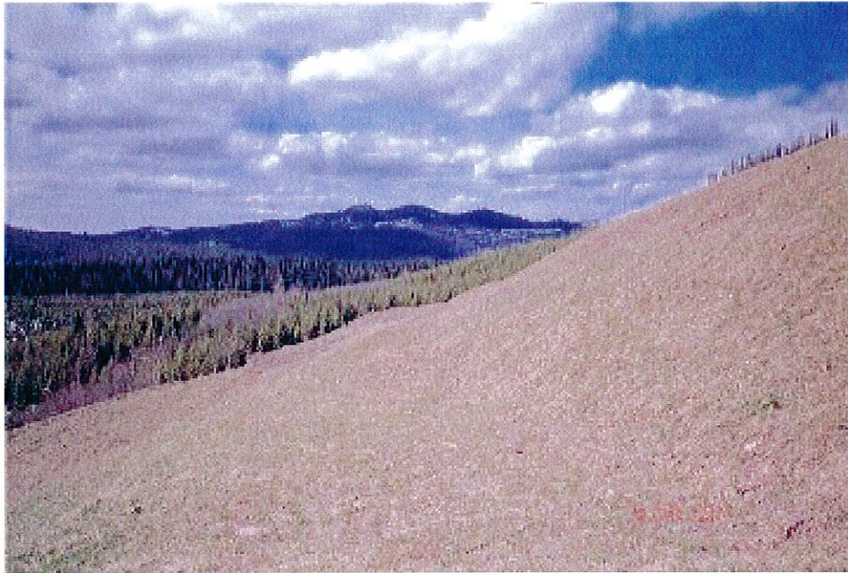
Photo No. 15: Southeast Sediment Pond. Downstream fill slope looking west. Slope is dry and stable and vegetation is well established.
