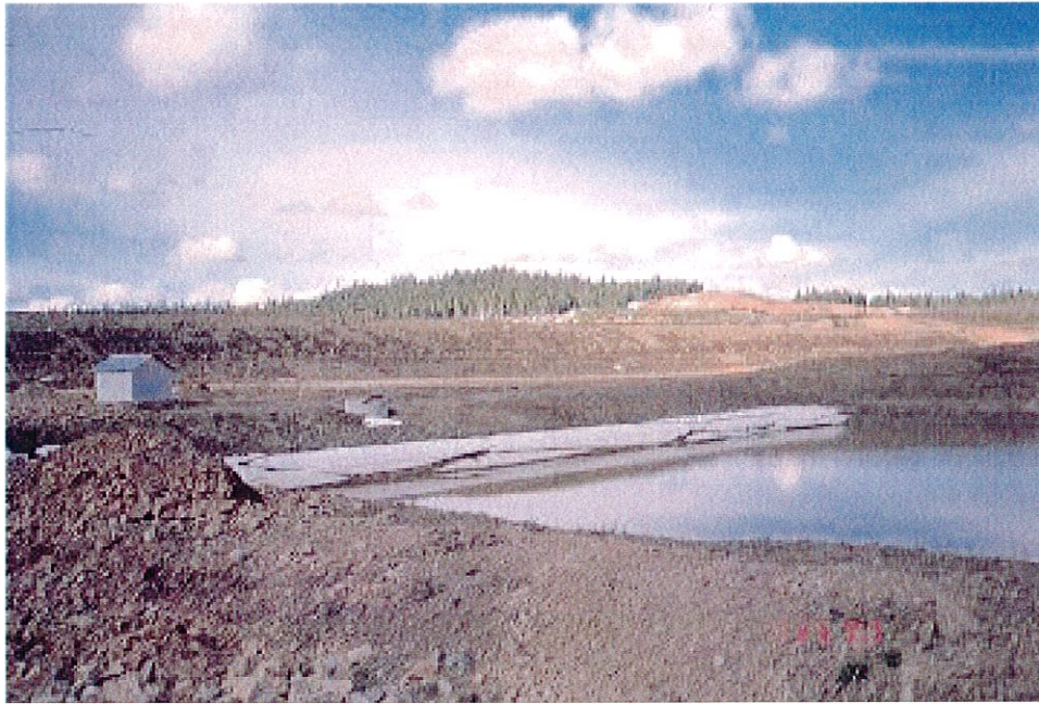
Photo No. 5: Perimeter Embankment and Seepage Collection Pond.
