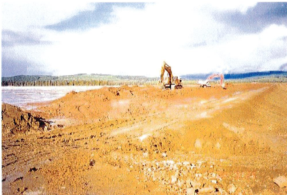
Photo No. 2: Upstream cycloned sand fill at the Main Embankment.
