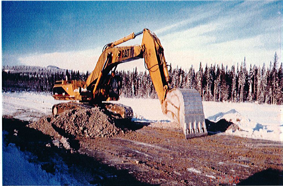
Photo No. 11: Removing snow and ice in preparation for fill placement.
