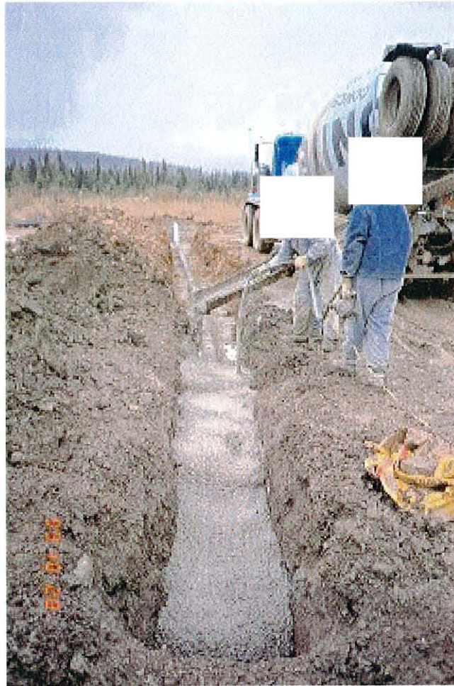
Photo No. 7: Upstream toe drain outlet pipe.
