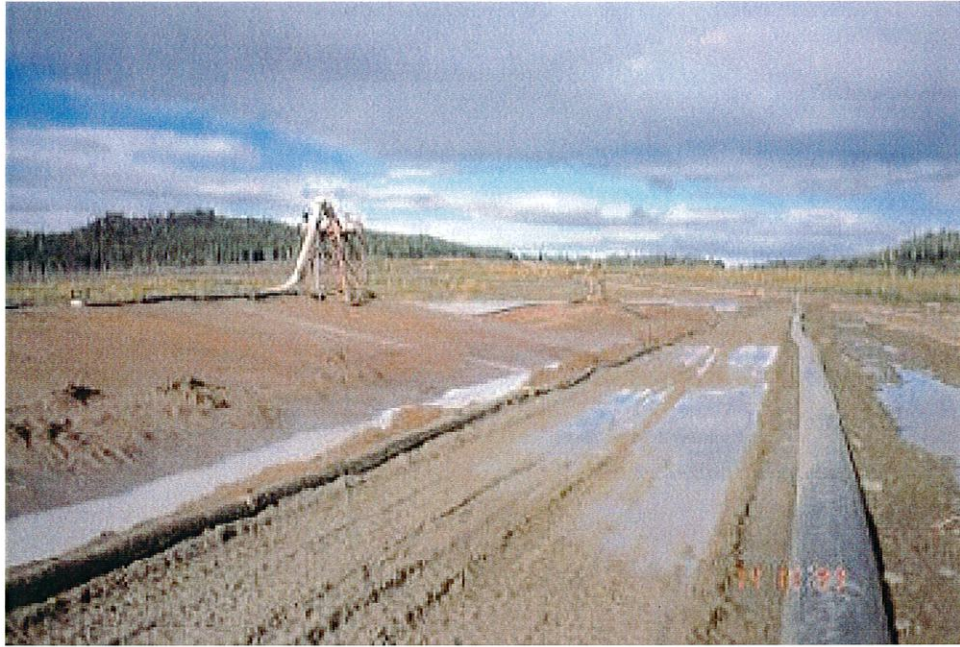
Photo No. 5: Upstream cycloned sand fill at the Perimeter Embankment.
