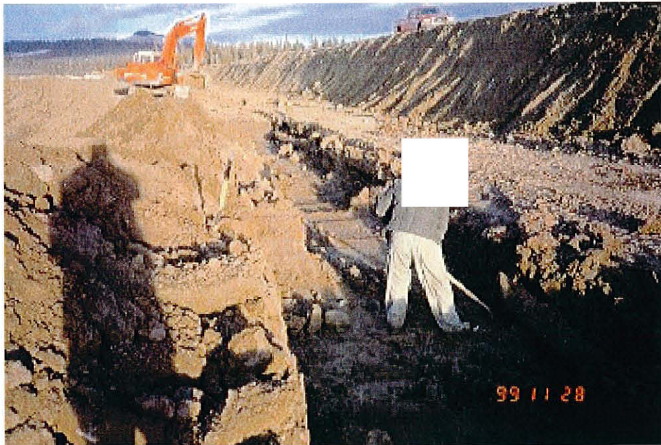
Photo No. 9: Trench for blank CPT pipe connecting Main and Perimeter Embankment upstream toe drains.
