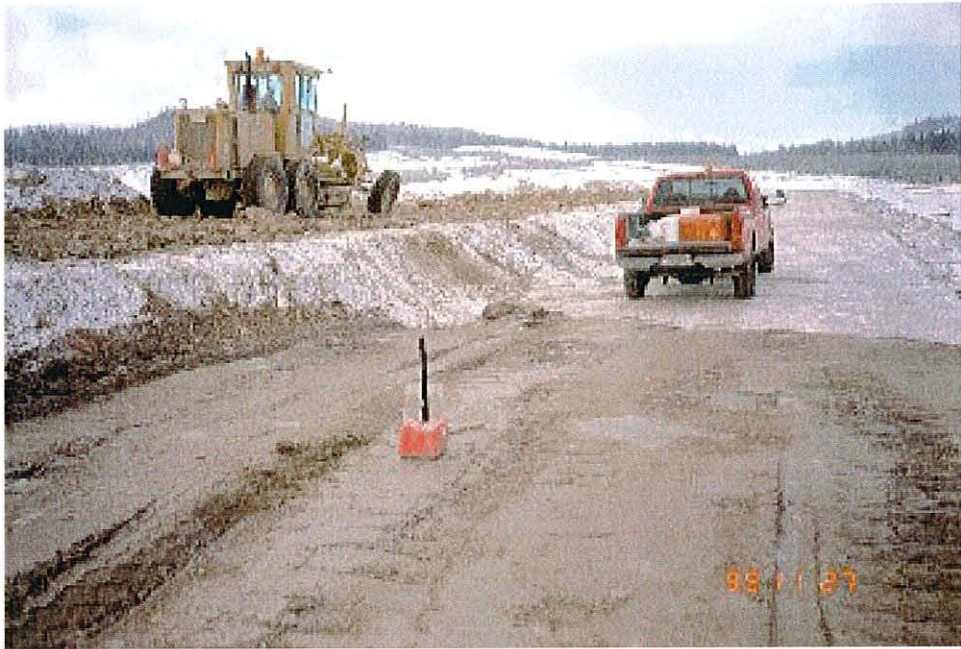
Photo No. 8: Density testing of Zone S fill.
