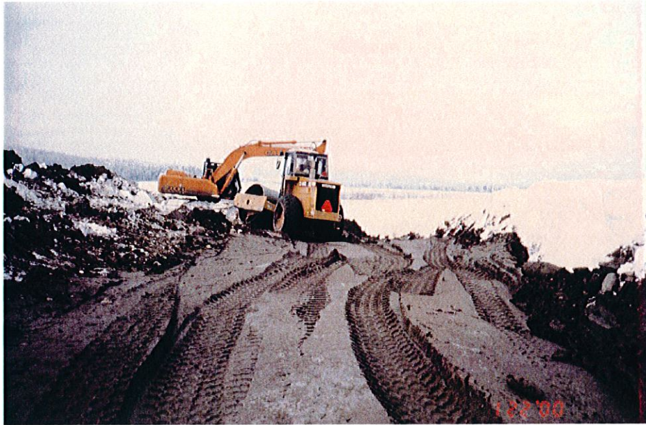
Photo No. 12: Backfilling basin liner trench.
