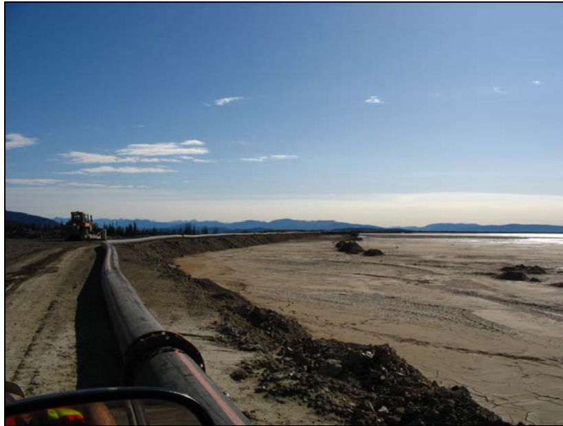
PHOTO 1 – Tailings beach development on the Perimeter Embankment
