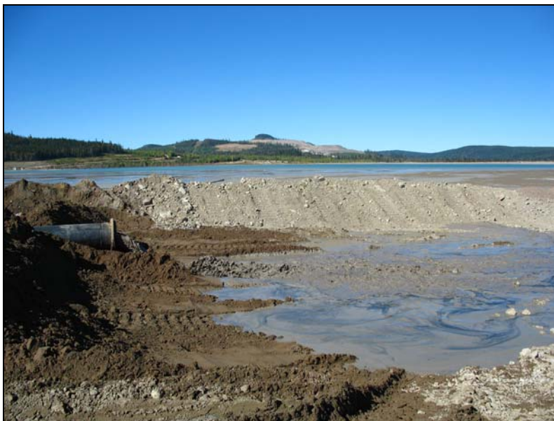
PHOTO 8 – Sand cell construction on Main Embankment.
