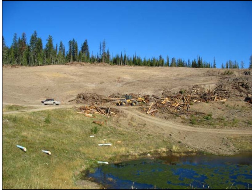
PHOTO 11 – Southeast Sediment Pond, west end showing outlet pipes
