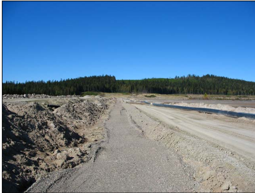
PHOTO 7 – South Embankment upstream toe drain.
