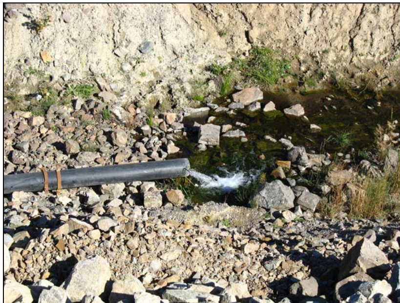
PHOTO 2 – Perimeter Embankment Toe Drain flow.
