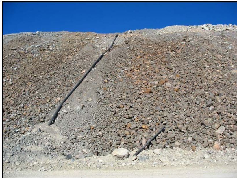
PHOTO 4 – Main Embankment Seepage Collection Pond Return Pipe
