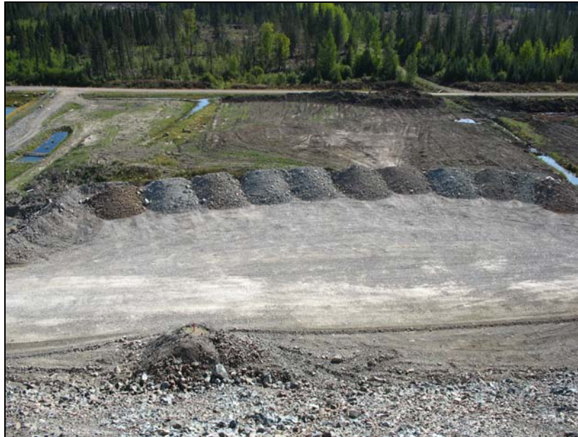
PHOTO 9 – Buttress construction at the Main Embankment.
