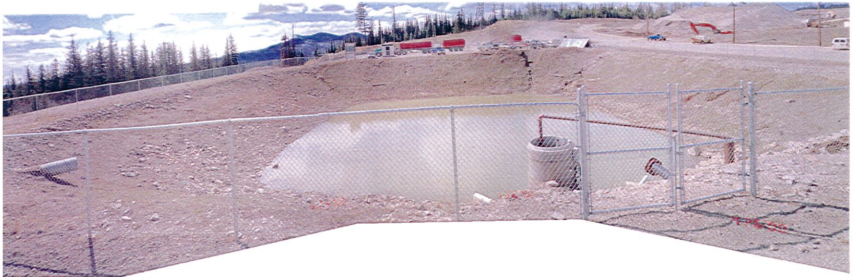
Photo No. 18: Millsite Sump.
