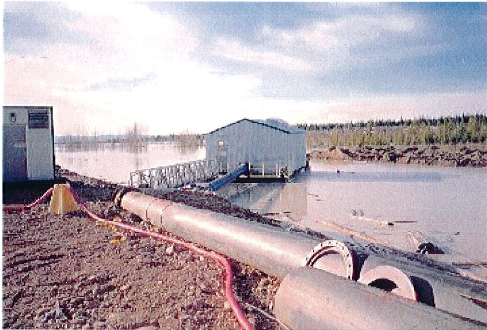
Photo No. 12: Reclaim Barge and Channel.
