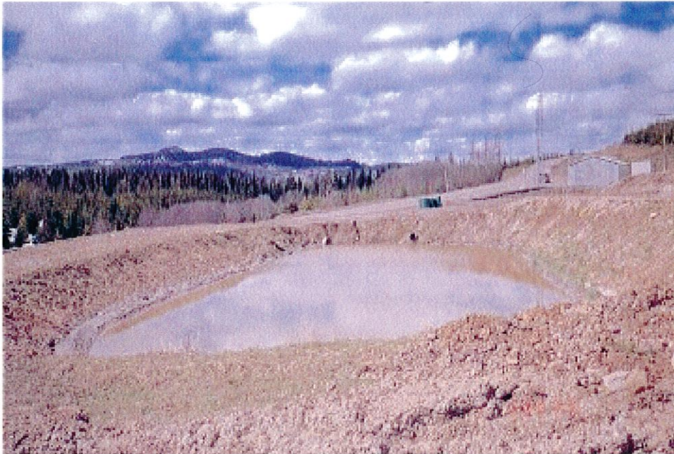
Photo No. 11: T2 Overflow Pond, full of water.
