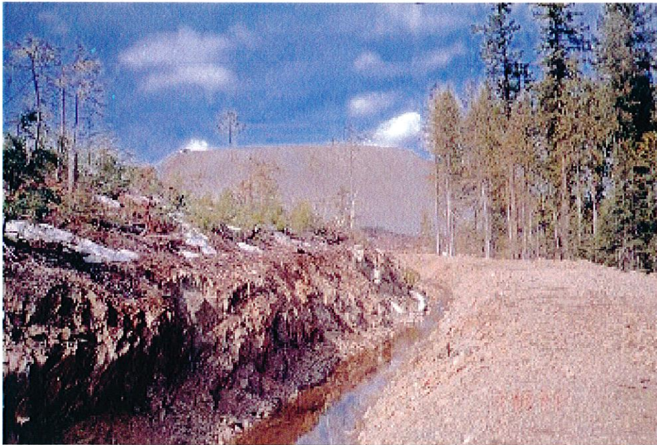
Photo No. 13: Runoff collection ditch leading to the Southeast Sediment Pond. Mine waste dump in background.
