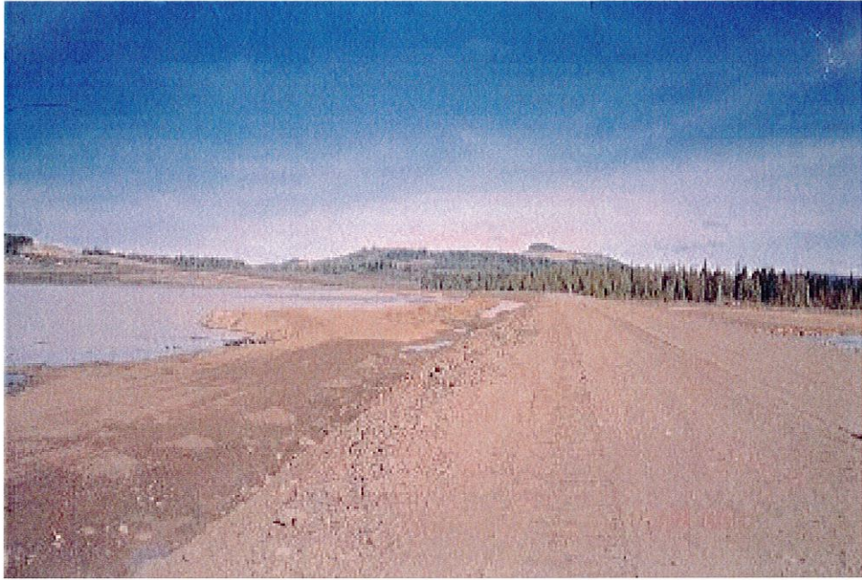
Photo No. 3: Perimeter Embankment, looking north from right abutment.
