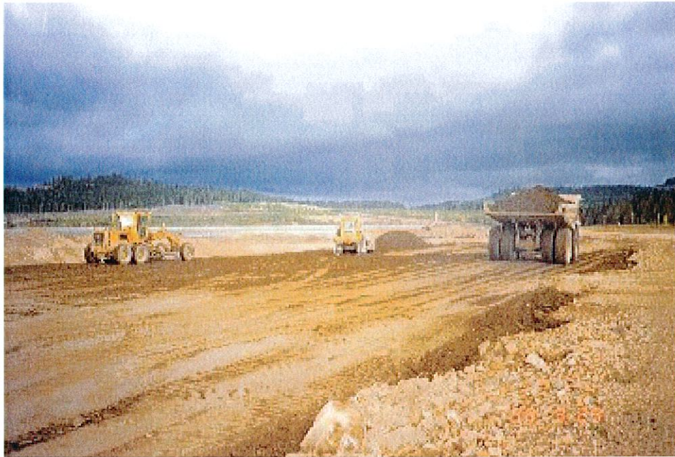
Photo No. 1: Fill placement at the Perimeter Embankment.
