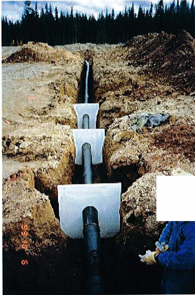
Photo No. 3: Upstream toe drain outlet with prefabricated seepage collars.
