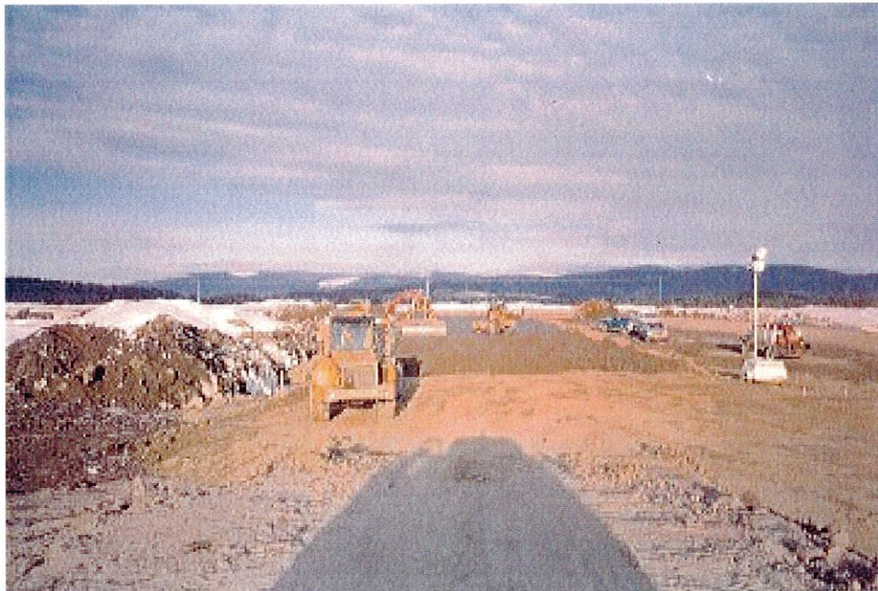
Photo No. 13: Fill placement at the Main Embankment.
