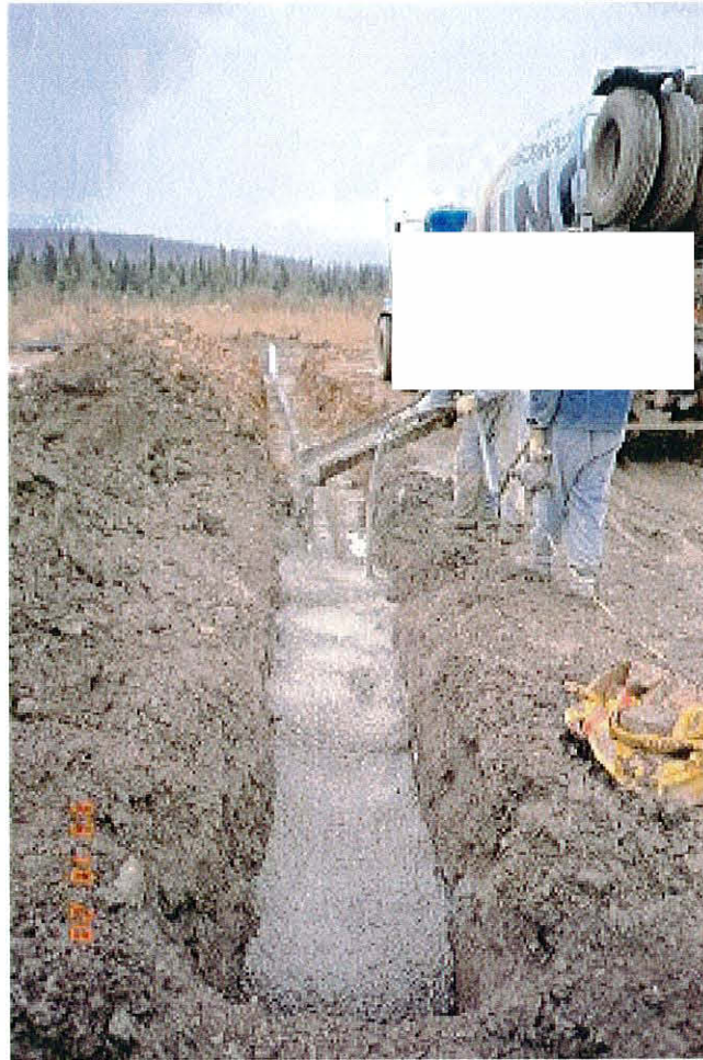
Photo No. 7: Upstream toe drain outlet pipe.
