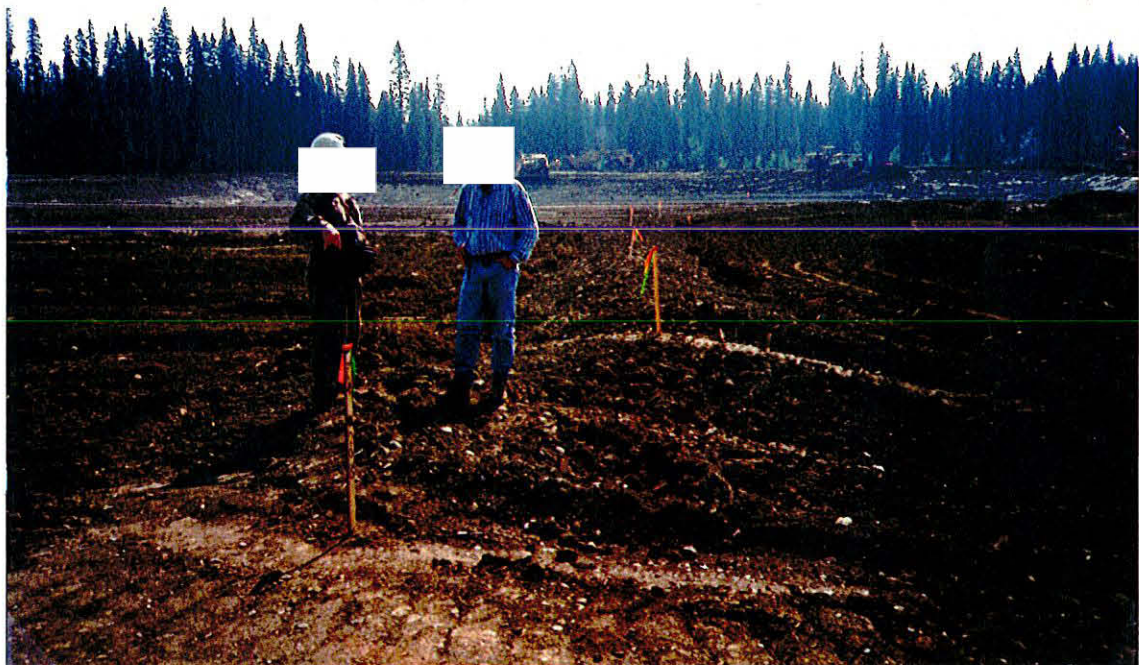
Photo 7. Base of Zone B of Stage 1b of Main Embankment. A Foundation Drain visible. Looking South-East.
