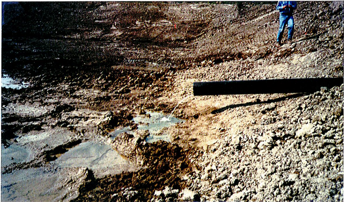
Photo 11. Outlet from Drain Monitoring Sump Discharging into Main Embankment Seepage Collection Pond.
