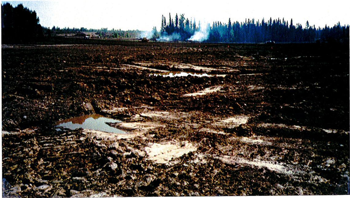
Photo 15. Surface of Basin Liner. Looking East.
