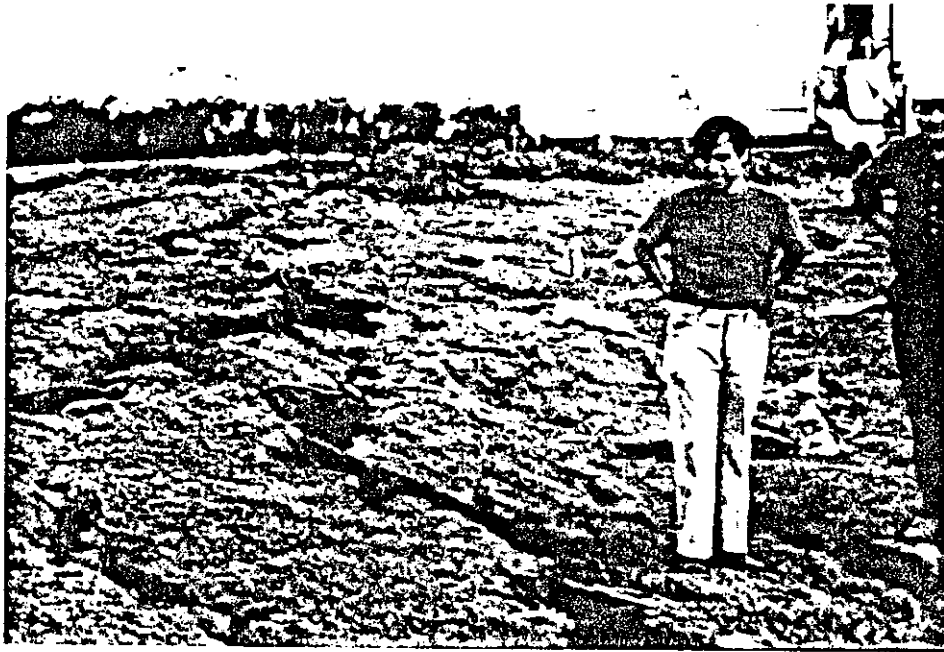
Damage behind the pitwall due to excessive blast charges per delay.
