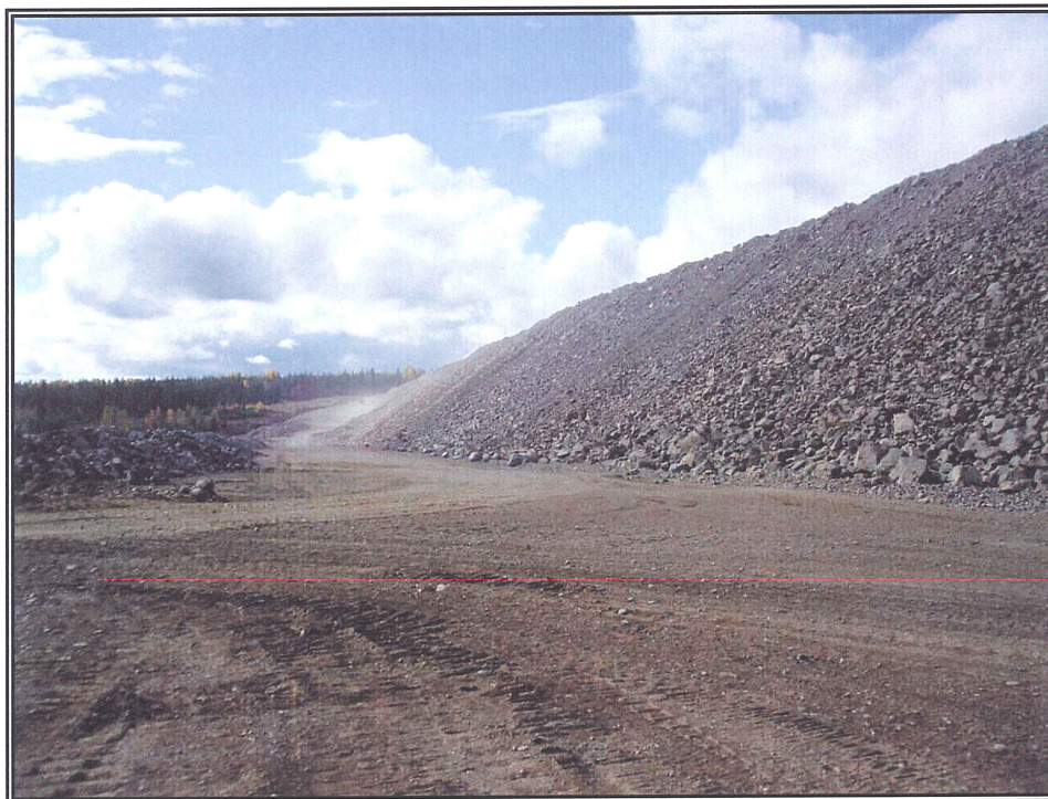
Photo 2: Main Embankment Shell – Looking Southwest
