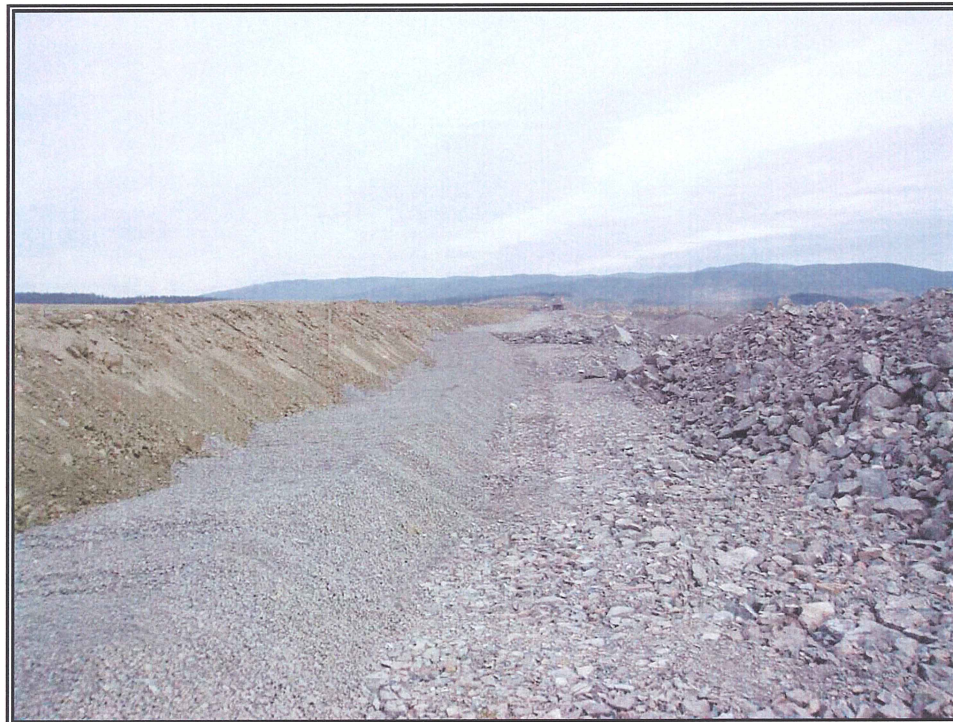
Photo 6: Zones of Main Embankment Dam
