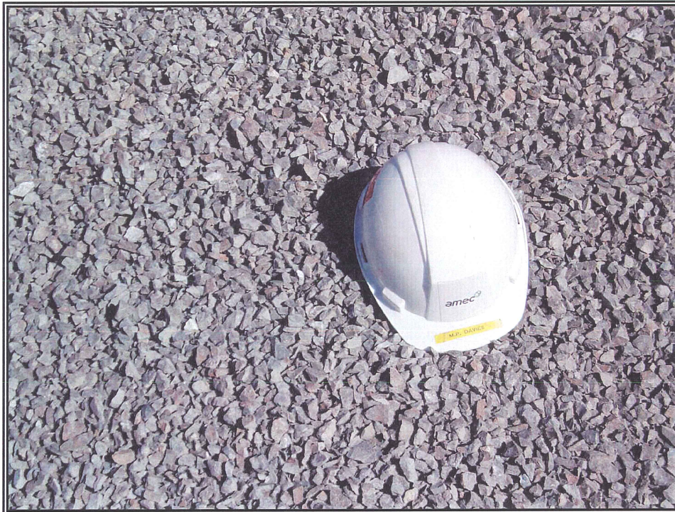
Photo 7: Main Embankment Transition Material
