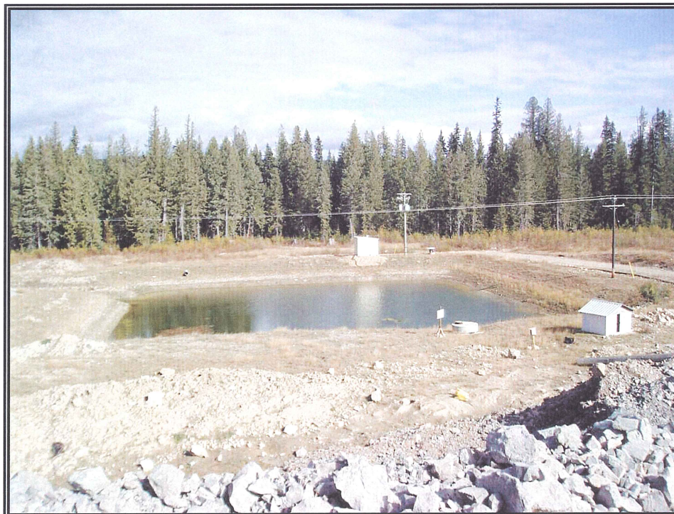
Photo 4: Main Embankment Seepage Collection
