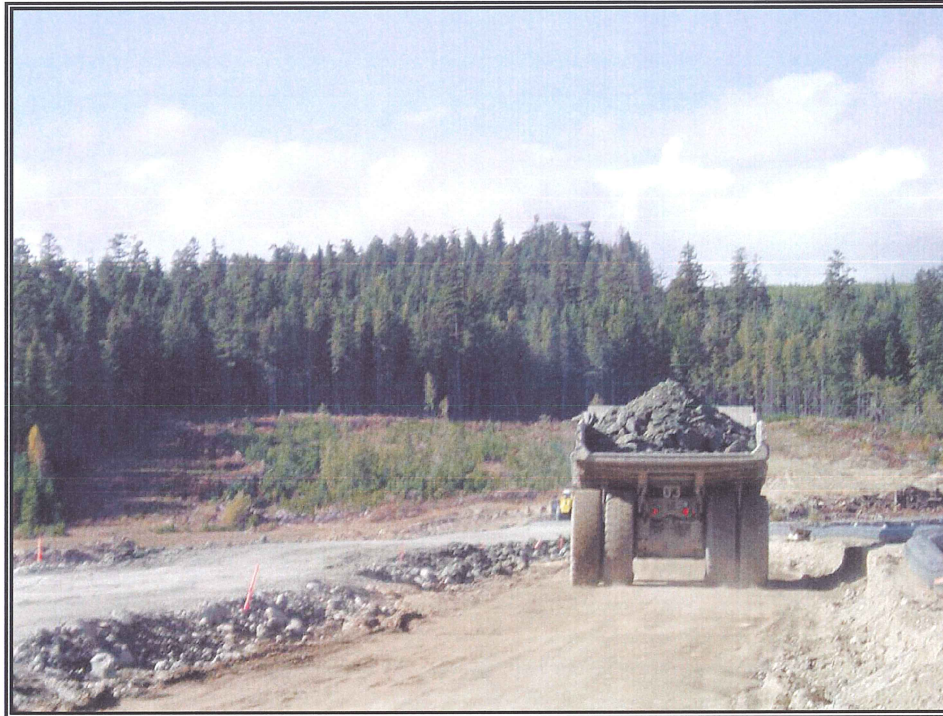
Photo 11: Till Haulage on South Embankment
