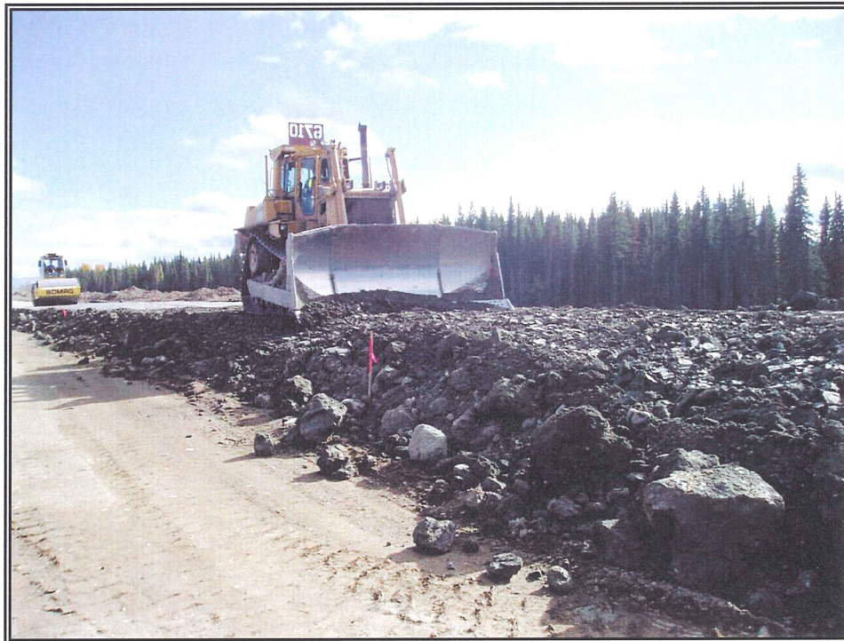
Photo 12: Placement of Till Core – South Embankment
