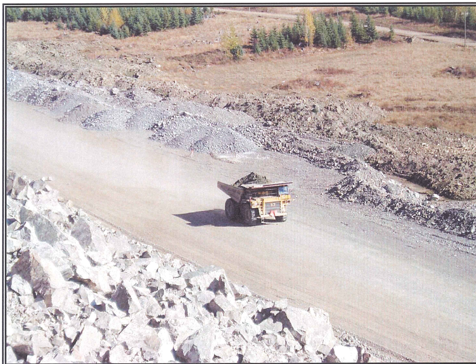
Photo 10: Haulage of Till from Borrow
