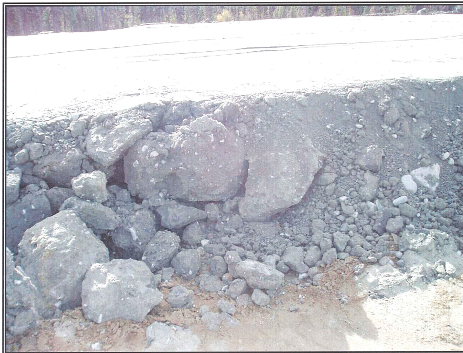
Photo 14: Compacted Till – South Embankment
