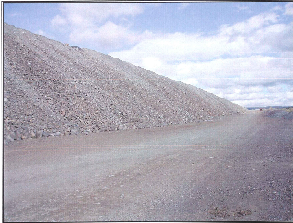
Photo 1: Main Embankment Shell – Looking Northeast
