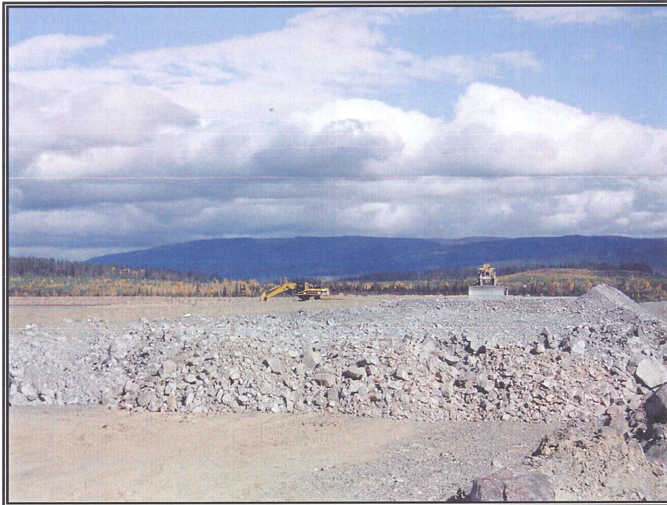
Photo 5: Construction on Main Embankment
