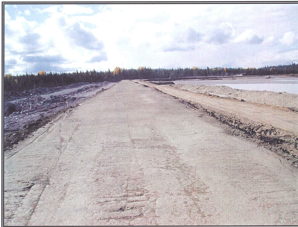
Photo 8: Main Embankment Compacted Core
