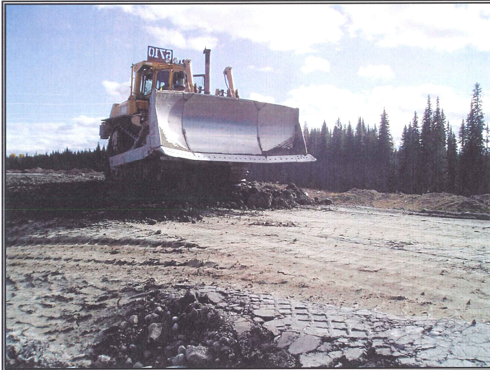
Photo 13: Compacted Till – South Embankment
