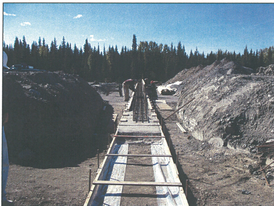
PHOTO 22 – South Embankment Concrete Encasement preparation.
