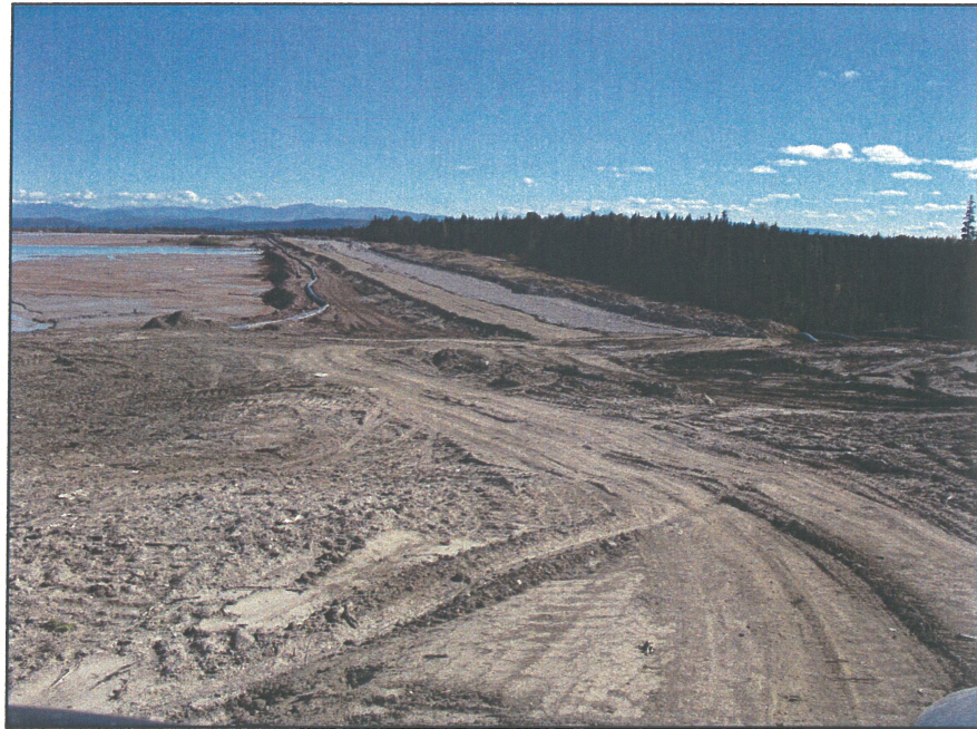
PHOTO 15 – South Embankment showing recent sand cell construction.
