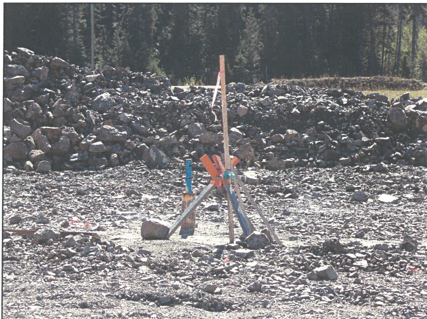
PHOTO 16 – Existing inclinometer at the Main Embankment.
