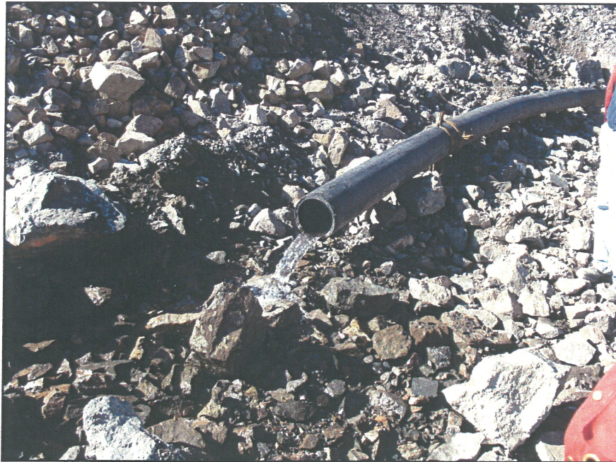
PHOTO 17 – Perimeter Embankment upstream toe drain flow
