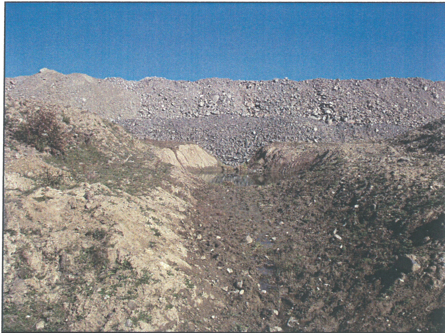
PHOTO 21 – South Embankment foundation drain excavated sump.
