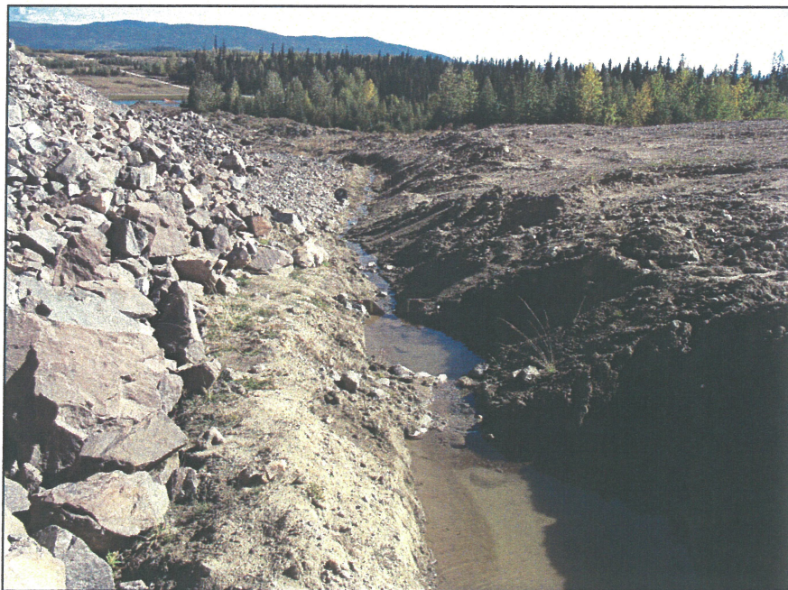
PHOTO 19 – Seepage from the Main/South Embankment corner routed to the Main Embankment Seepage Collection Pond.
