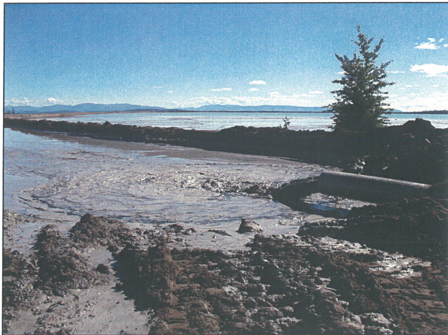
PHOTO 7 – Single point discharge on the Perimeter Embankment during sand cell construction.
