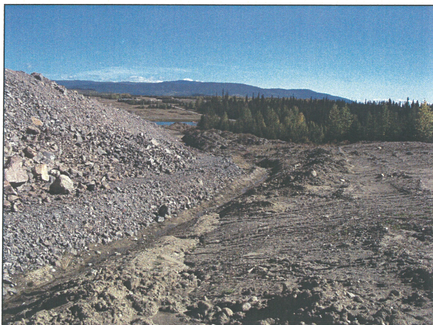
PHOTO 20 – Main Embankment ultimate downstream toe with a ditch routed to the Main Embankment Seepage Pond.
