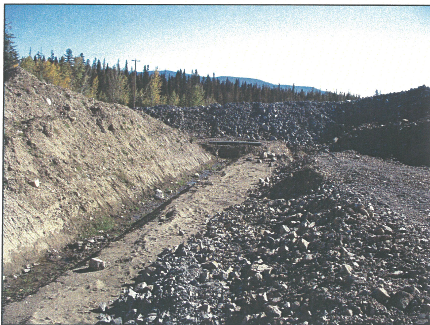
PHOTO 18 – Perimeter Embankment ditch routed to Perimeter Embankment Seepage Collection Pond for the upstream toe drain flow.
