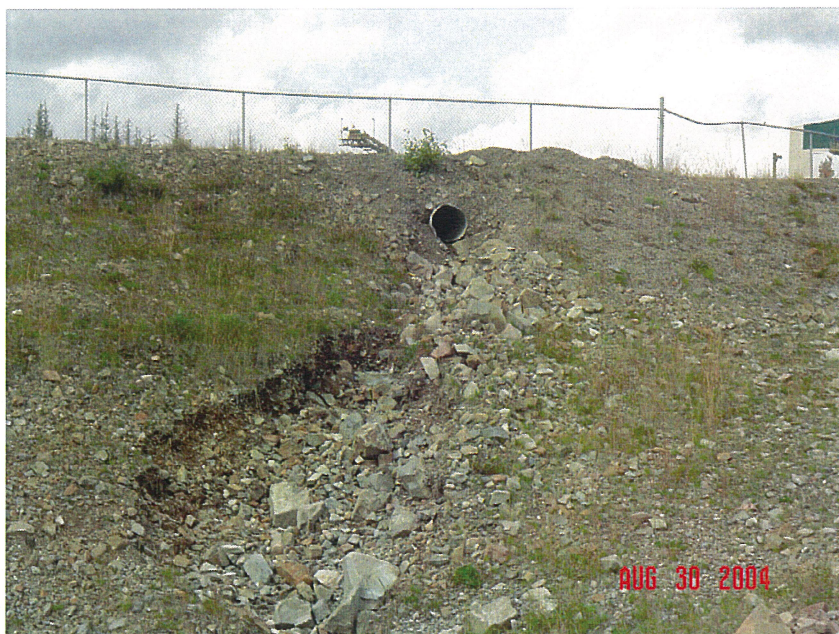
PHOTO 8 – Millsite Sump Spillway showing signs of erosion.
