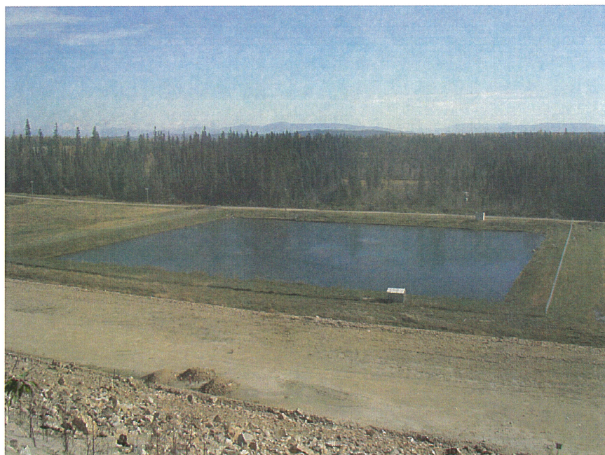
PHOTO 1 – Main Embankment Seepage Collection Pond.
