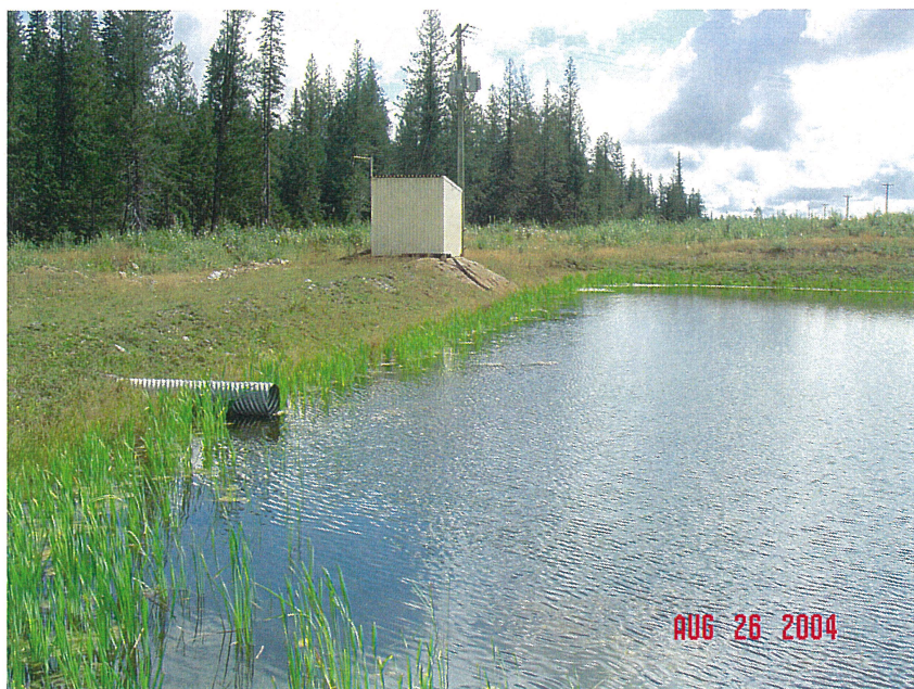
PHOTO 4 – Perimeter Embankment and Seepage Collection Pond.
