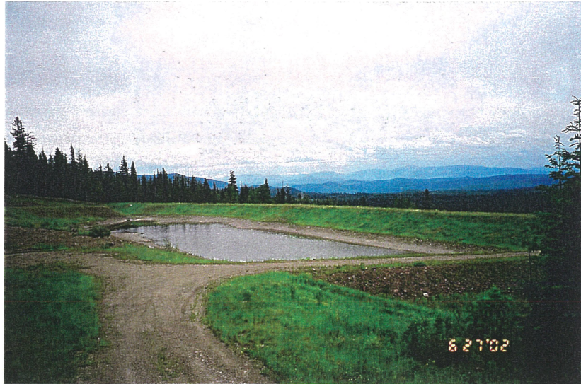
PHOTO 1: Southeast Sediment Control Pond
