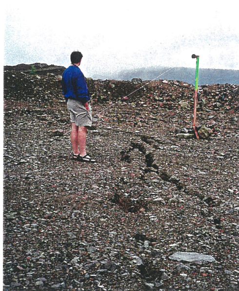
PHOTO 10: Tension cracks along east side of Waste Dump
