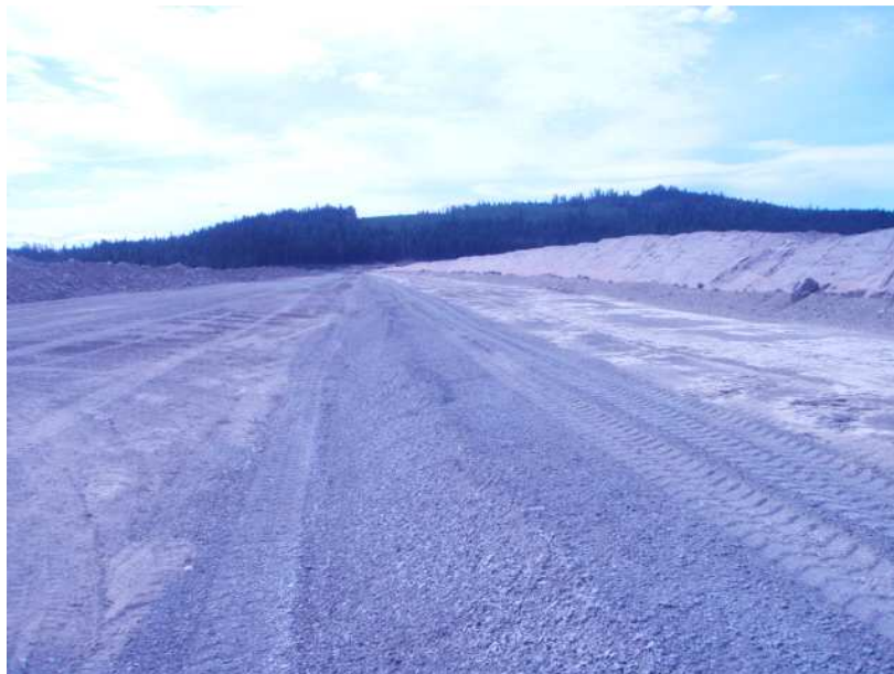
Figure 2: Completion of the SE filter layer.
