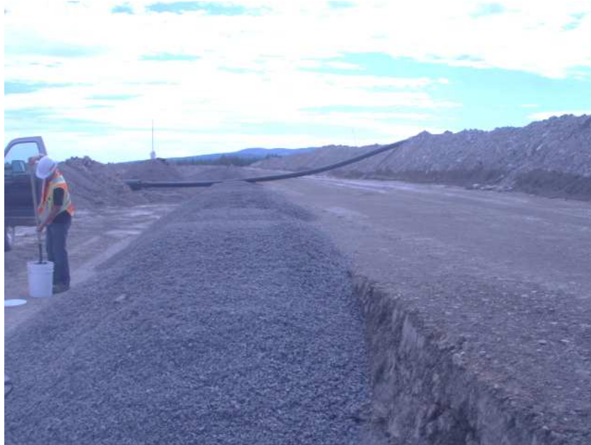
Figure 1: Filter placed near to the ME pipe.
