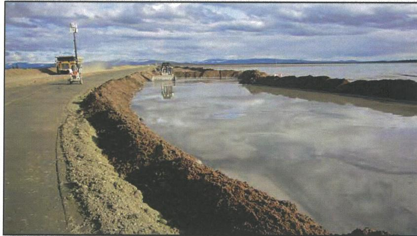
**PHOTO 2 – Sand cell construction on the Perimeter Embankment**
