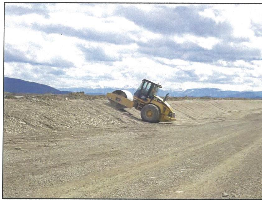
**PHOTO 13 – Compaction of Zone T transition material on the South Embankment**
