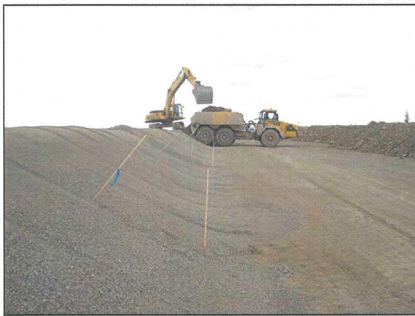
**PHOTO 12 – Placement of Zone T transition material on the South Embankment**
