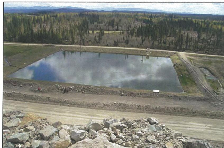
**PHOTO 21 – Main Embankment seepage pond**
