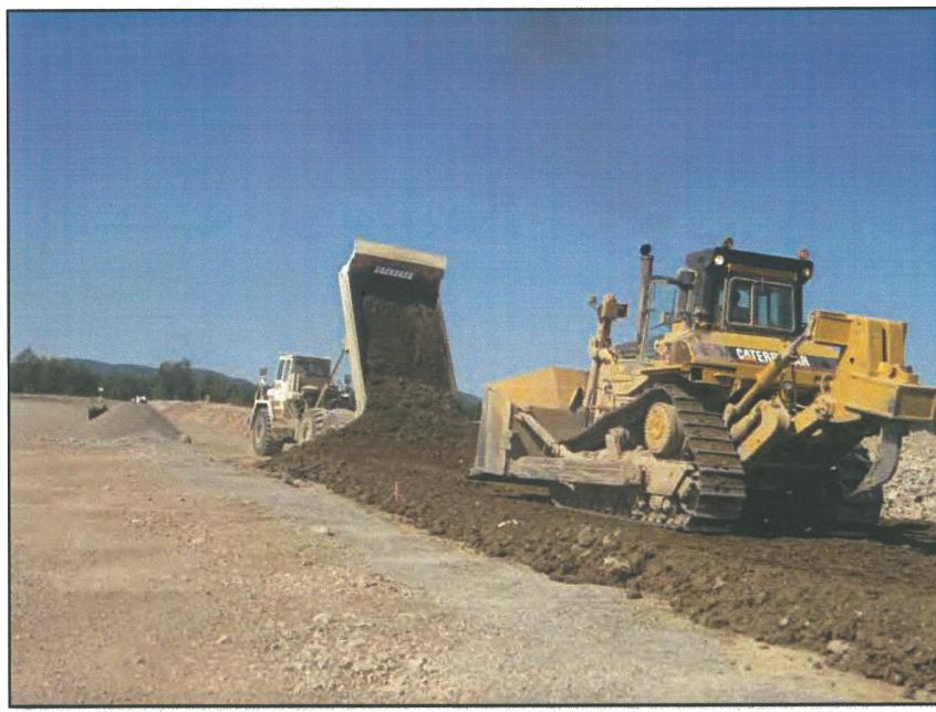
**PHOTO 4 – Placement of till material on the Main Embankment**
