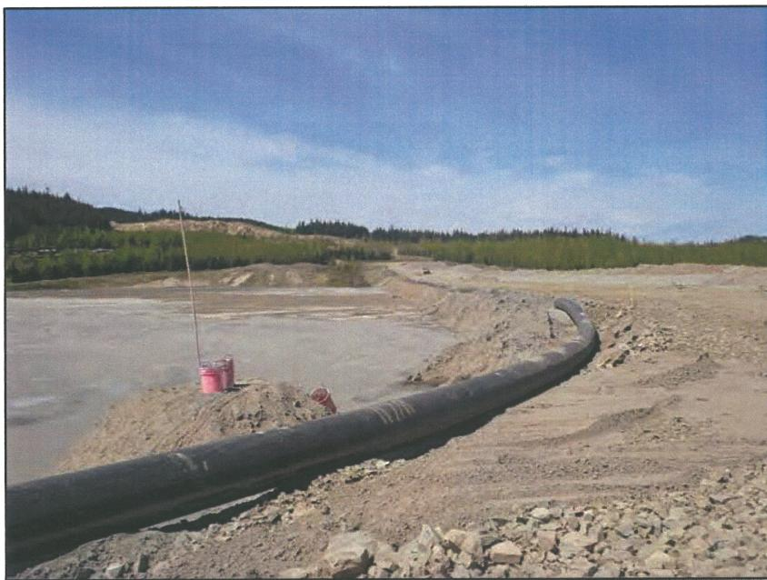
**PHOTO 19 – Tailings beach piezometers on the Perimeter Embankment**
