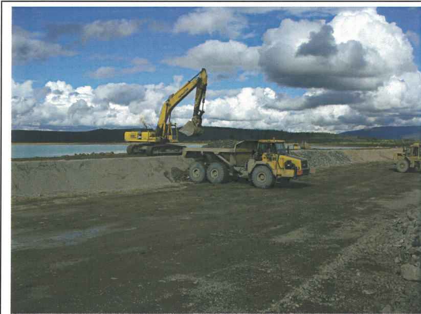
PHOTO 2 – Downstream components of TSF, Zone C (foreground), Truck is placing Zone T on top of Zone F, Excavator is sitting on Zone S at 954m
