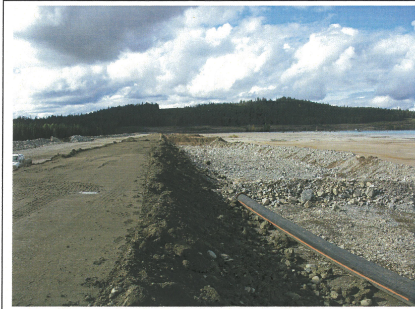
PHOTO 1 – Components of the TSF, Zone S (left) Zone U (centre) and Tailings Beach (right)
