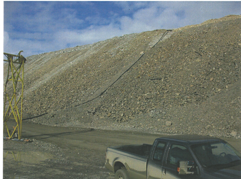
PHOTO 6 – Main Embankment Seepage Pond Return Pipe
