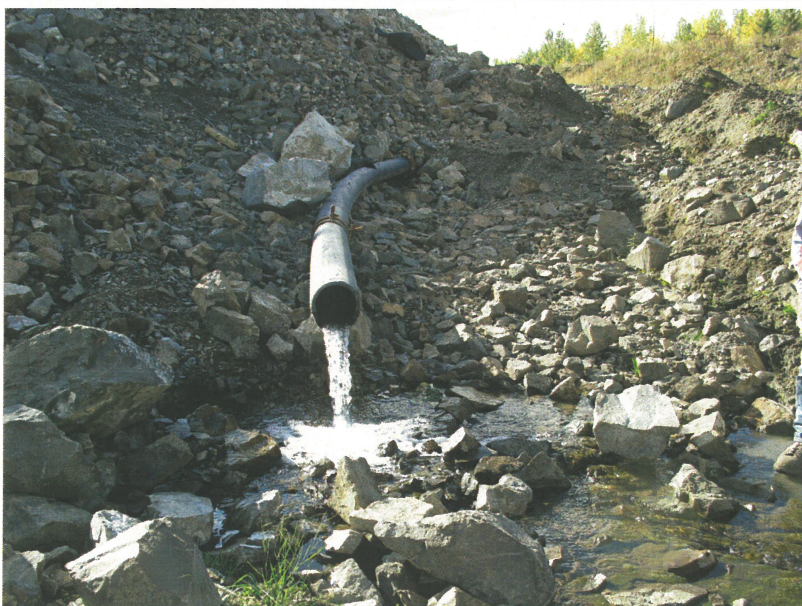
PHOTO 4 – Perimeter Embankment Toe Drain flow running clear
