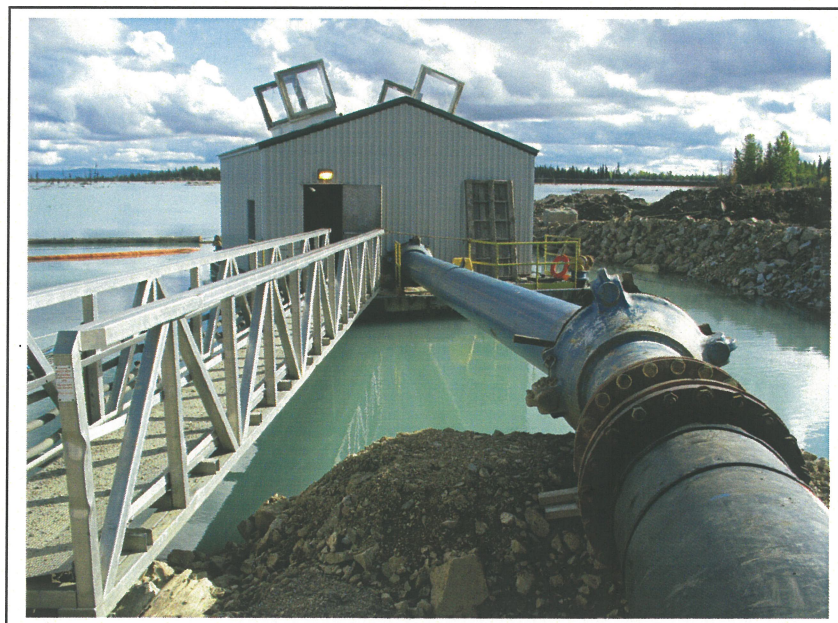
PHOTO 12 – Pump barge and reclaim pipeline
