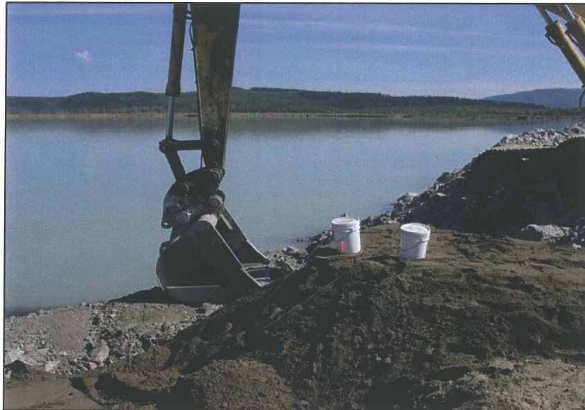
PHOTO 27 – Constructing a sand pile for the piezometers with a rock armor.
