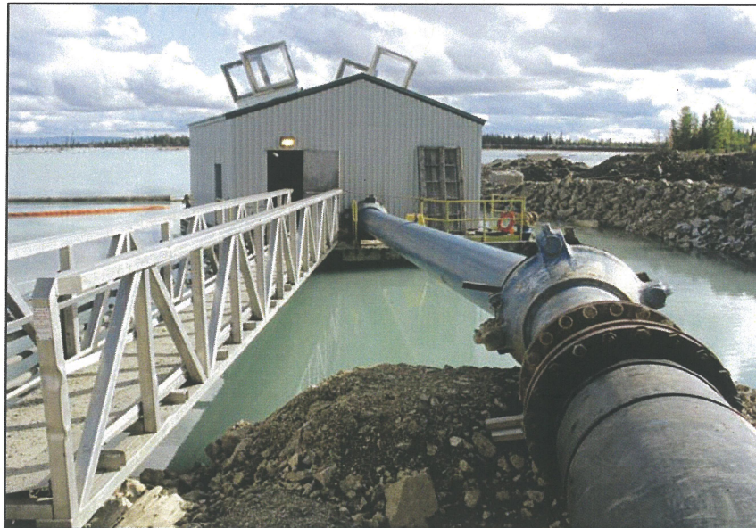
PHOTO 31 – TSF Reclaim Barge.
