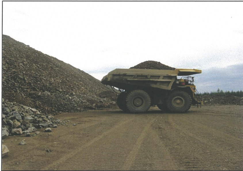
PHOTO 23 – Adding material to the Main Embankment buttress.
