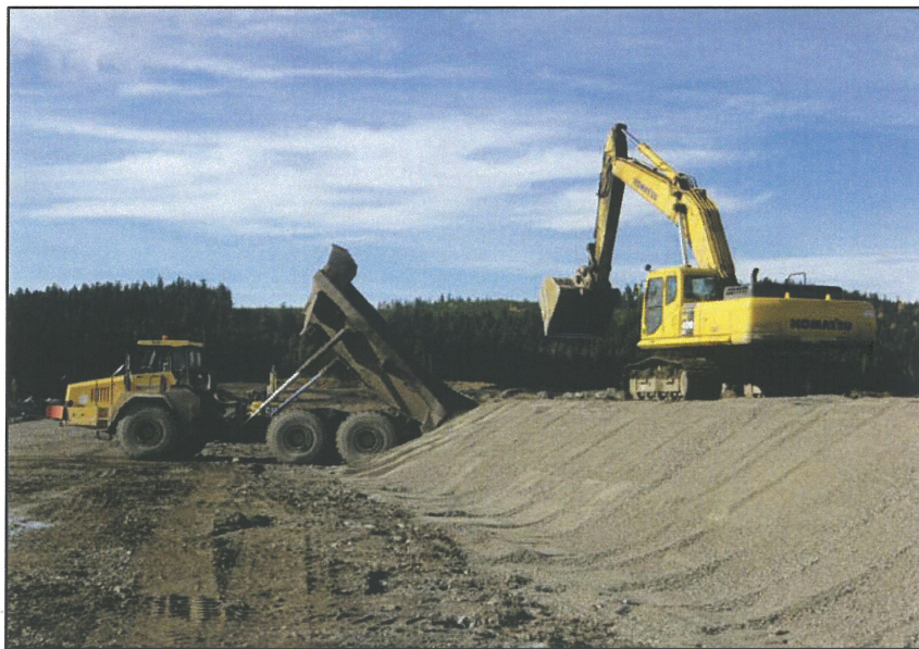
PHOTO 16 – Placing Zone F filter on the 2:1 upstream slope.
