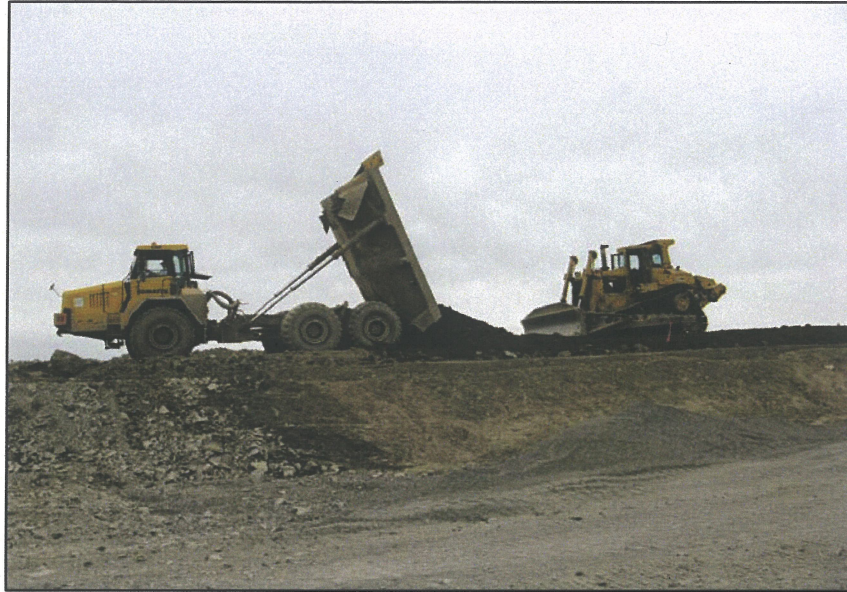
PHOTO 3 – Placing Till (Zone S) on the Tailings Dam
