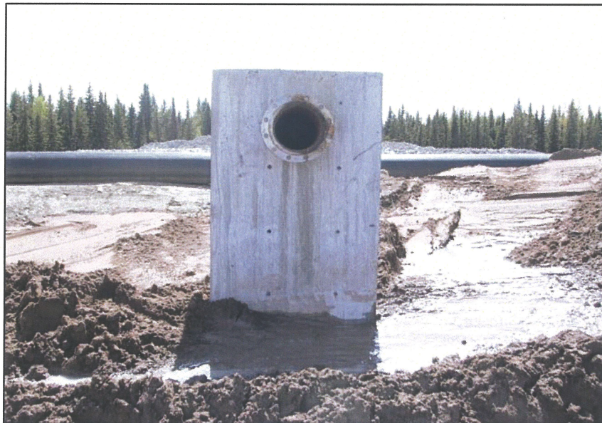
PHOTO 28 – South Embankment toe drain concrete encasement.
