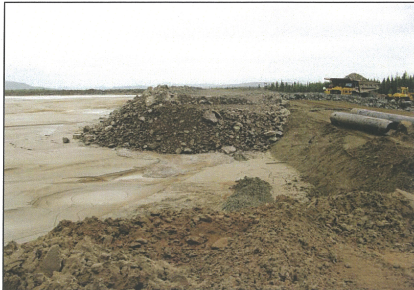
PHOTO 13 – Using pit waste rock to build Zone U.
