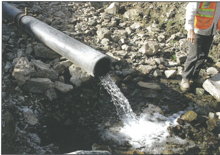
PHOTO 30 – Perimeter Embankment toe drain flows.
