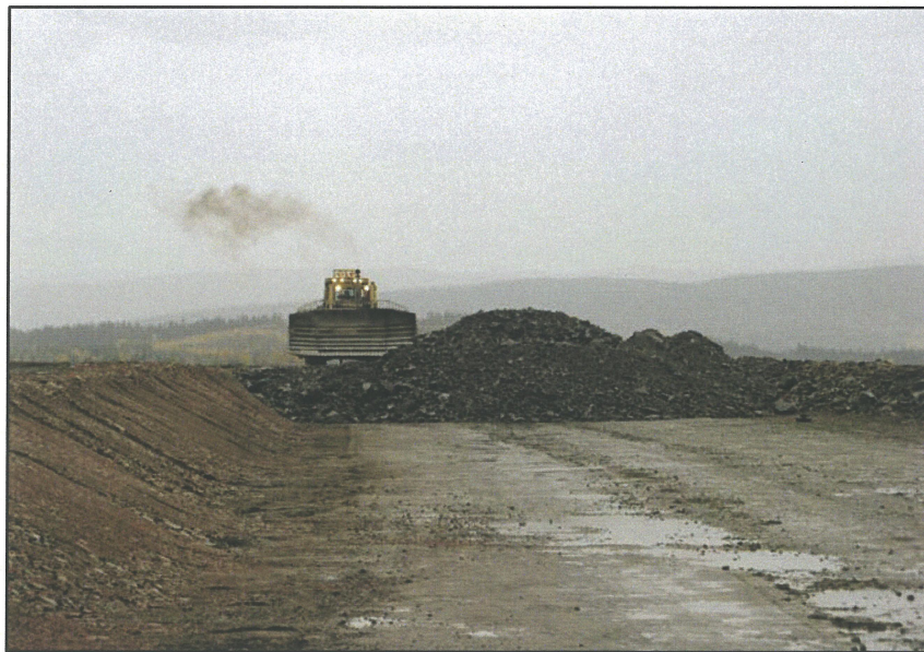
PHOTO 22 – Zone C lifts are kept to less than 2m.
