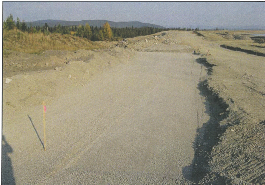
PHOTO 25 – Zone FT material on the Perimeter Embankment abutment
