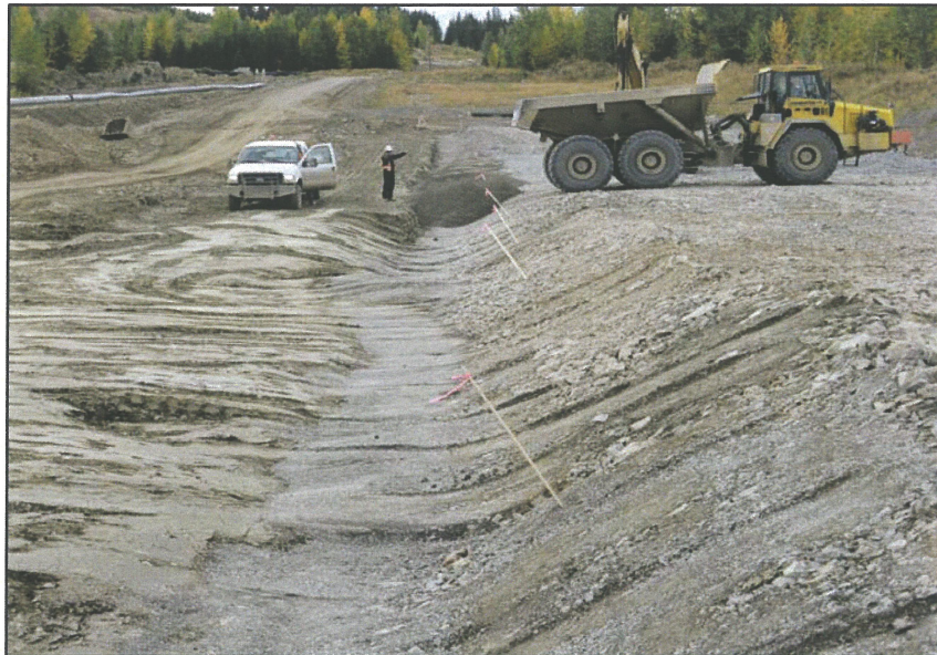
PHOTO 15 – Placing Zone F filter material on the 1.5:1 downstream slope.
