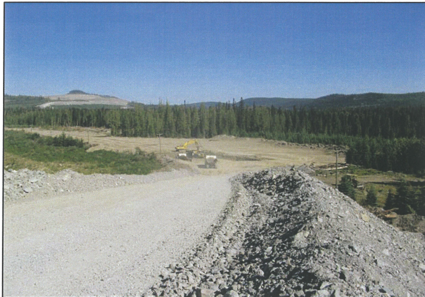
PHOTO 5 – The new Perimeter Embankment Borrow Pit
