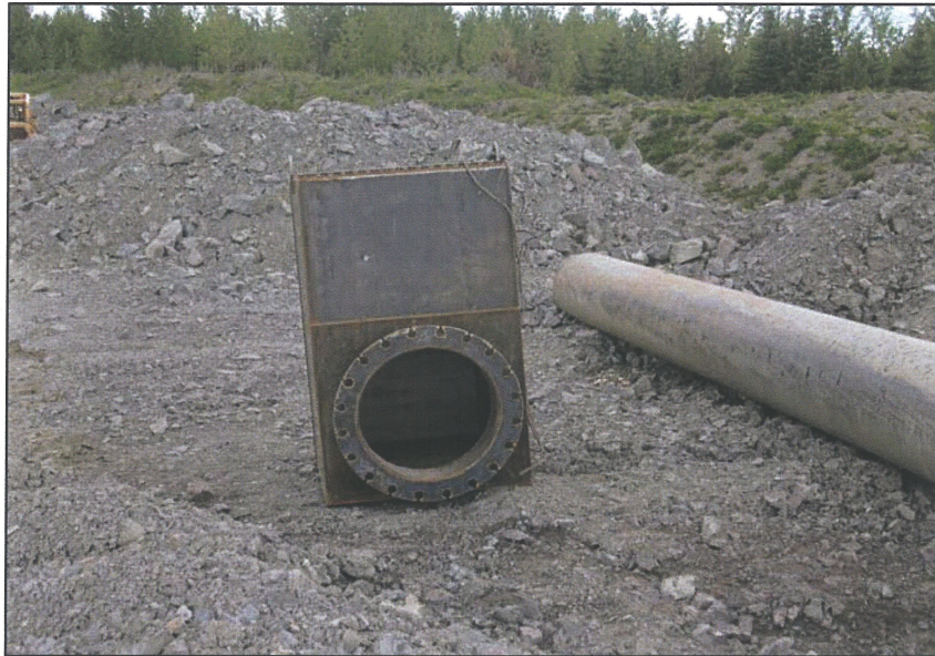
PHOTO 11 – Sand cell decant box showing the drain opening
