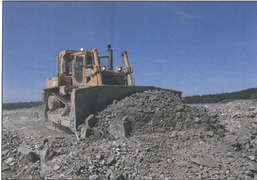
PHOTO 21 – Zone C material is pushed into place by a D8 dozer.
