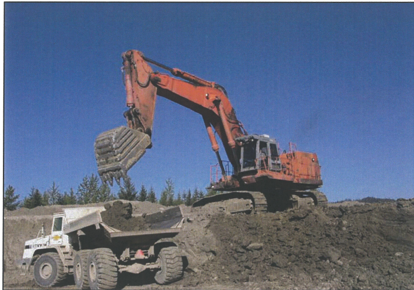
PHOTO 4 – Removing Till (Zone S) from Borrow Area 2
