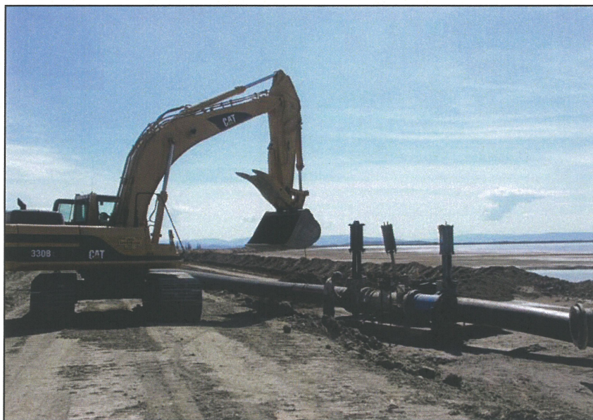
PHOTO 14 – Moving the valve sled in preparation for sand cell construction.
