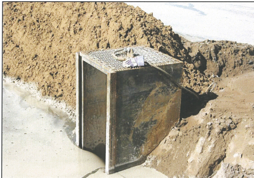
PHOTO 12 – Sand cell decant box. Note the control is at the entry to the box.
