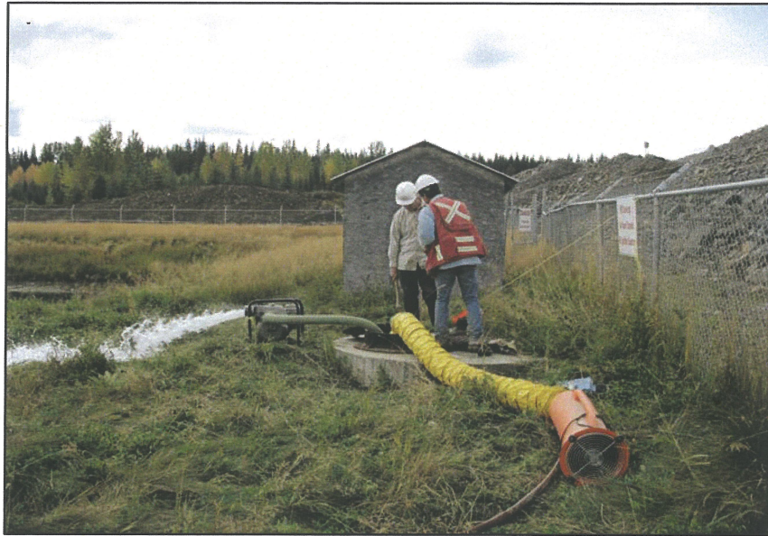
PHOTO 29 – Main Embankment seepage pond sump.
