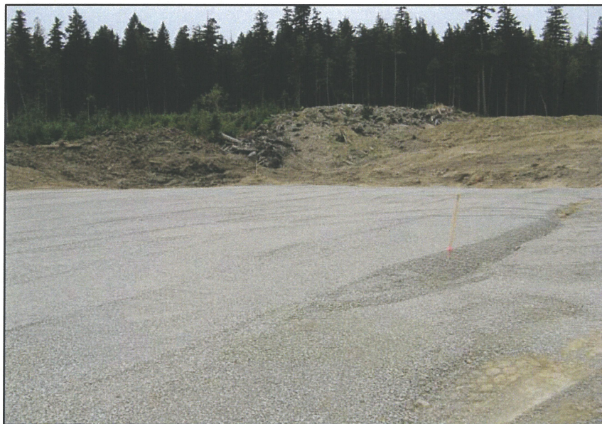
PHOTO 24 – Zone FT on the South Embankment abutment.
