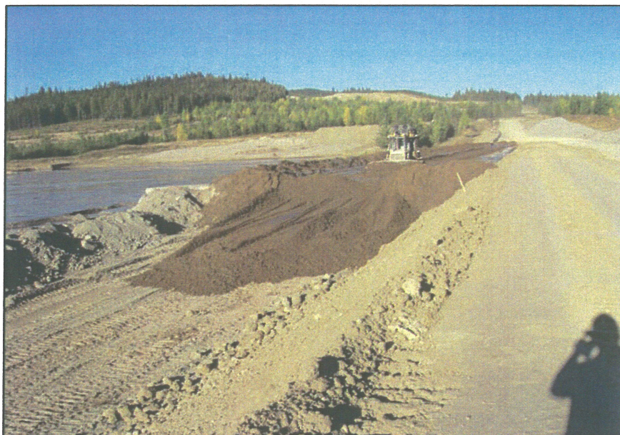
PHOTO 5 – Sand cell production along the Perimeter Embankment
