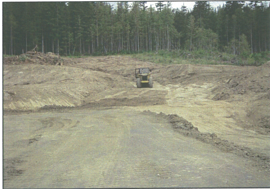
PHOTO 46 – Preparing the north end of the South Embankment for placement of Zone S material.
