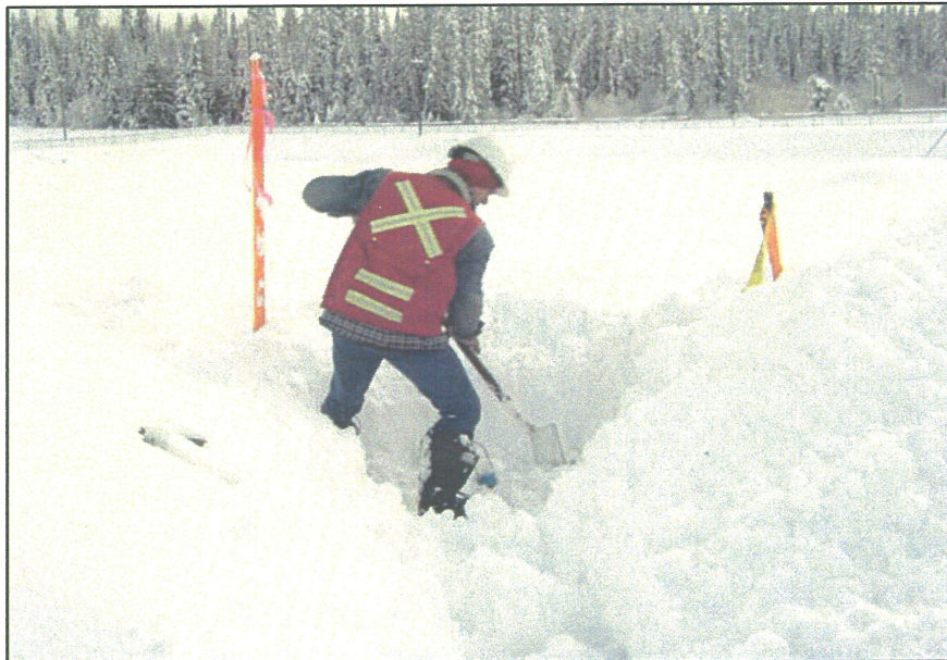
PHOTO 30 – Uncovering an inclinometer
