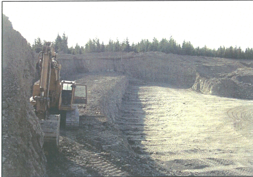
PHOTO 37 – Taking till from Borrow Area No. 3
