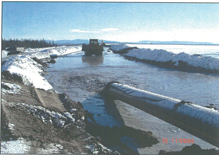
PHOTO 4 – Sand cell production along the Perimeter Embankment
