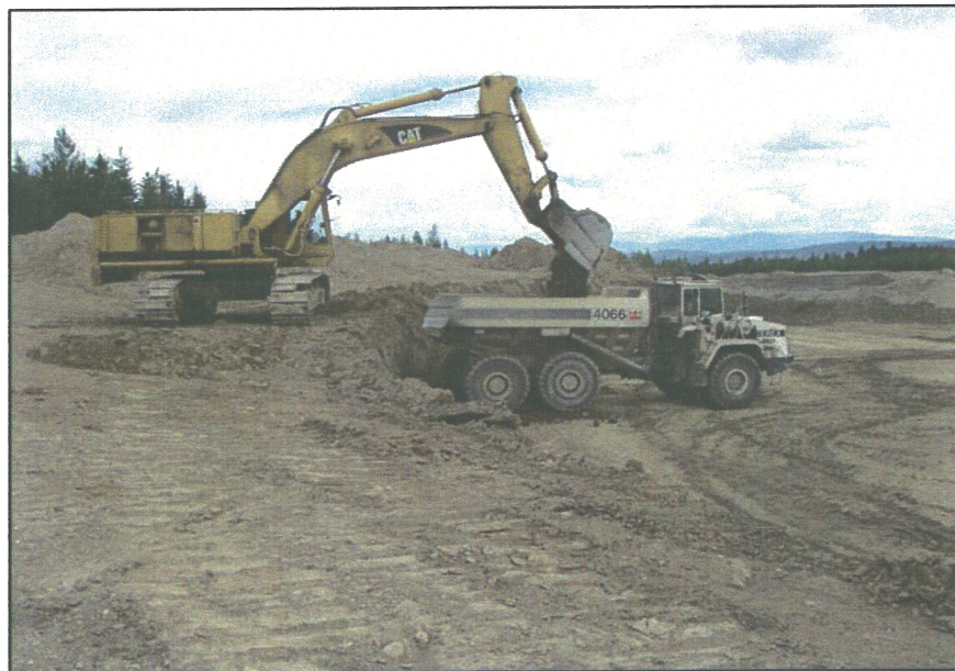
PHOTO 38 – Loading till from Borrow Area No. 4
