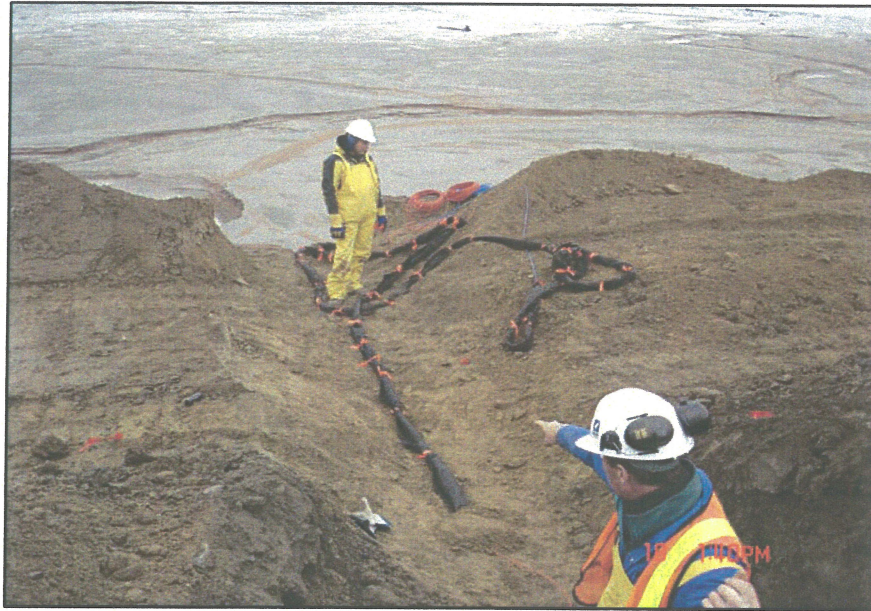
PHOTO 7 – Tailings Piezometer Installation in the Perimeter Embankment
