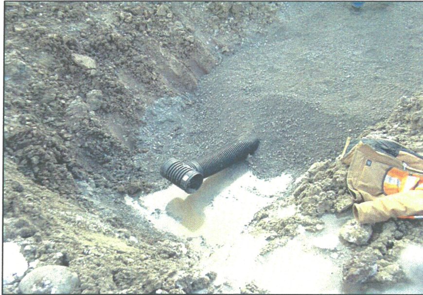
PHOTO 27 – Section connecting the South Embankment longitudinal drain to the toe drain
