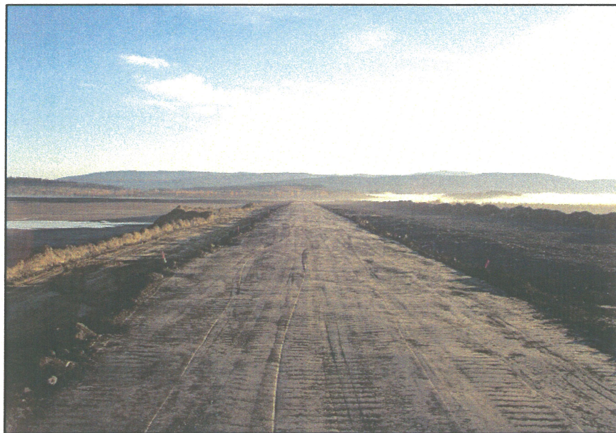
PHOTO 48 – Looking eastward along the Main Embankment with Zone S up to 951 m.
