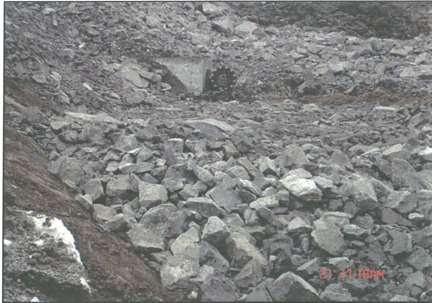
PHOTO 21 – The discharge point of the steel pipe
