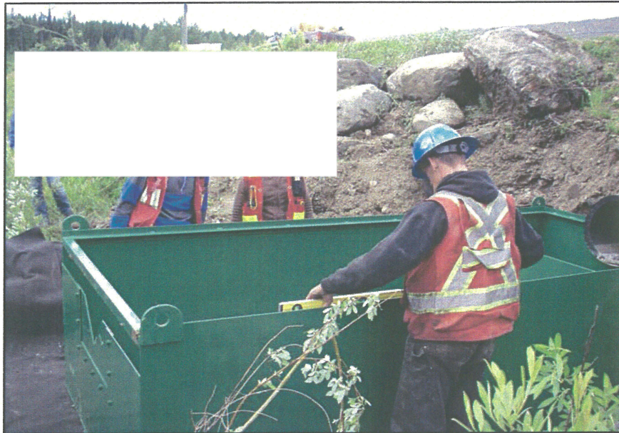
PHOTO 35 – Leveling the weir box, which will be used to measure flows exiting the Main Seepage Pond once a permit is received.
