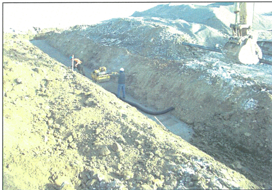
PHOTO 26 – Compacting Zone F material around the longitudinal drain
