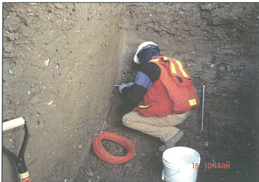
PHOTO 6 –Piezometer Installation
