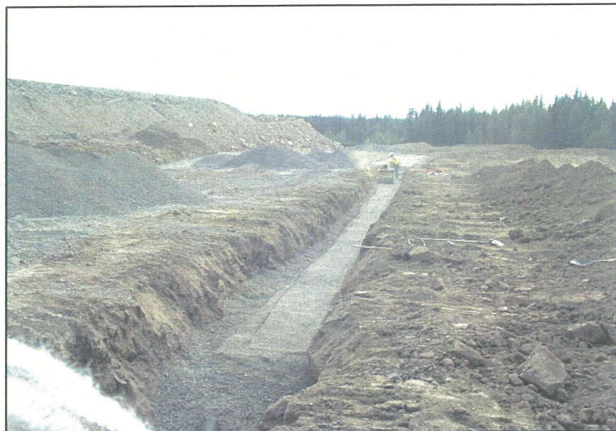
PHOTO 41 – Compacting the Zone F material around the South Embankment foundation drain
