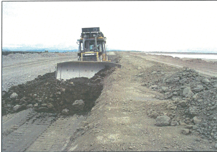
PHOTO 43 – Keying in to the till in the underbuilt sections, to sufficiently blend the new and existing tills.
