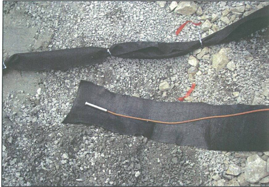
PHOTO 9 – Wrapping a vibrating wire piezometer in geotextile for protection
