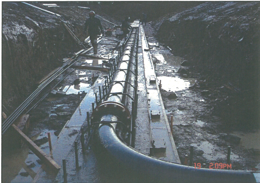
PHOTO 16 – Steel pipe to be joined to the Perimeter Embankment upstream toe drain
