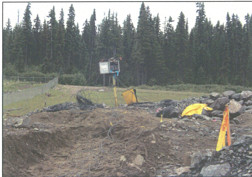
PHOTO 12 – Placing the piezometers in a read-out box for more efficient data collection
