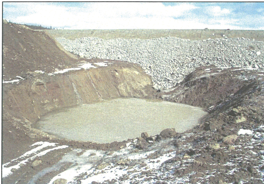
PHOTO 28 – Larger view of South Embankment sump.
