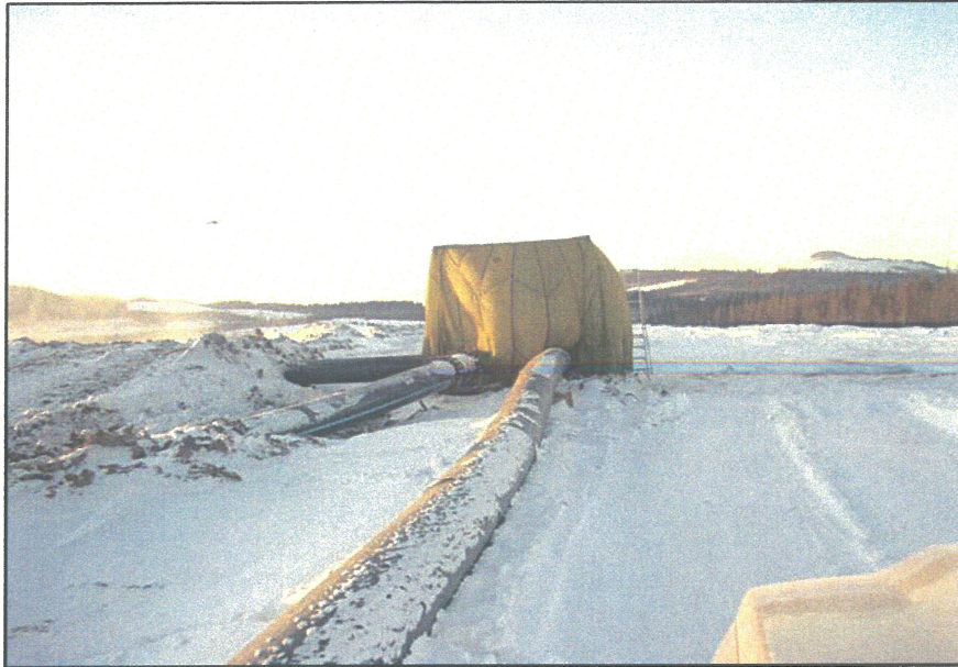
PHOTO 31 – Heating the tailings pipeline valves during the winter months to prevent them from freezing
