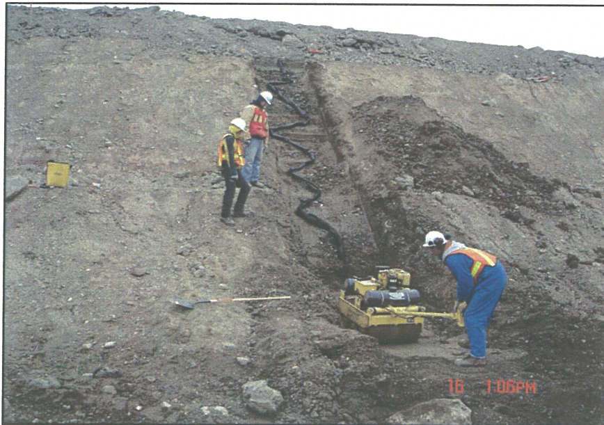
PHOTO 8 – Piezometer Installation in the South Embankment
