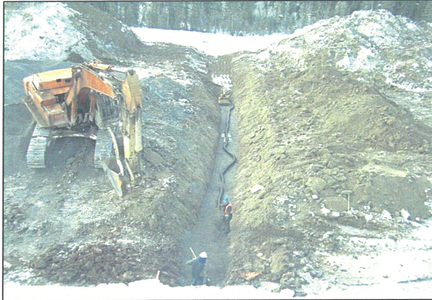
PHOTO 25 – Installing the longitudinal drain to be connected to the South Embankment toe drain
