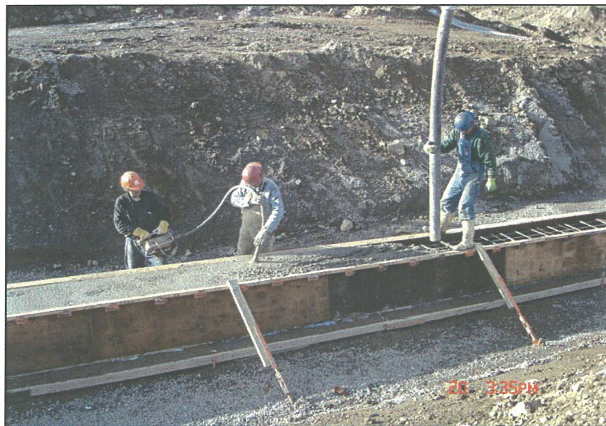
PHOTO 18 – Pouring the concrete to form the encasement
