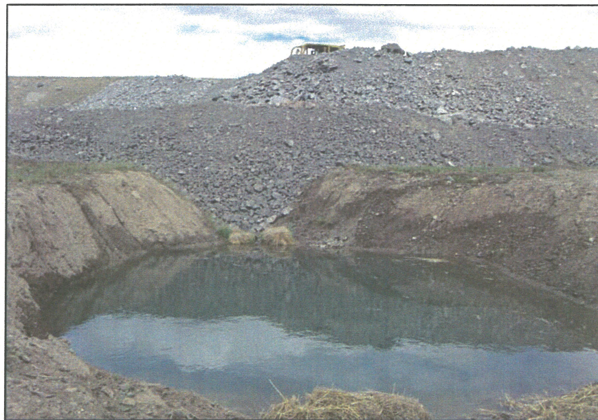
PHOTO 24 – South Embankment sump, collecting water from the downstream slope and subsequently released to the environment.
