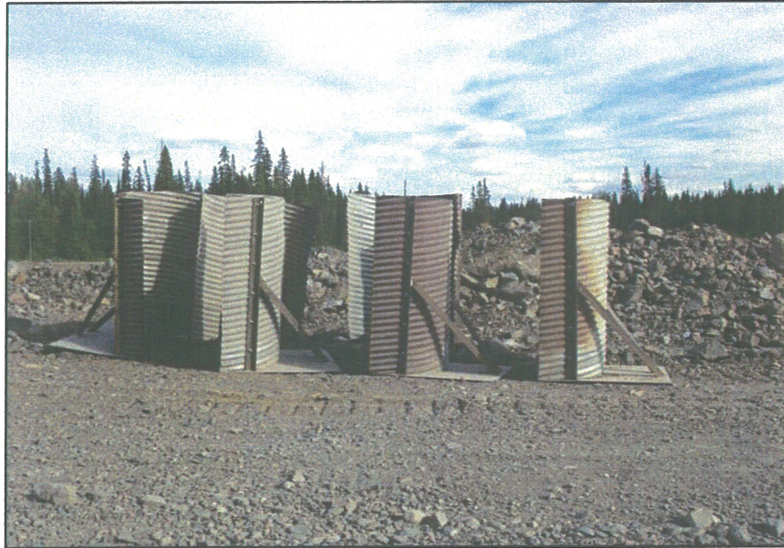
PHOTO 11 – Protective covers for the piezometers located at the Main Embankment toe, to shield them from loose Zone C material
