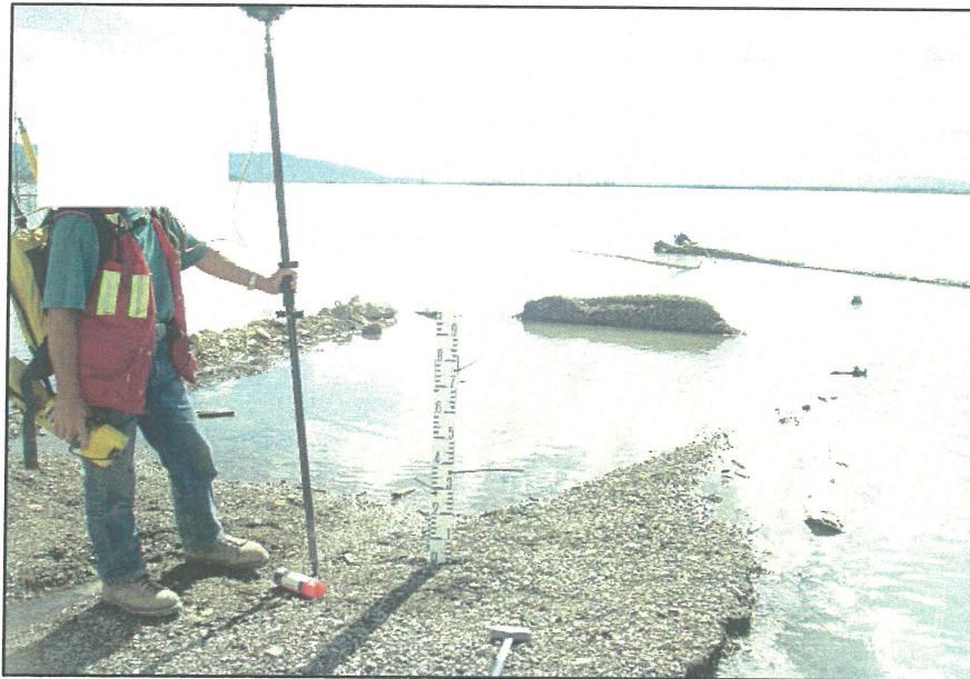
PHOTO 3 – Performing a weekly water elevation reading at the reclaim barge.
