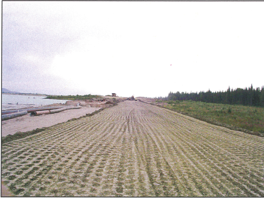
PHOTO 21 – Scarifying the Zone S material at the South Embankment with a sheepsfoot prior to placing the next lift.
