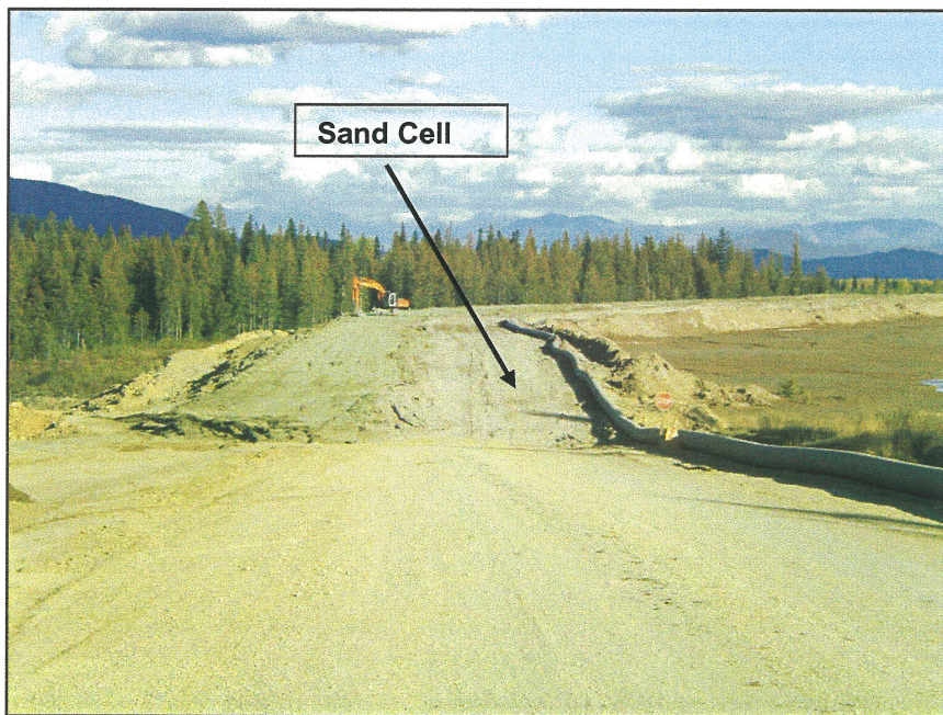
PHOTO 32 – Perimeter Embankment. The Zone U was completed using sand cell construction.
