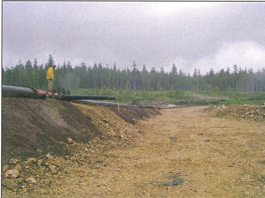
PHOTO 8 – South Embankment sand cell.
