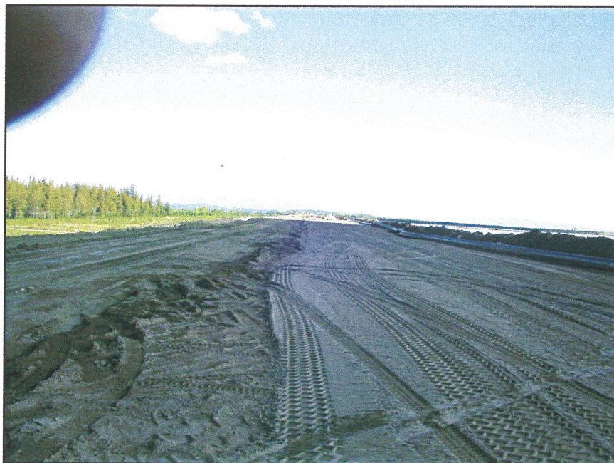
PHOTO 17 – Completed sand cell on the Perimeter Embankment.
