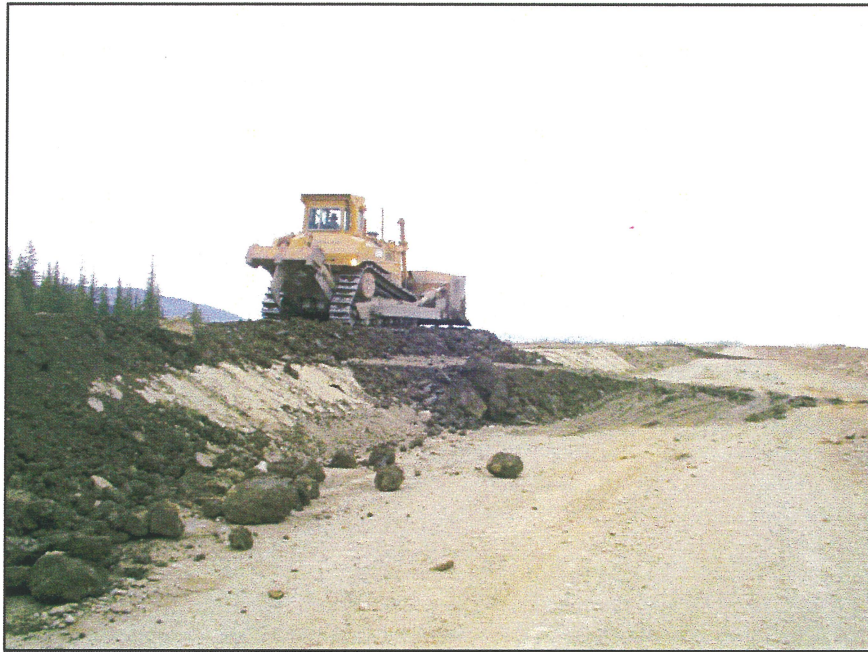
PHOTO 27 –Till ramps were set up to minimize the traffic on the Zone S material with the 777 haul trucks.
