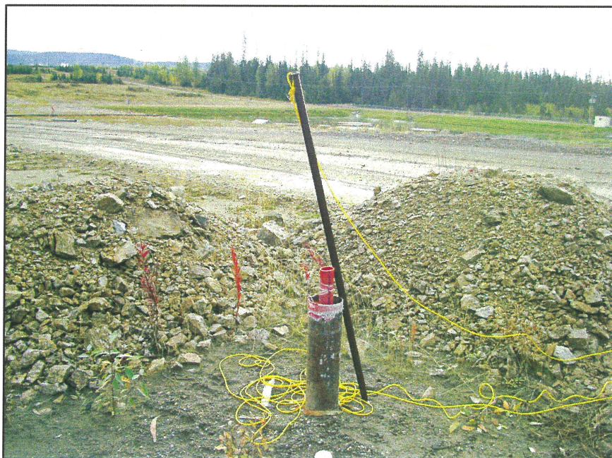
PHOTO 33 – A “poorboy” was used to ensure that there were no “pinch points” in the inclinometers.
