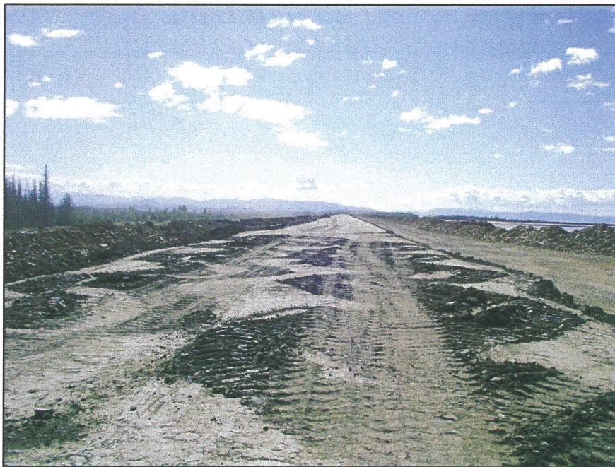
PHOTO 20 – Scarifying the Zone S material at the Perimeter Embankment with a dozer prior to placing the next lift.
