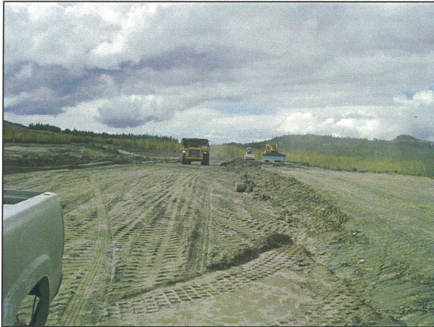
PHOTO 19 – Placing sand from the Cyclone sand stock pile on the Perimeter Embankment as Zone U.
