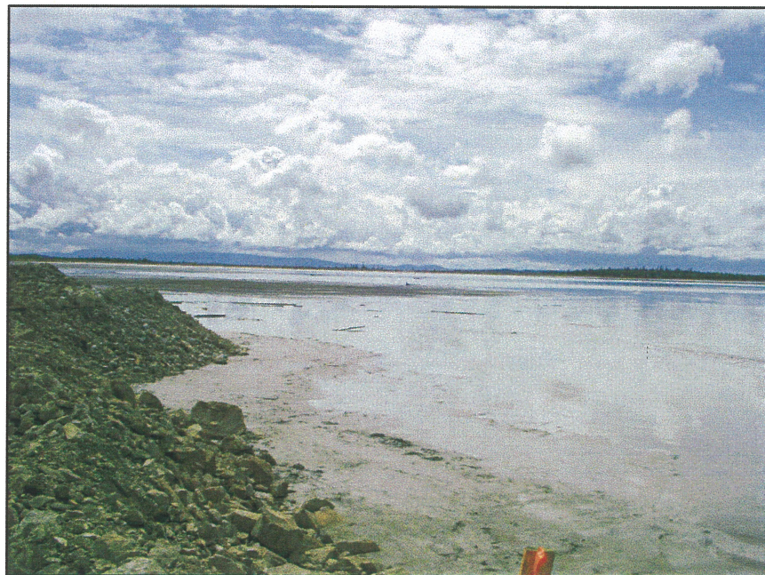
PHOTO 34 – The Mount Polley TSF facing the Main Embankment.
