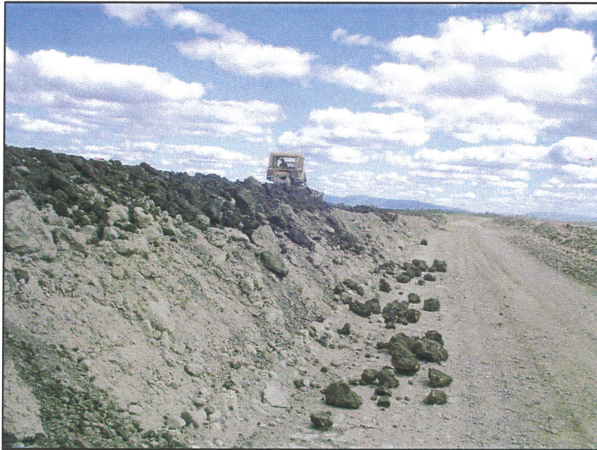
PHOTO 25 – 0.3 m lift of Zone S placed on the Perimeter Embankment.
