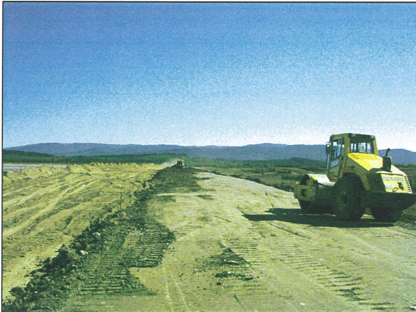
PHOTO 24 – The vibratory smooth drum compacting Zone S material on the Main Embankment.
