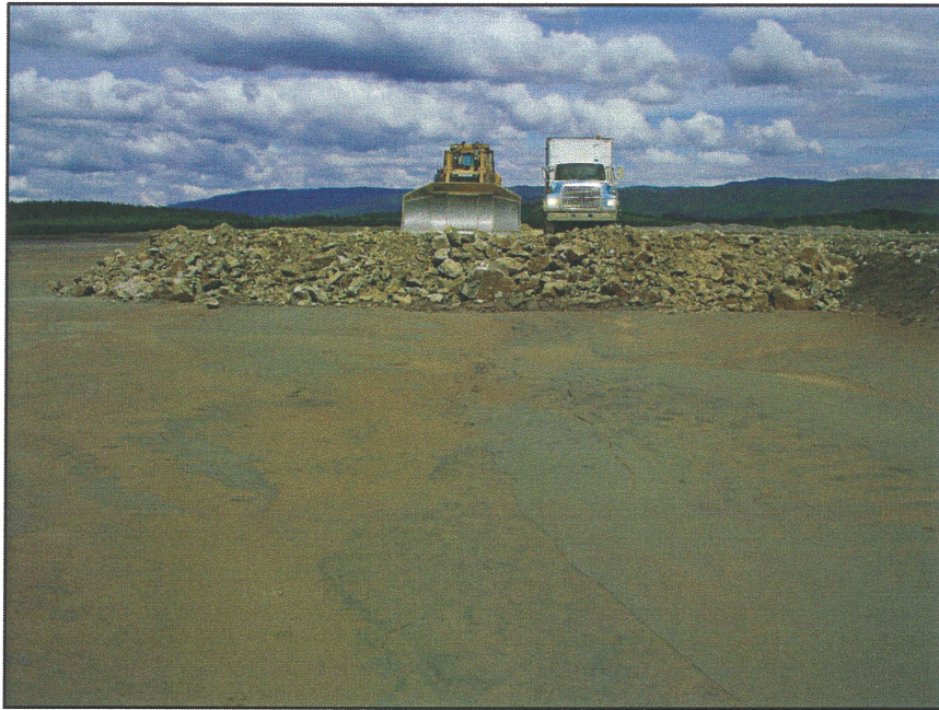
PHOTO 5 – CBL placement on the tailings beach at the Main Embankment.
