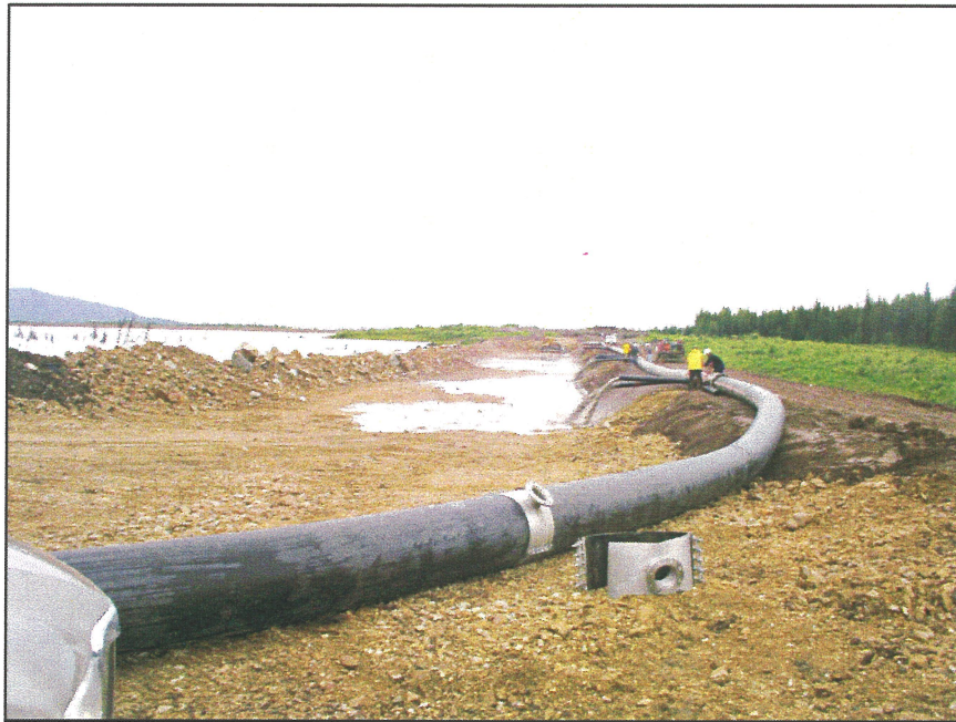
PHOTO 9 – Spigoting tailings into the sand cell at the South Embankment.
