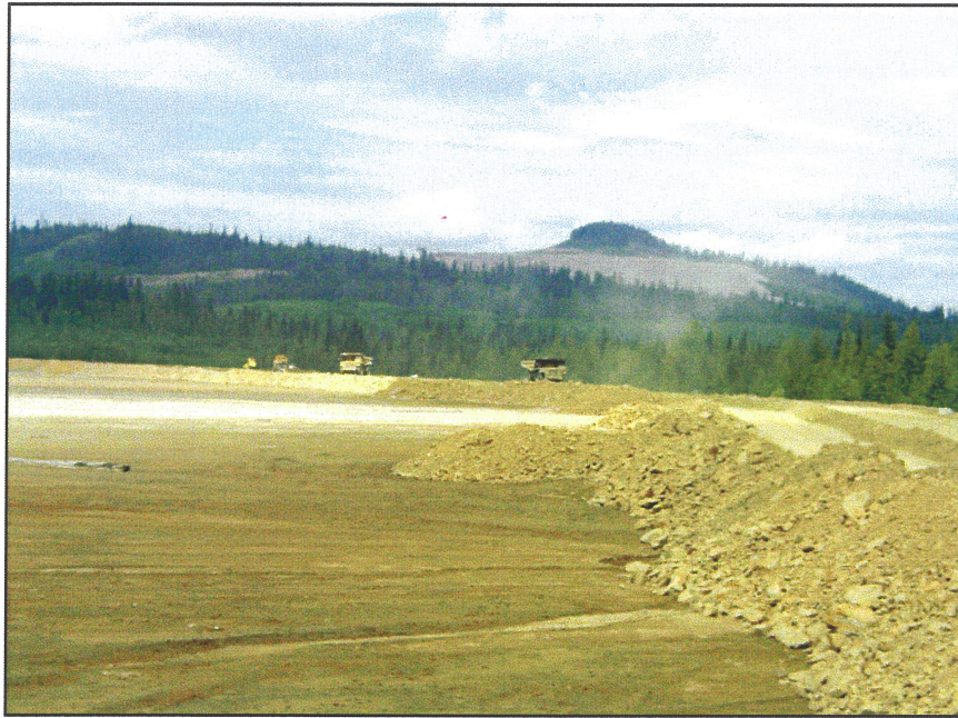
PHOTO 29 – Perimeter Embankment looking up towards the mine.
