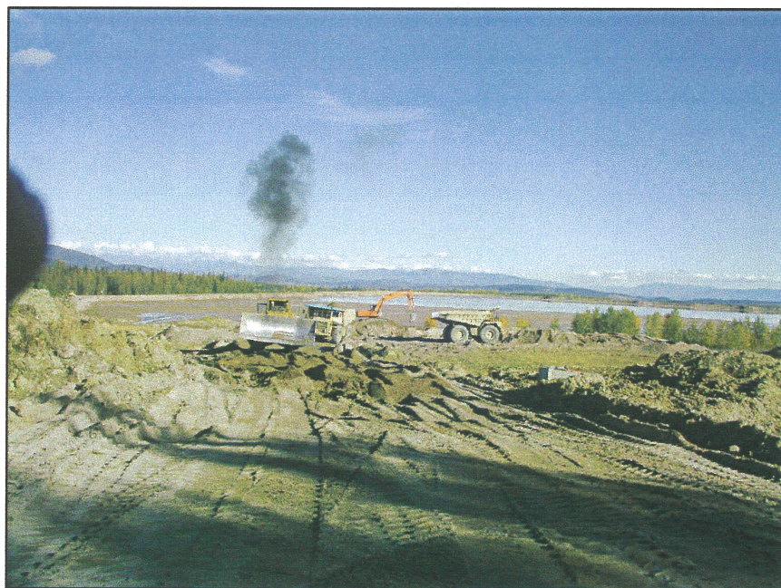
PHOTO 18 – Sand from the Cyclone sand stock pile was also used as Zone U material on the Perimeter Embankment.
