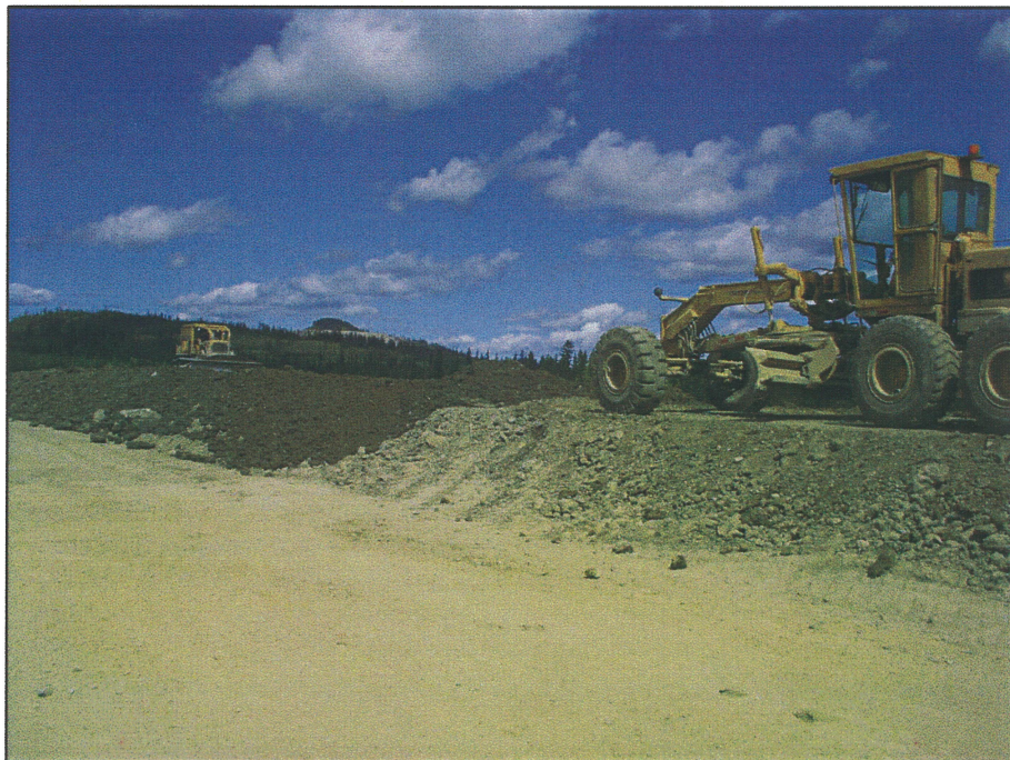
PHOTO 22 – Placing till on the Perimeter Embankment.
