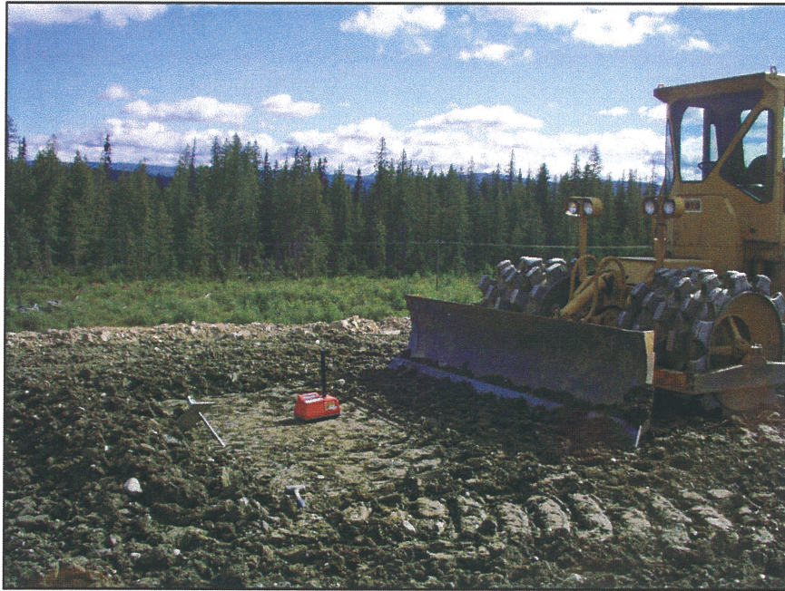
PHOTO 23 – Nuclear densometer testing on the Perimeter Embankment.
