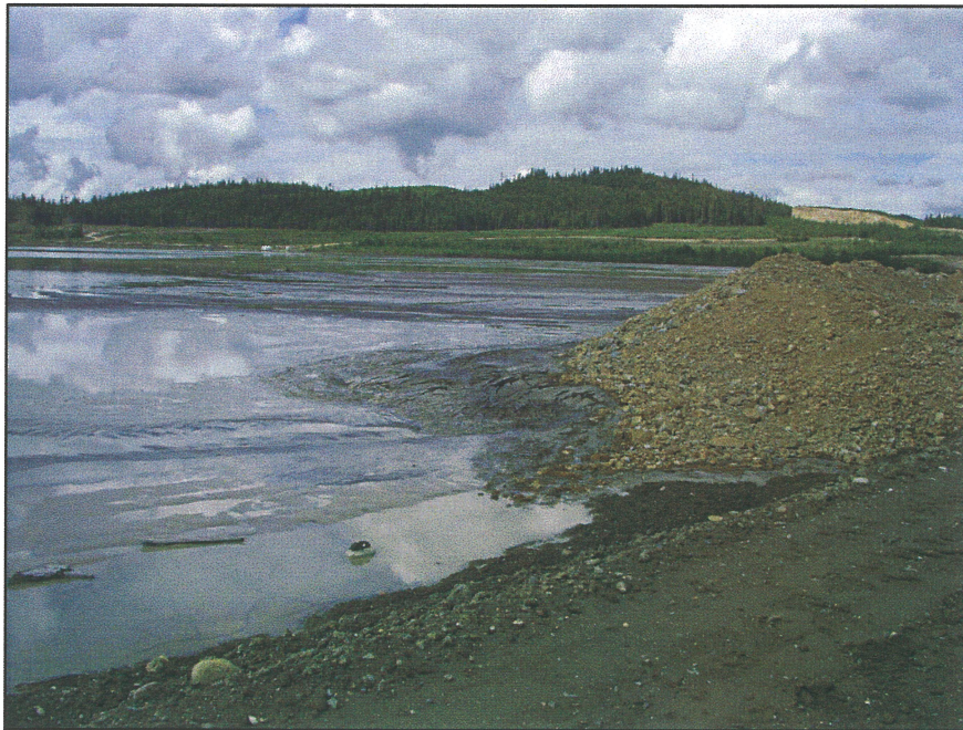
PHOTO 6 –CBL placement on the tailings beach at the Perimeter Embankment.
