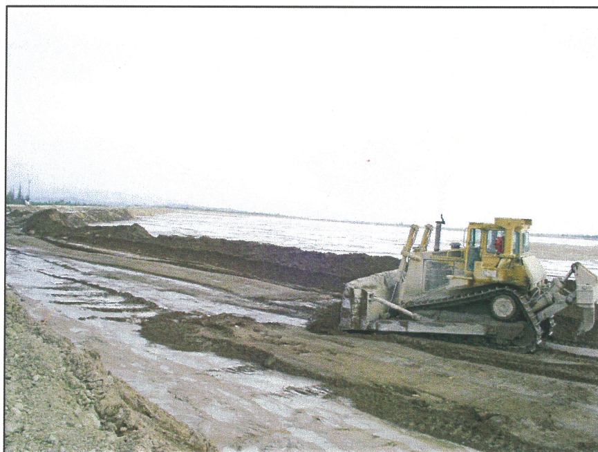
PHOTO 15 – Sand Cell on the Perimeter Embankment.
