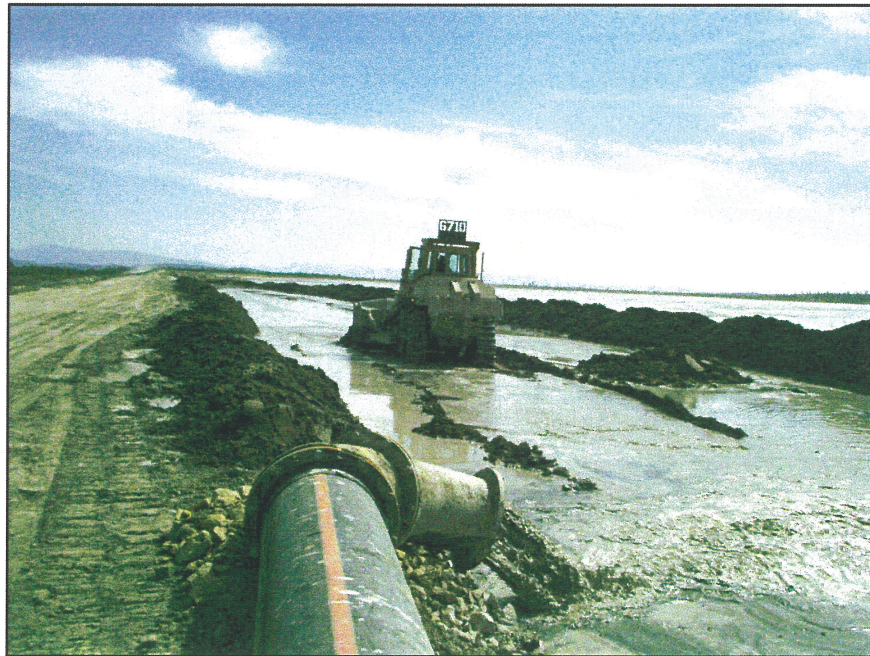
PHOTO 14 – Sand cell on the Perimeter Embankment.
