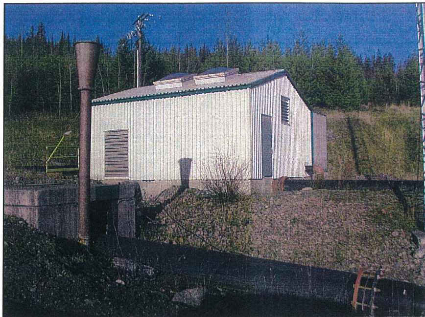
PHOTO # 5 – Reclaim Booster Pumpstation and T2 Dropbox
