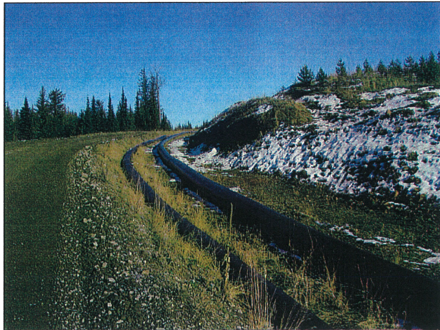
PHOTO # 4 – Tailings and Reclaimed Water Pipelines (View 2)
