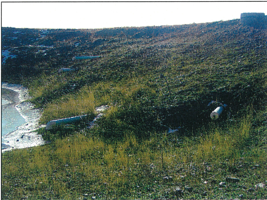
PHOTO # 10 – SE Sediment Pond showing Outlet Pipes
