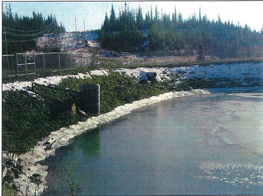
PHOTO # 13 – Mill Site Sump
