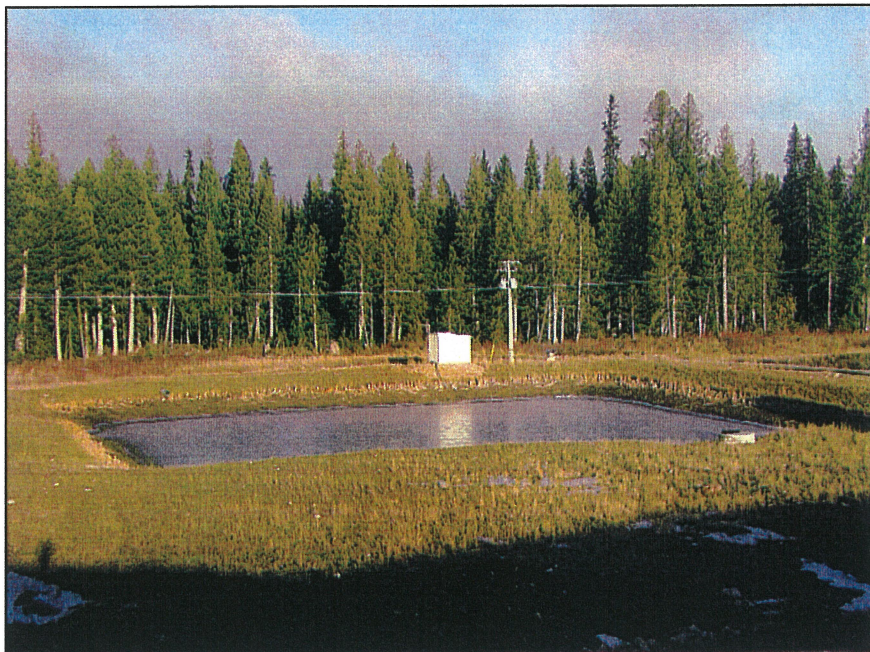
PHOTO # 12 – Perimeter Embankment Seepage Collection Pond
