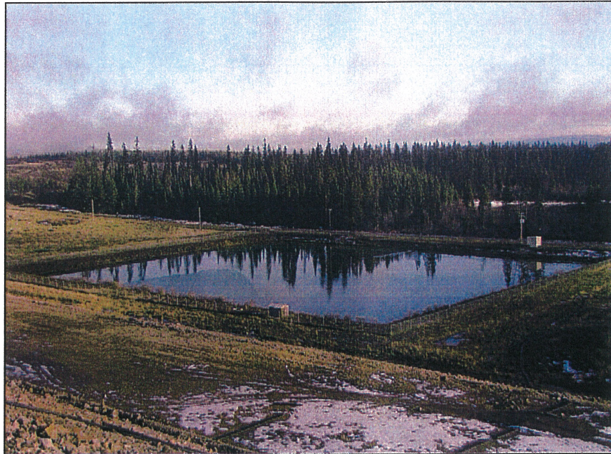
PHOTO # 11 – Main Embankment Seepage Collection Pond
