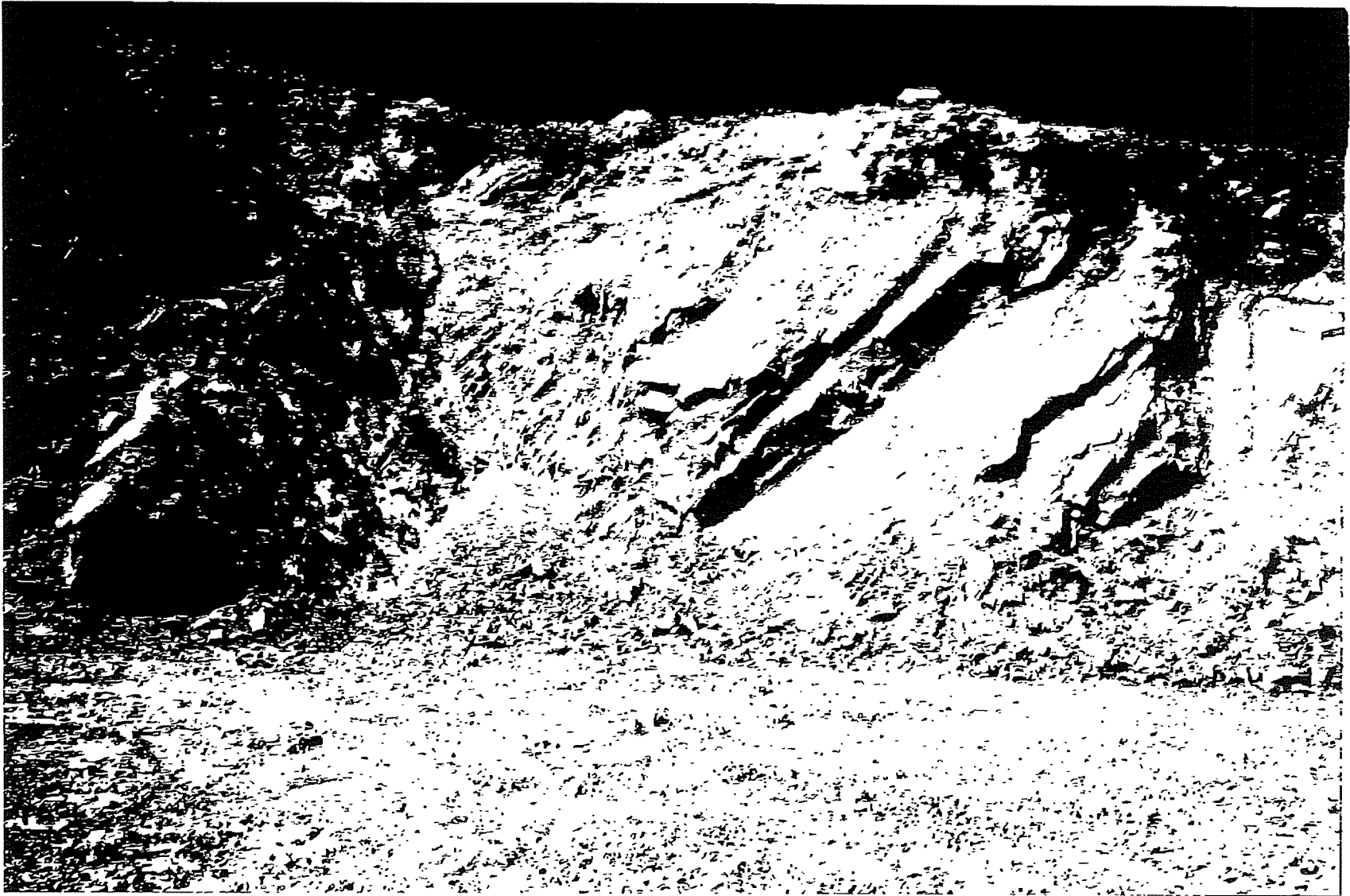
Photograph 1: Northwest Wall. 70 degree bench face angle undercuts Joint Set A causing sliding and slabbing.
