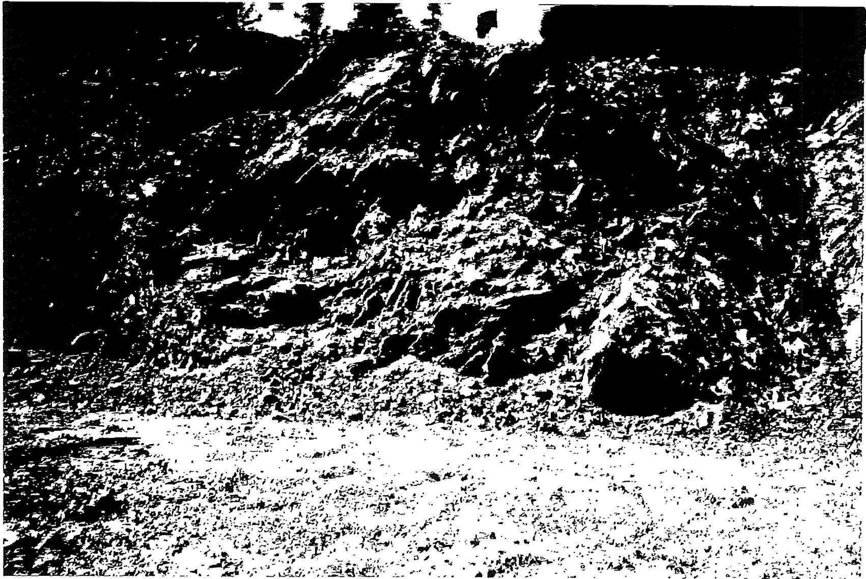
Photograph 2: Southwest Wall. Joint Set B strikes sub-parallel to the wall and forms a back plane for small wedges.
