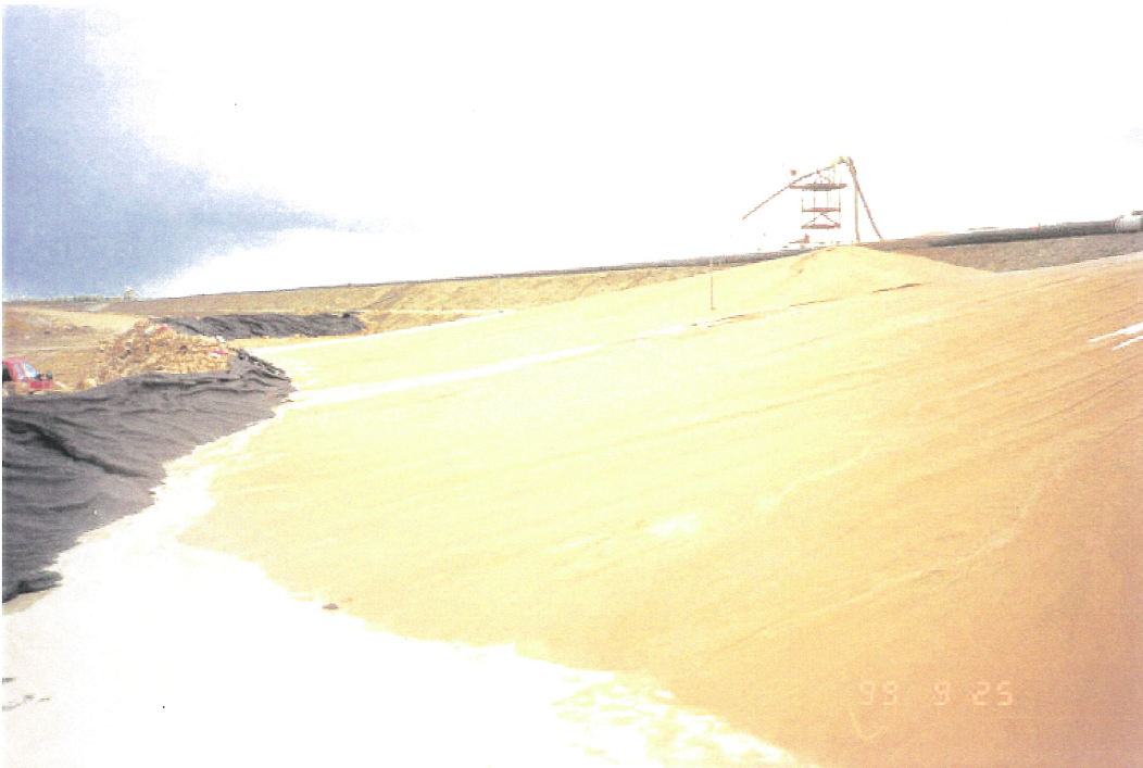
Photo No. 5: Downstream Trial – Phase I cycloned sand deposition.
