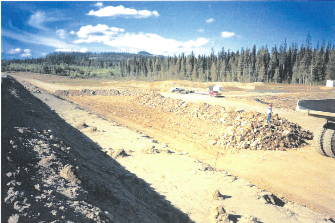
Photo No. 1: Downstream Trial Rockfill Berm.
