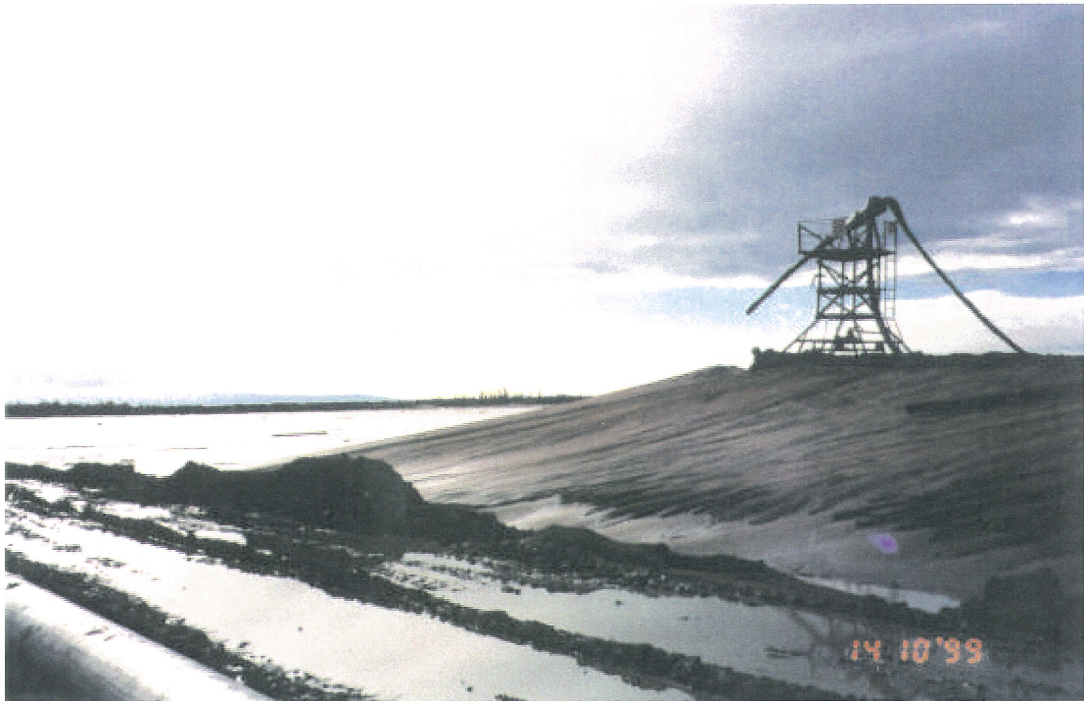
PhotoNo. 4: Perimeter Embankment Upstream Trail Berm.
