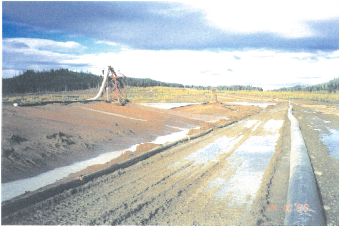
Photo No. 5: Perimeter Embankment Upstream Trial Berm.
