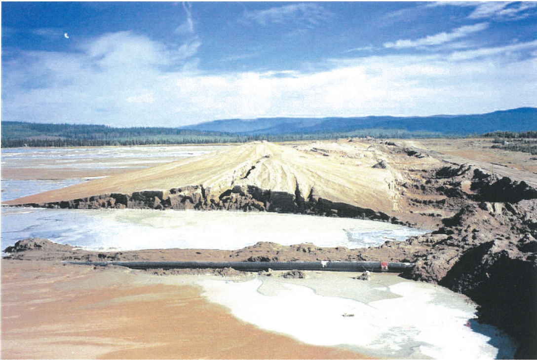
Photo No. 1: Upstream Trial Berm – Main Embankment cycloned sand cone.
