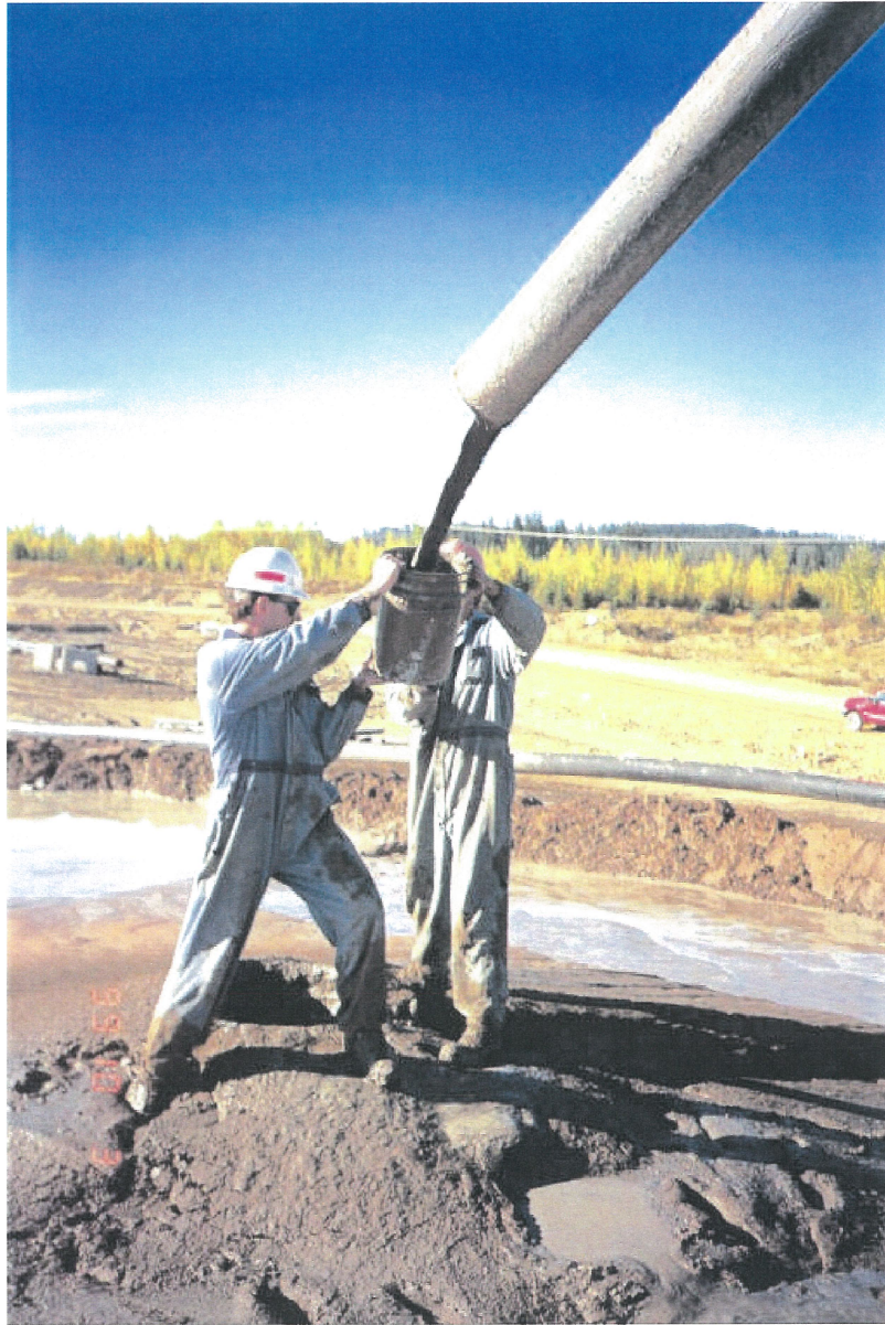
Photo No. 6: Upstream cycloned sand timed discharge bucket test.
