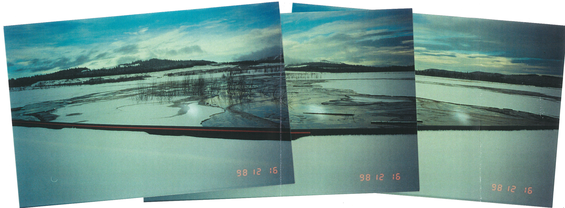
December 16, 1998 - View of the tailings beach looking upstream from the Main Embankment. Bulk tailings are being discharged from the Movable Discharge Section.
