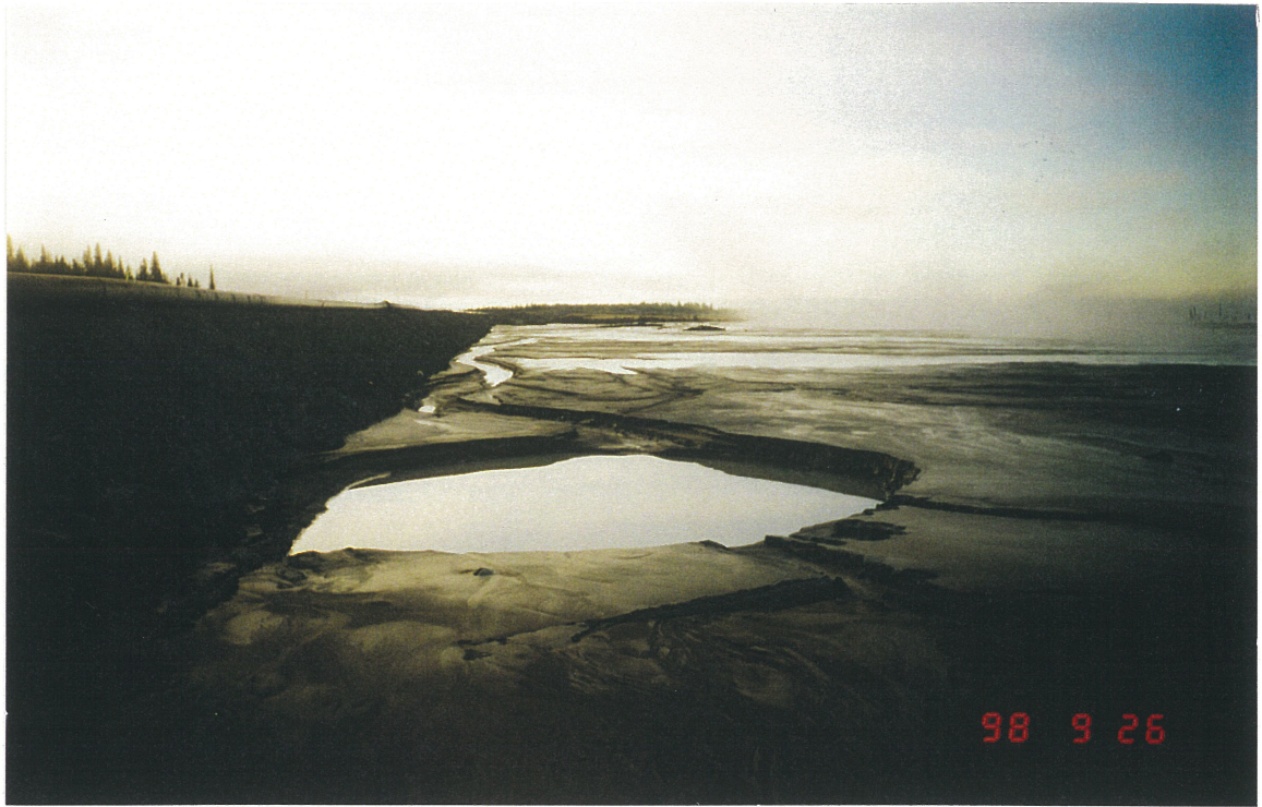
September 26, 1998 - View of the tailings beach looking west along the Main Embankment. Beach developed from discharged of bulk tailings from the Movable Discharge Section.
