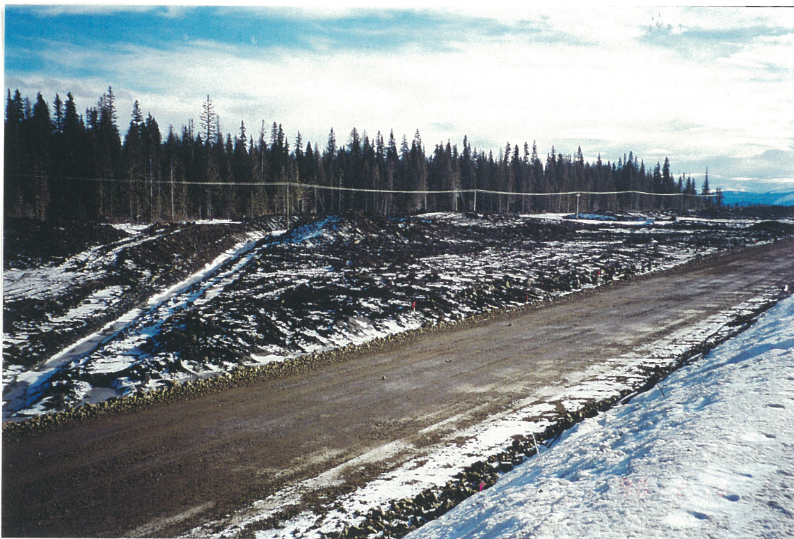
Photo No. 4: Completed Zone T Haul Road at Perimeter Embankment, February 13, 1998.
