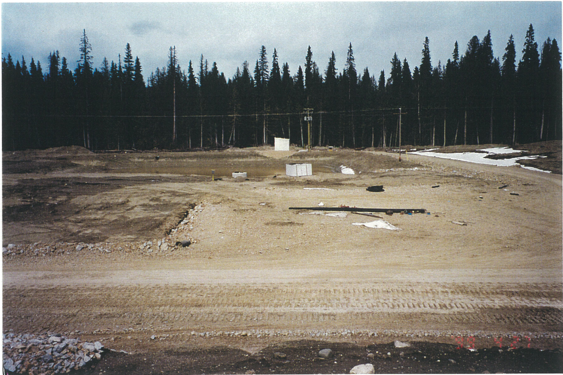
Photo No. 7: Perimeter Embankment. Looking downstream to Seepage Collection Pond. Note grading of area. Zone T platform was extended to final downstream toe.
