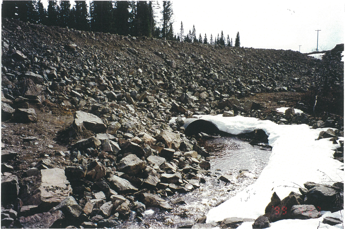
Photo No. 10: Bootjack Creek Culvert. Upstream side.
