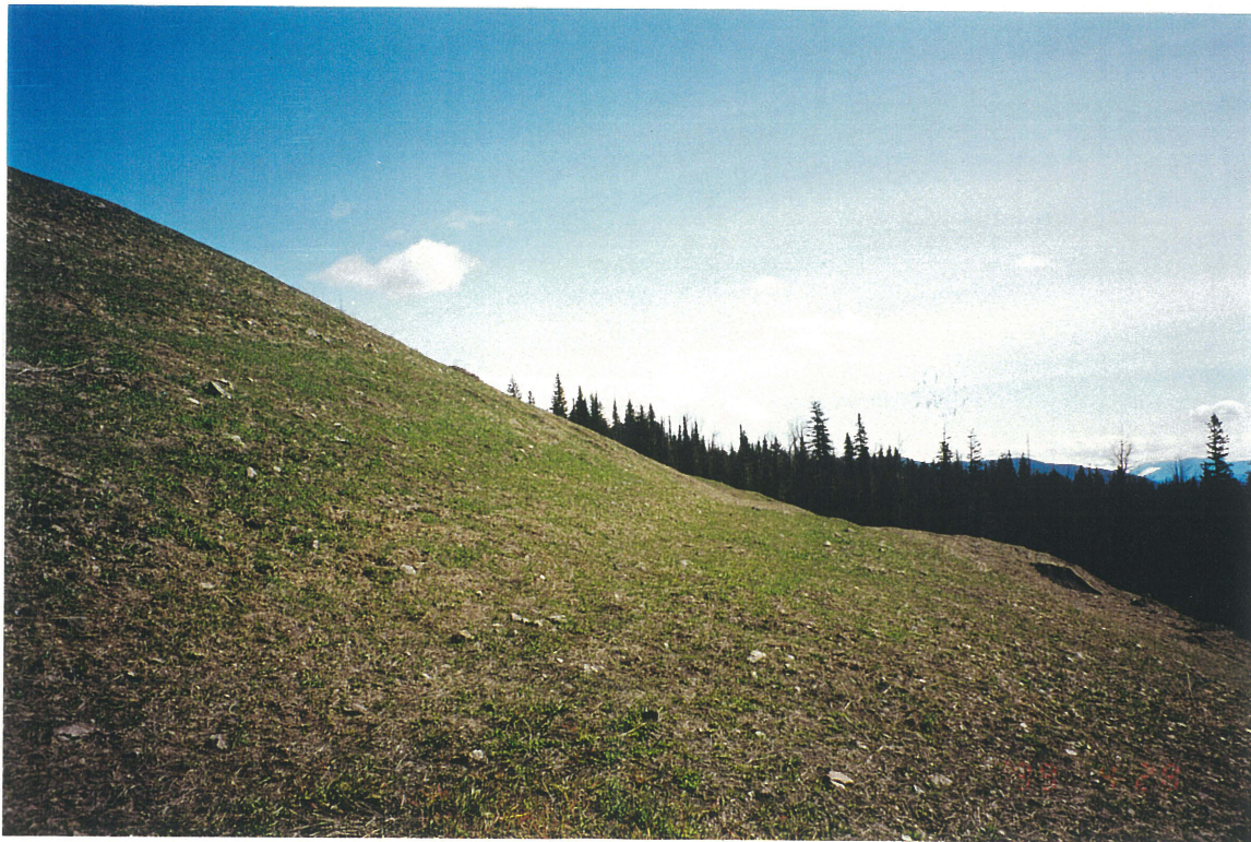
Photo No. 18: Southeast Sediment Pond. Downstream fill slope looking east. Note dry stable slope and well established re-vegetation.
