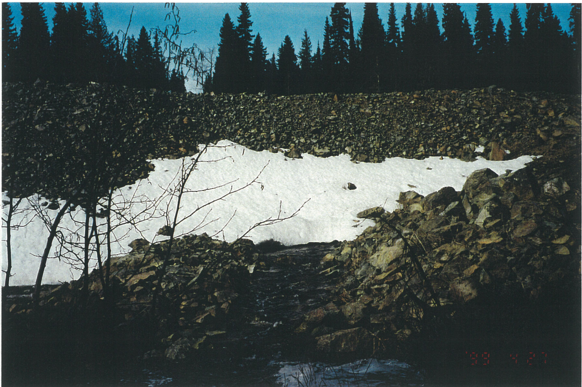
Photo No. 11: Bootjack Creek Culvert. Downstream side.
