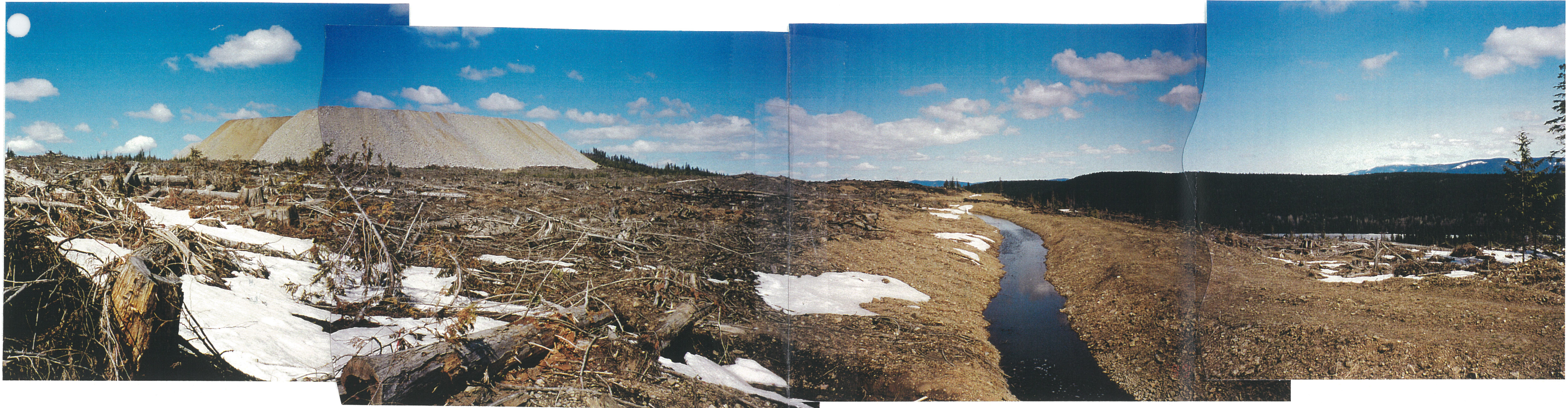
Photo No. 15: Southeast Sediment Pond – Runoff collection ditch, looking north. Note Mine waste dump to left and Polley Lake to right.
