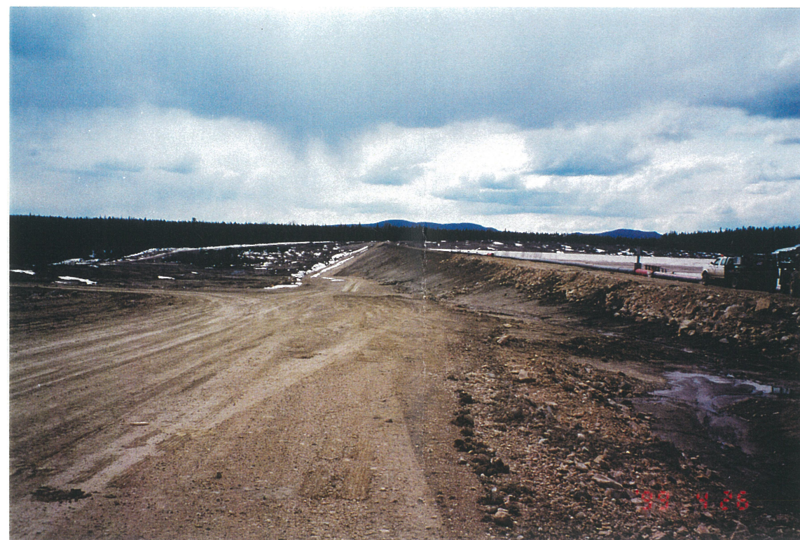
Photo No. 3: Main Embankment. View looking west, from left abutment.
