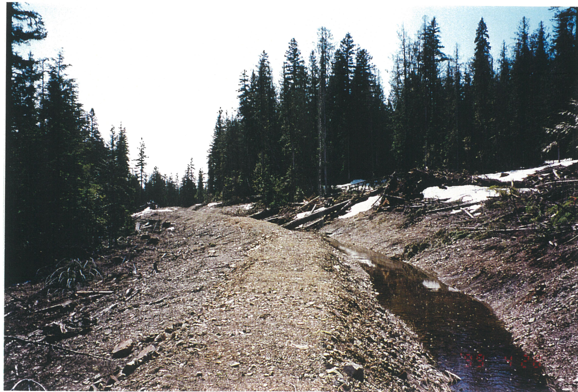
Photo No. 16: Southeast Sediment Pond – Runoff collection ditch, looking south.
