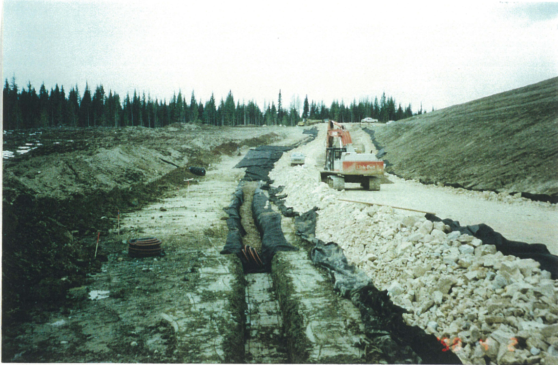
Photo No. 1: Installing Foundation Drain FD-5 at Main Embankment, April 2, 1998.
