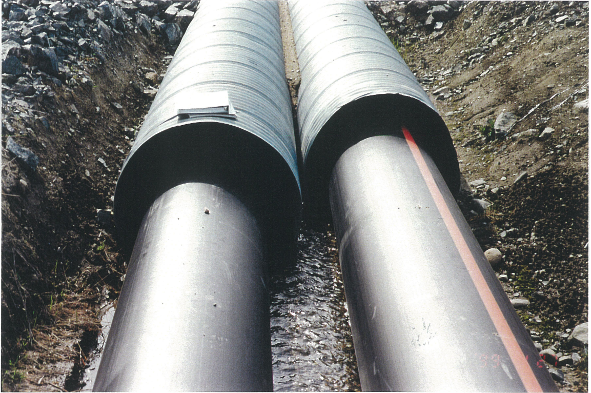
Photo No. 8: Pipeline Containment Channel. Upstream end of pipeline sleeves at Bootjack Creek Crossing. Minor amount of tailings at bottom of sleeves.
