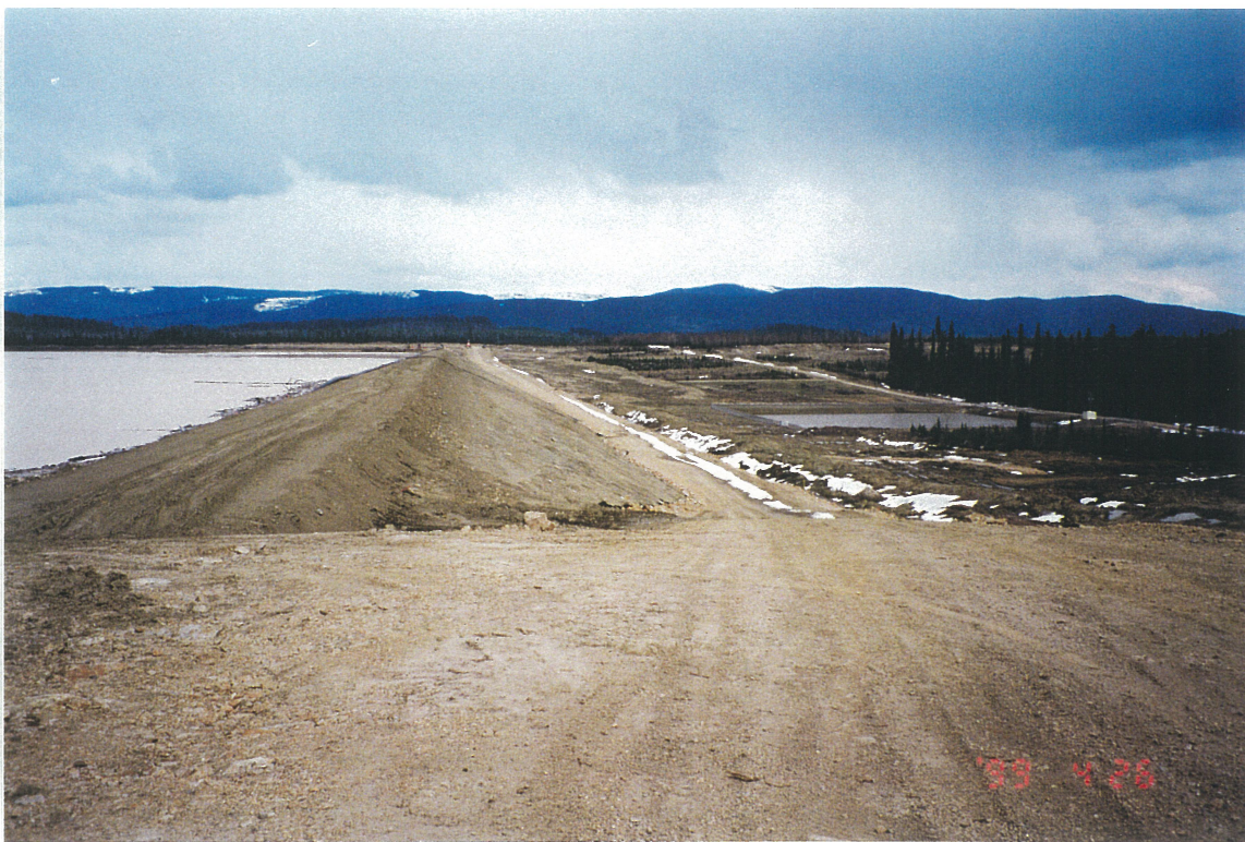
Photo No. 2: Main Embankment. View looking east, from right abutment.
