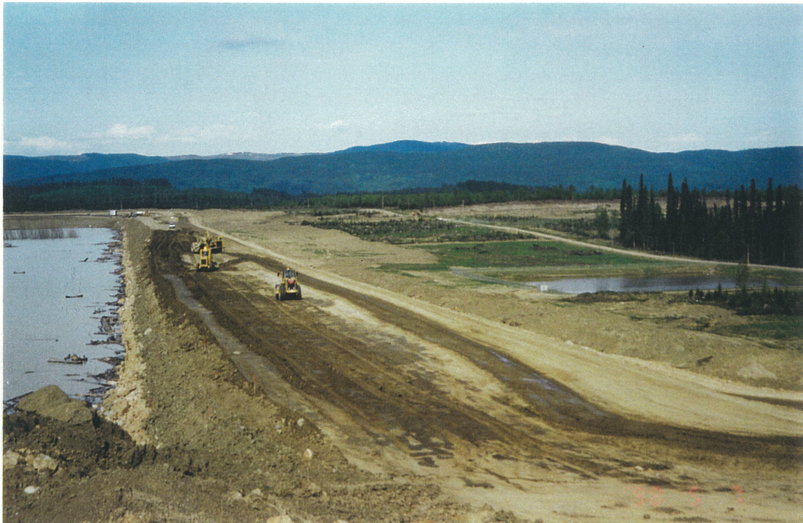
Photo No. 7: Placement of Zone S Glacial Till at Main Embankment, May 7, 1998.
