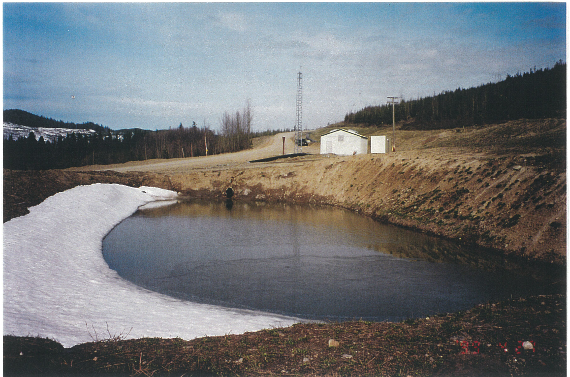
Photo No. 13: Tailings Pipeline System. Full T2 Overflow Pond (water).
