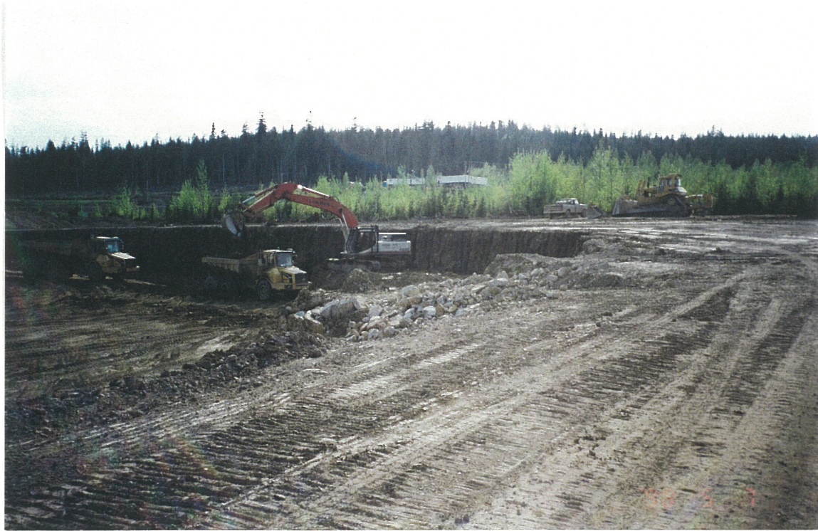
Photo No. 6: Glacial Till Borrow Area 4, near Perimeter Embankment, May 7, 1998.
