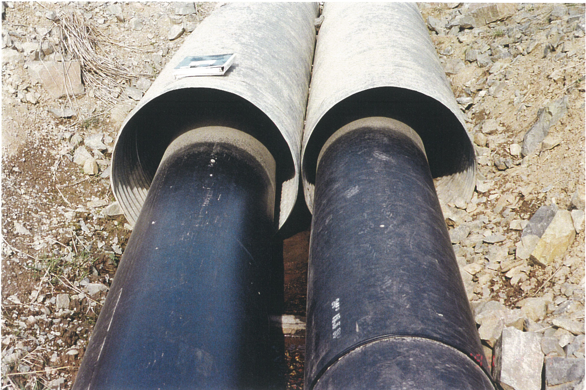
Photo No. 9: Pipeline Containment Channel. Downstream end of pipeline sleeves at Bootjack Creek Crossing. Note minor amount of tailings at bottom of sleeves.
