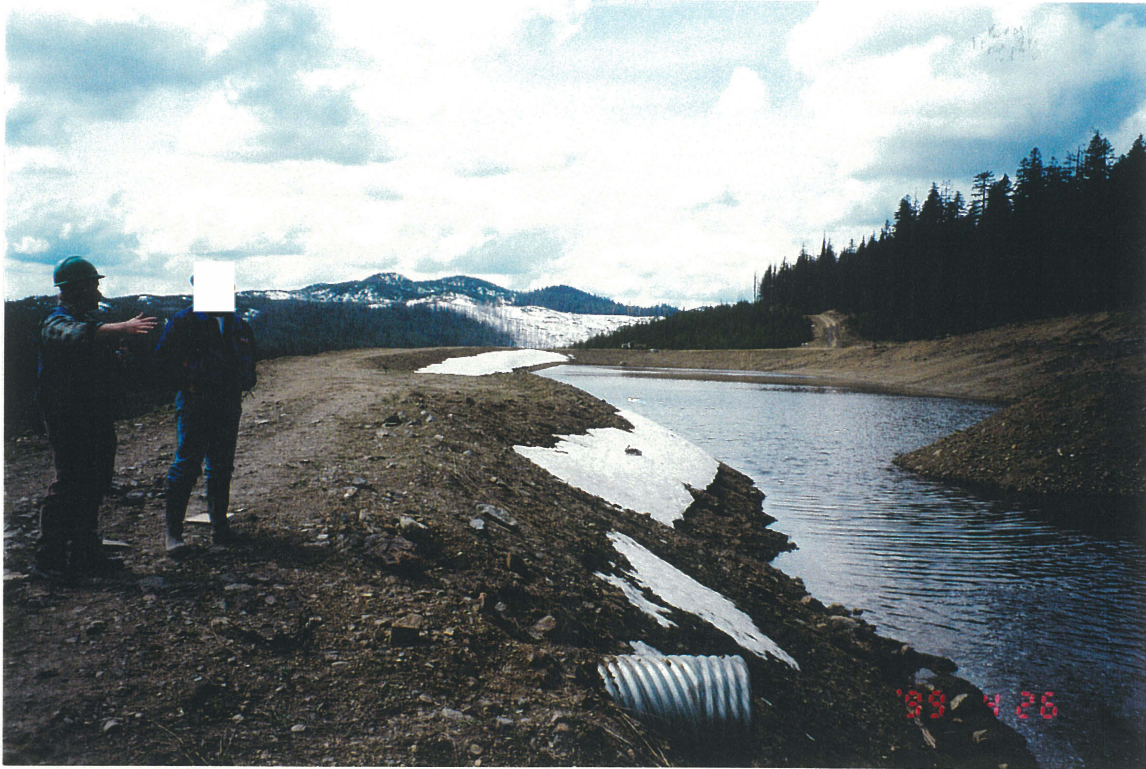
Photo No. 17: Southeast Sediment Pond. Looking west, from end of runoff collection ditch to the manhole sump. Note overflow culvert in foreground.
