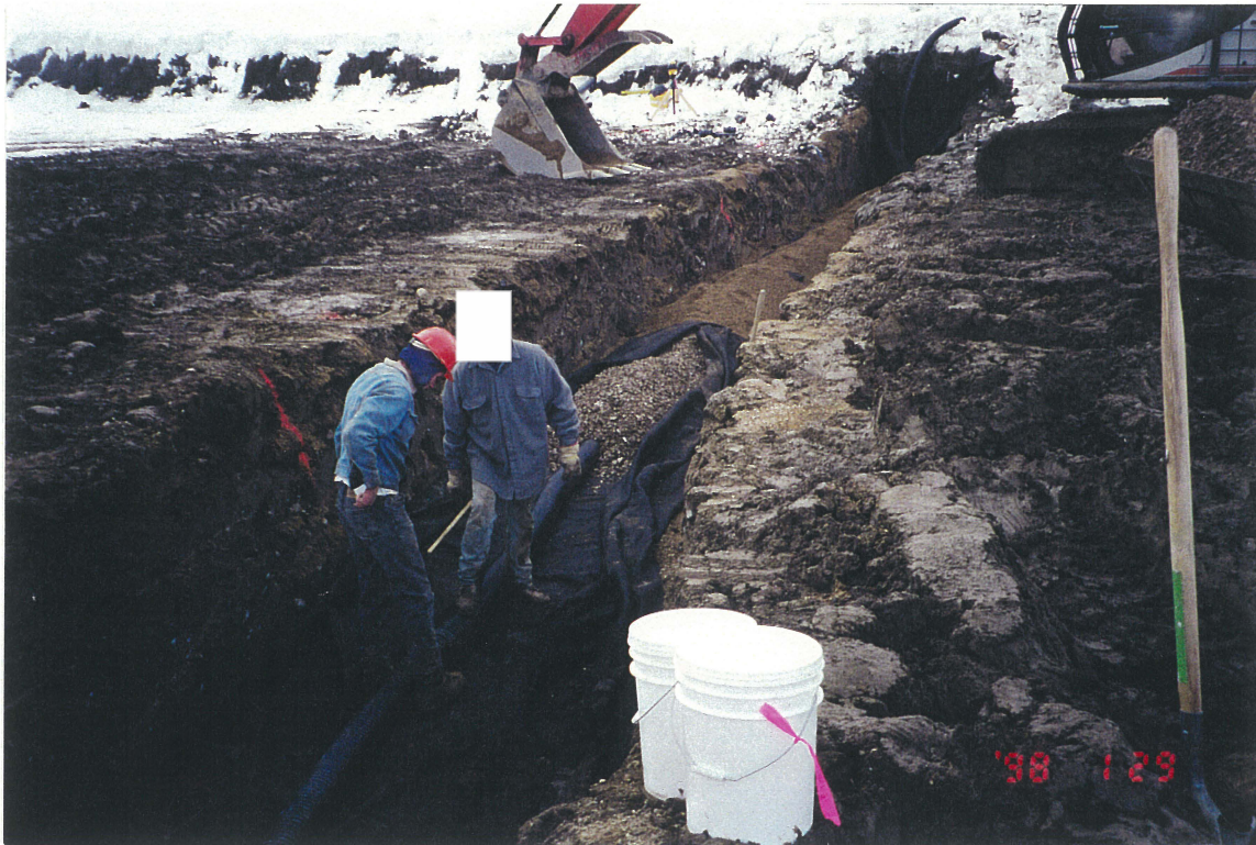
Photo No. 2: Installing Outlet Drain OD-5 at Perimeter Embankment, January 29, 1998.
