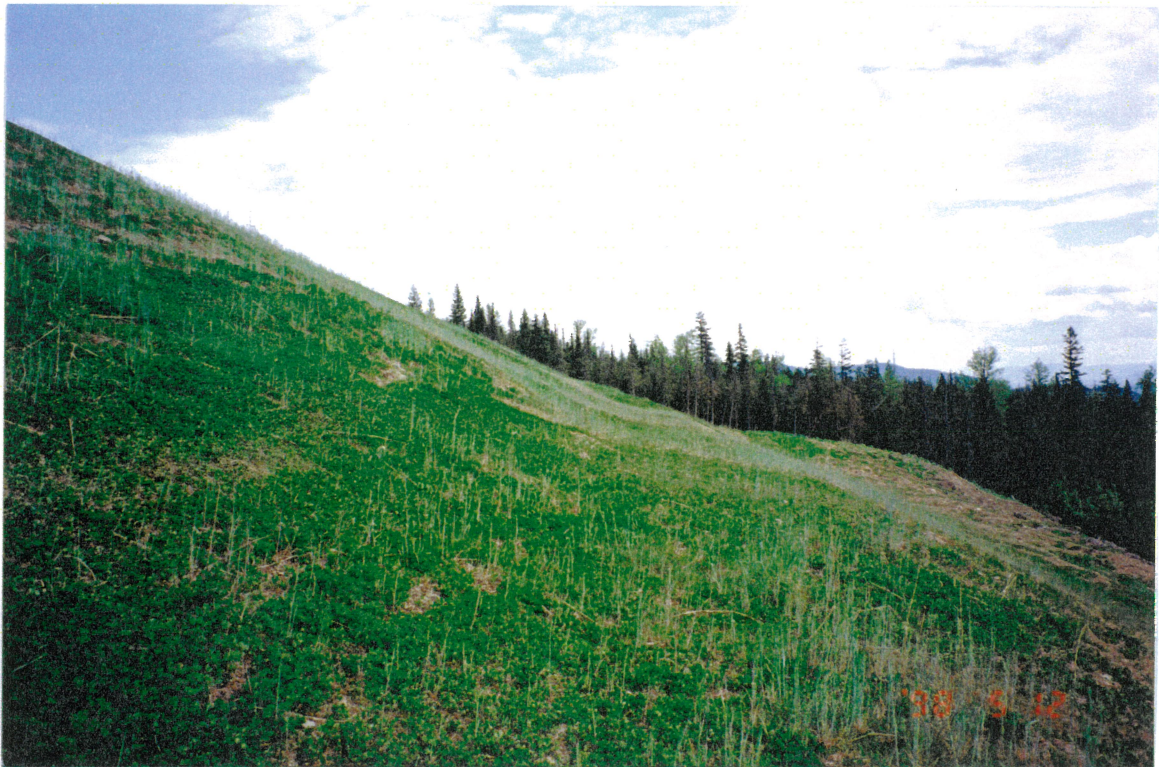
Southeast Sediment Pond. Downstream fill slope looking east. Note dry stable slope and well established re-vegetation.
