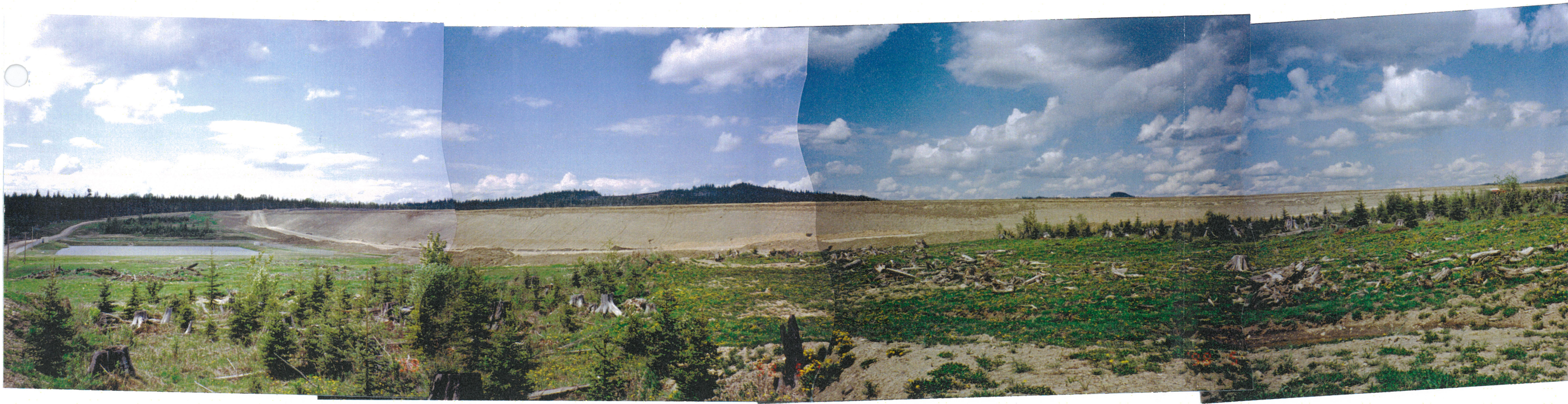
Main Embankment. View looking north, from Bootjack - Morehead Connector Road east of the Seepage Collection Pond. Photo taken near end of construction and only outstanding work is dressing of downstream slope. Note Seepage Collection Pond on left. Zone T material now provides good access to entire Tailings Storage Facility.
