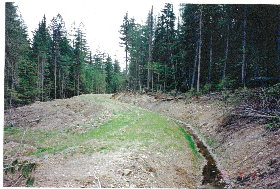
Southeast Sediment Pond - Runoff collection ditch, looking south. Ditch is clear of obstructions.
