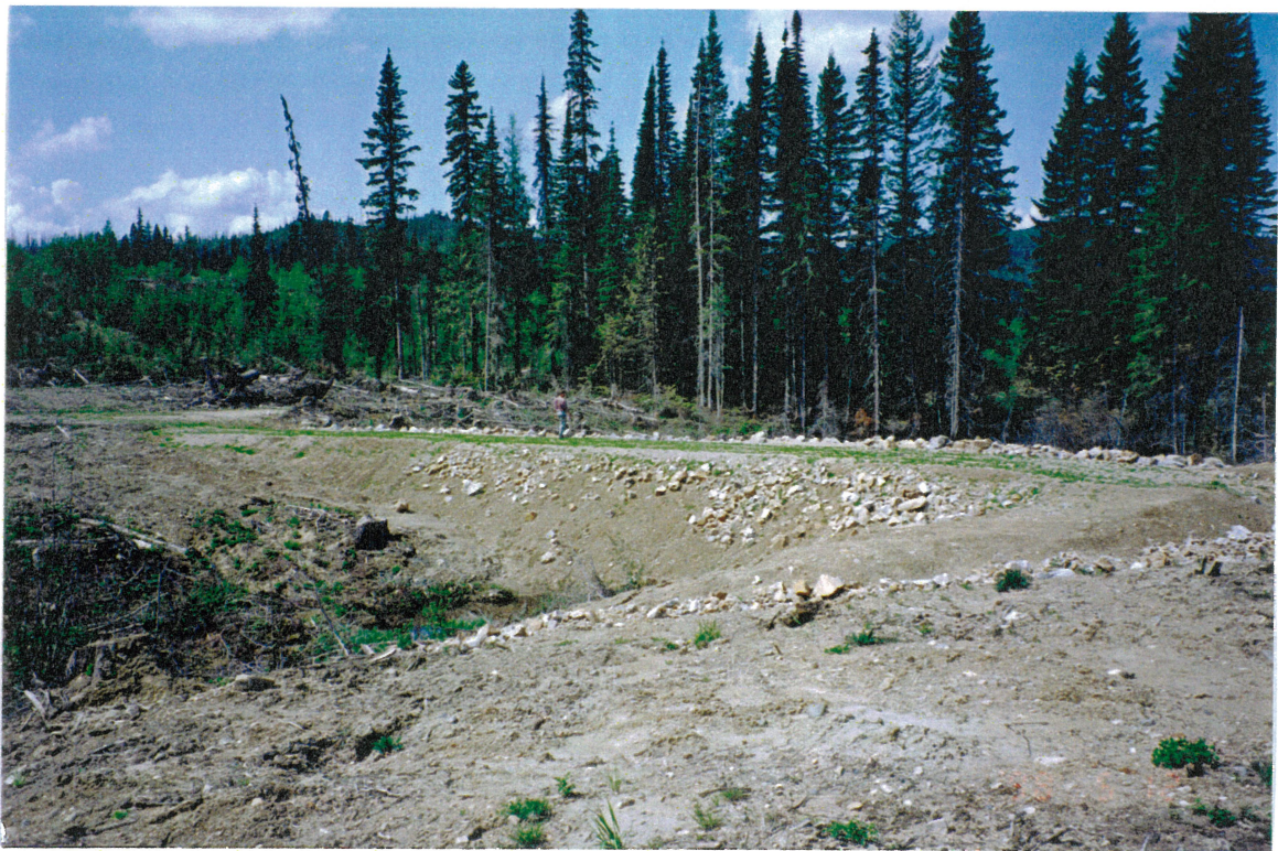
South Bootjack Dam. View of downstream face of embankment, looking northeast. Spillway in foreground is clear of obstructions.
