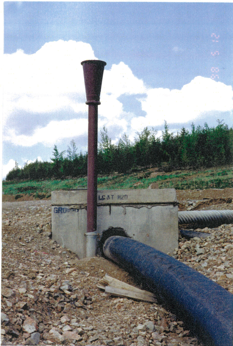
Tailings Pipeline System. Revised T2 Dropbox. Tailings Pipeline now extends all the way from the Mill to the Tailings Storage Facility. T2 Dropbox provides surge protection and is connected to the pipeline by a bifurcation.
