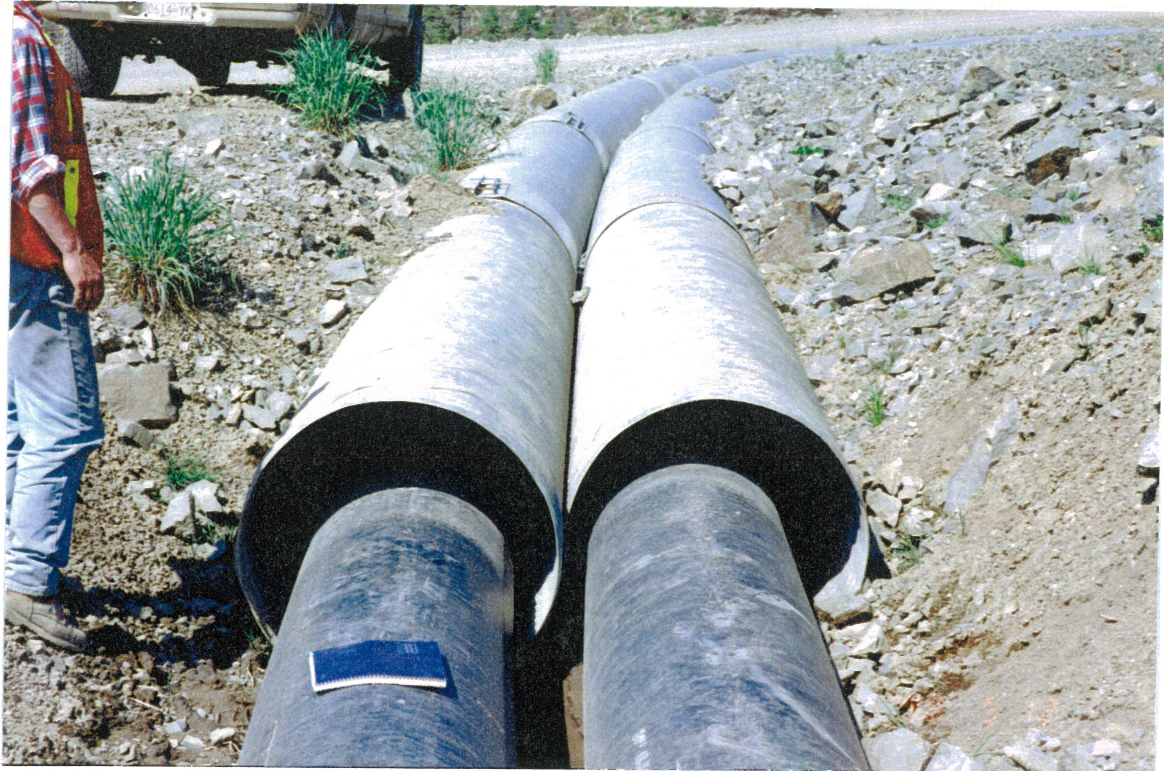
Pipeline Containment Channel. Downstream end of pipeline sleeves at Bootjack Creek Crossing. Note minor amount of tailings at bottom of sleeves.
