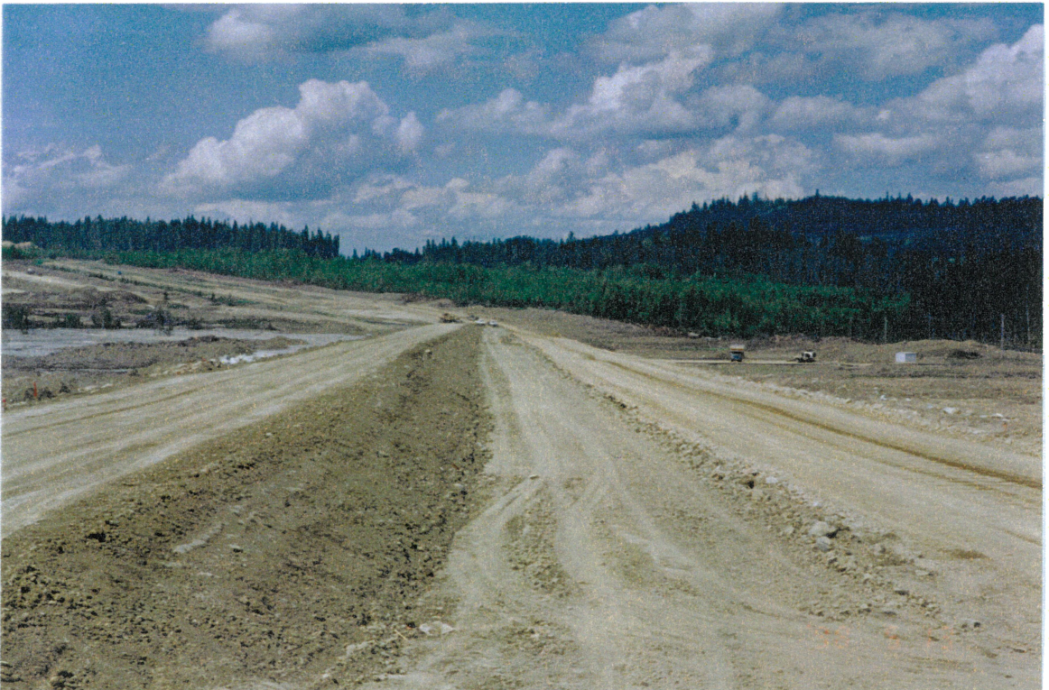
Perimeter Embankment from near right abutment. Note bench left on downstream side for construction of Longitudinal Drain in Stage 2B Construction.
