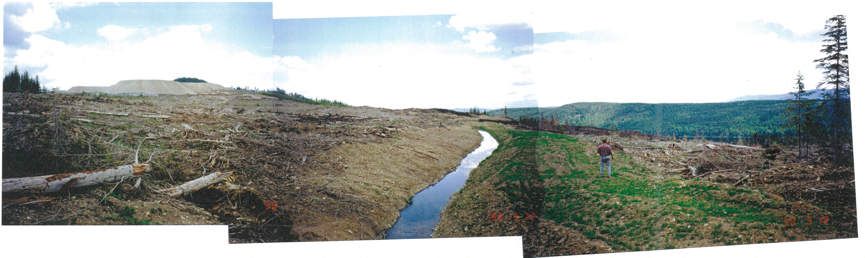
Southeast Sediment Pond - Runoff collection ditch, looking north. Note Mine waste dump to left and Polley Lake to right. Ditch is clear of obstructions.
