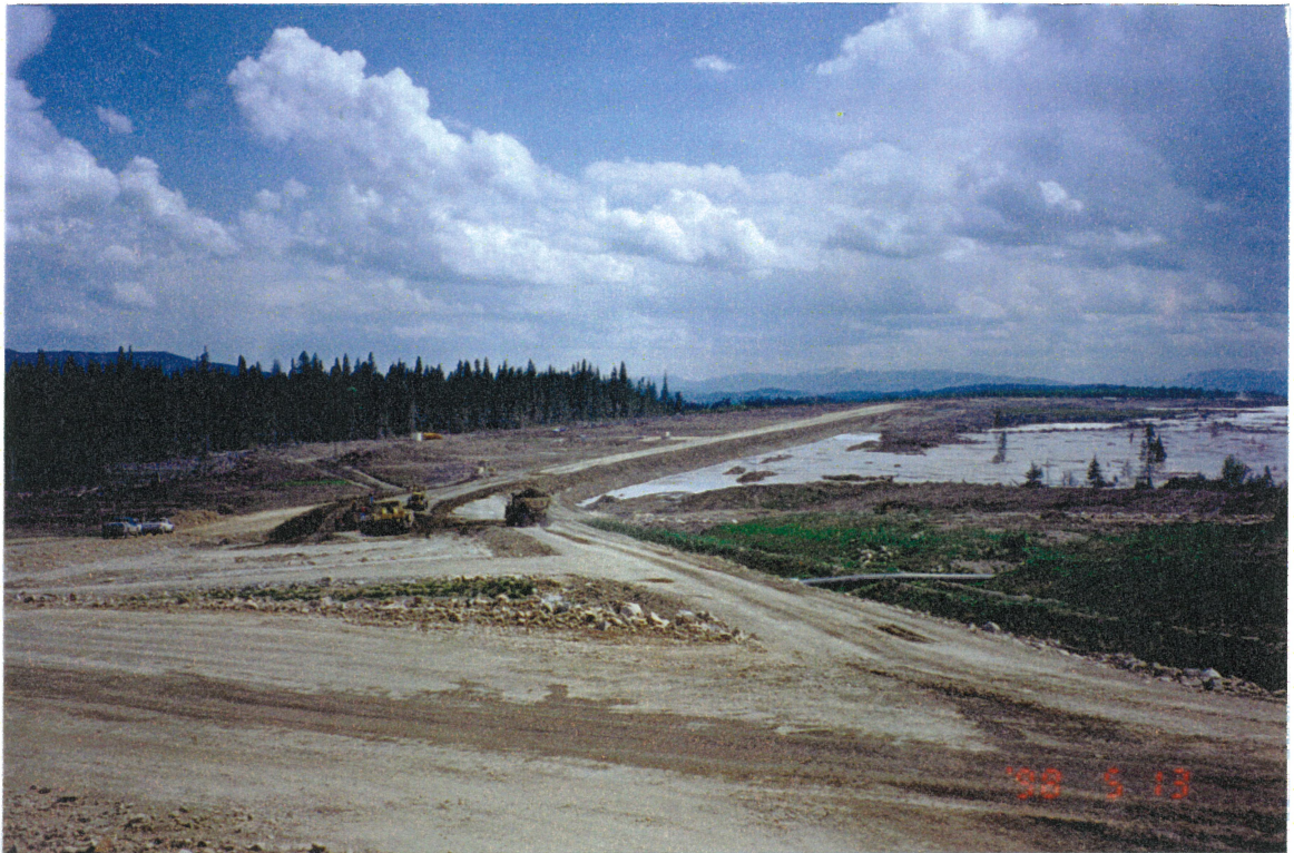
Perimeter Embankment from Left Abutment, end of Stage 2A Construction. Tailings discharge is through M1A dump valve. Note tailings beach development.
