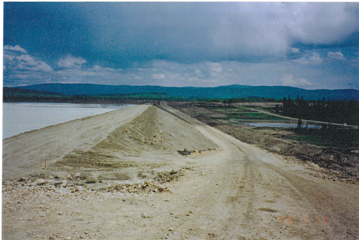
Main Embankment View looking east, from right abutment. Note Zone T material with filter fabric extending up to Stage 2A crest at right abutment.
