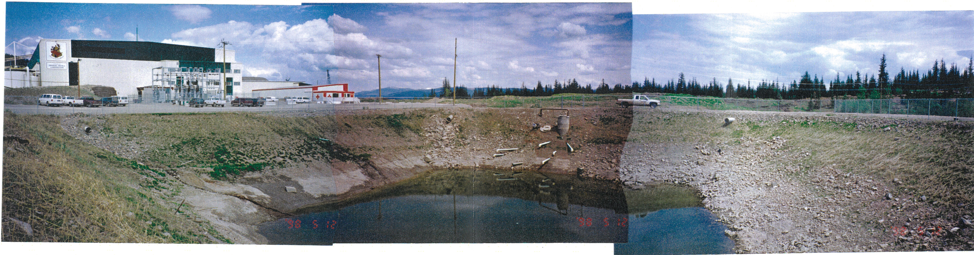
Millsite Sump. Note low water level and stable inner slopes.
