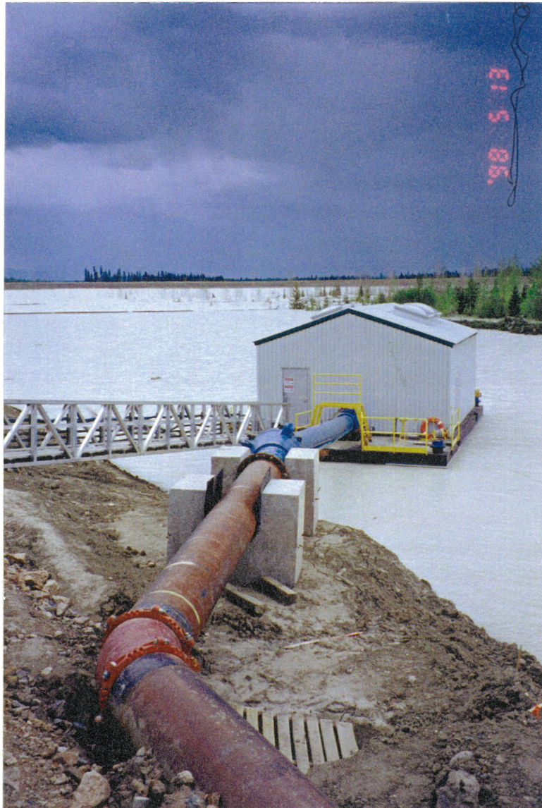
Reclaim Pipeline System. Reclaim Barge and Channel. Note 35 degree elbow added and barge alignment changed.
