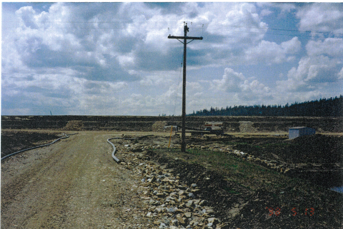
Perimeter Embankment. Looking upstream from access road on east side on Seepage Collection Pond. Note Outlet Drains going up face of embankment.
