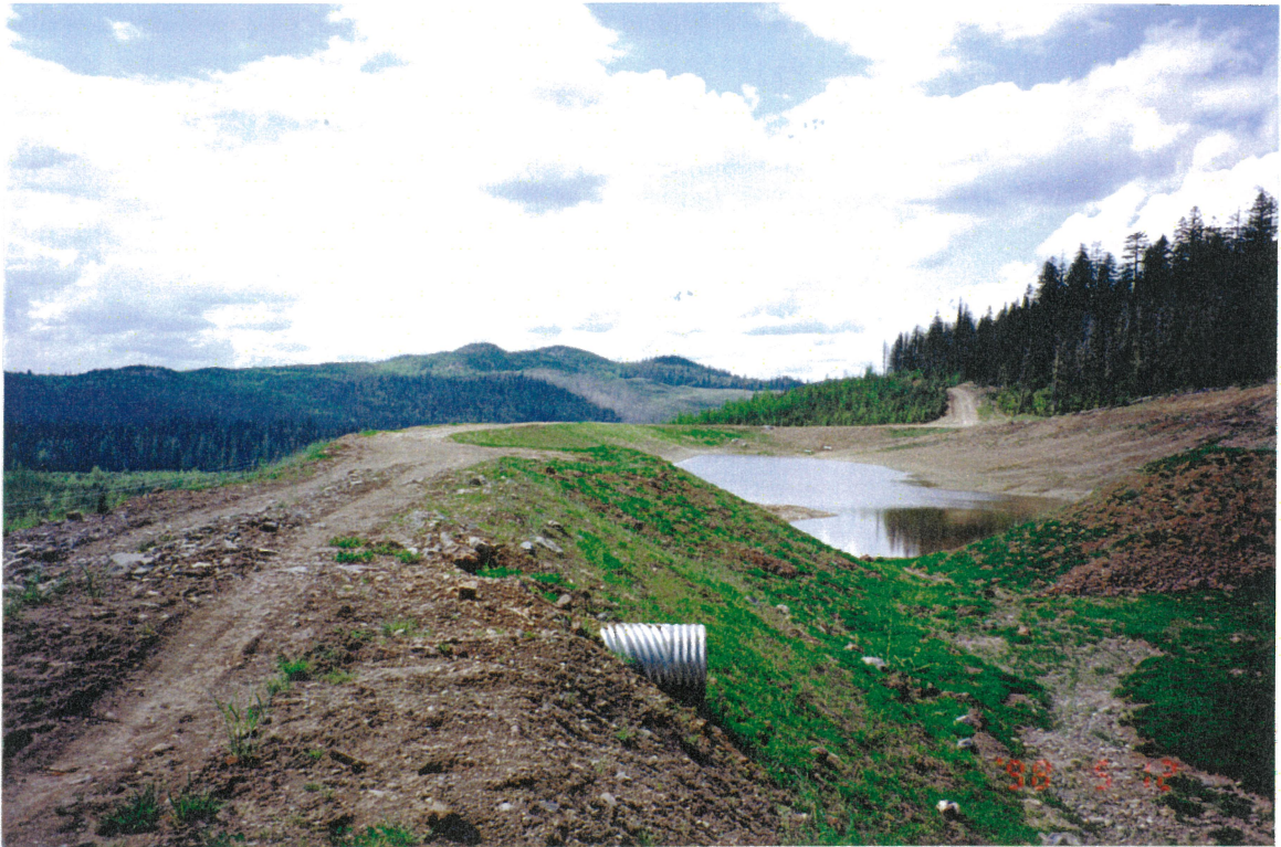
Southeast Sediment Pond. Looking west, from end of runoff collection ditch to the manhole sump. Note low water level and overflow culvert in foreground.
