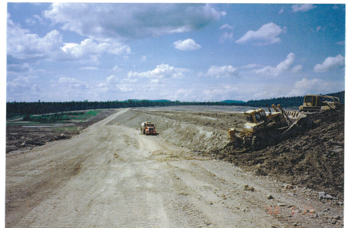
Main Embankment View looking west from left abutment. Final dressing of downstream slope.
