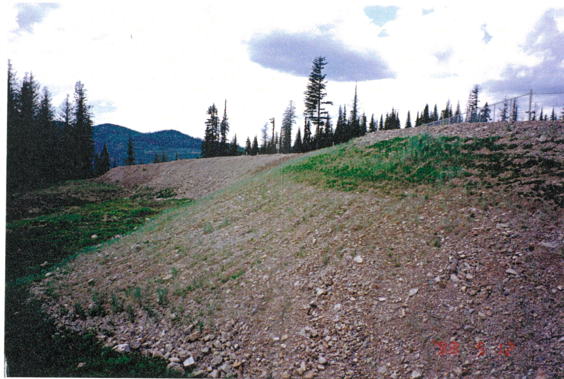
Millsite Sump. View of south slope, looking west. Slope was repaired and is stable. No seepage observed.
