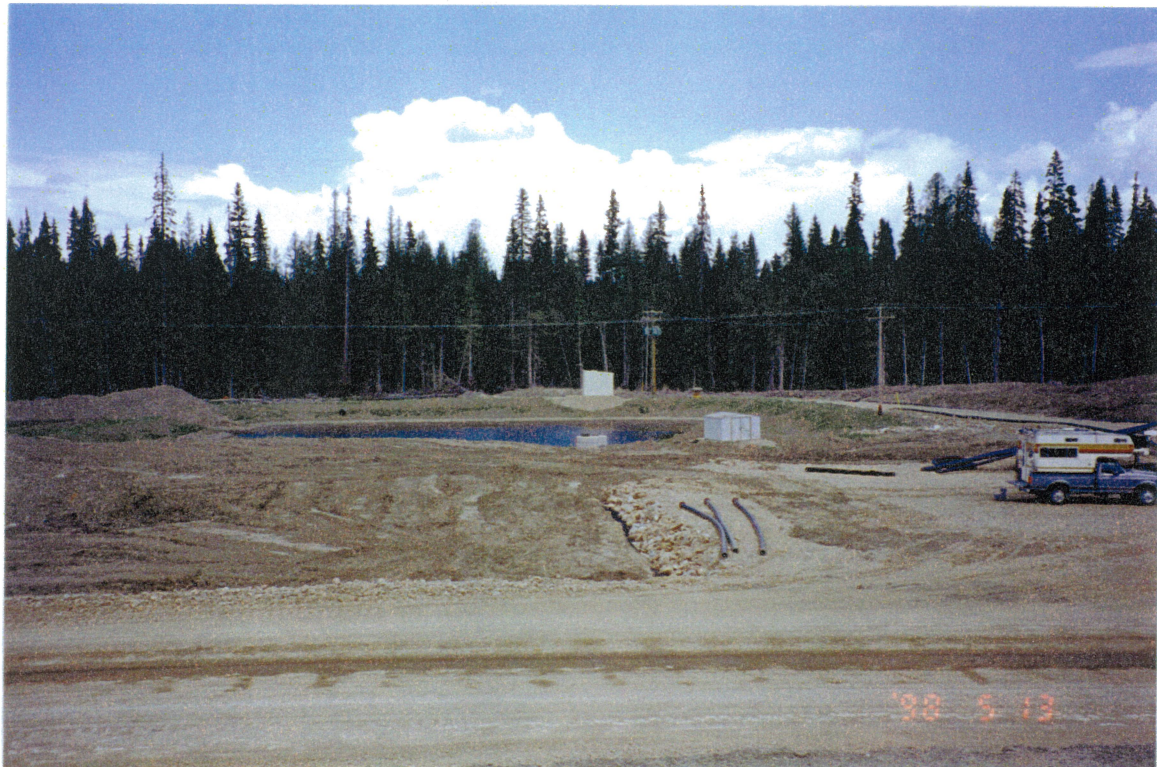
Perimeter Embankment. Looking downstream to Seepage Collection Pond. Note grading of area. Zone T platform was extended to final downstream toe.
