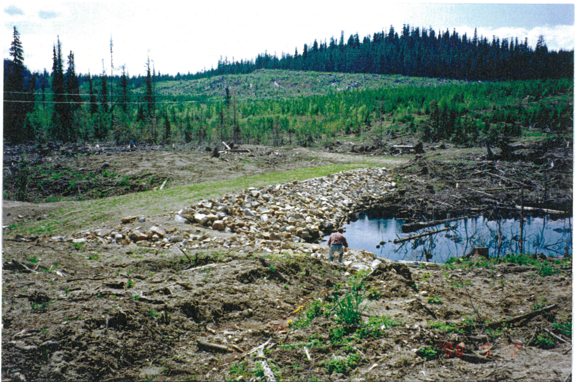
Southeast Bootjack Dam. View of upstream face of embankment, looking southwest. Ponded water is now seeping through old dam back into Bootjack Lake.
