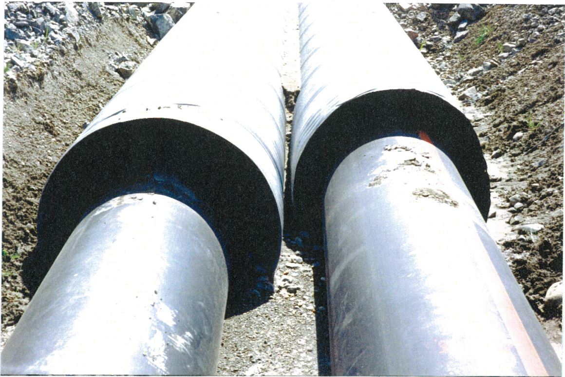
Pipeline Containment Channel. Upstream end of pipeline sleeves at Bootjack Creek Crossing. Note tailings at bottom of sleeves.
