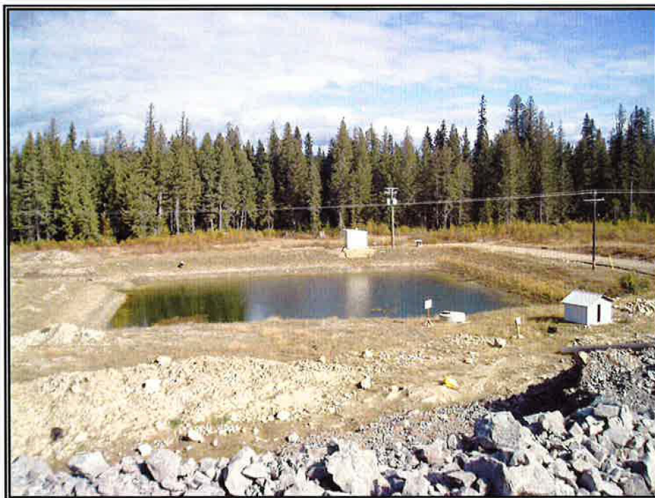
Photo 4: Main Embankment Seepage Collection
