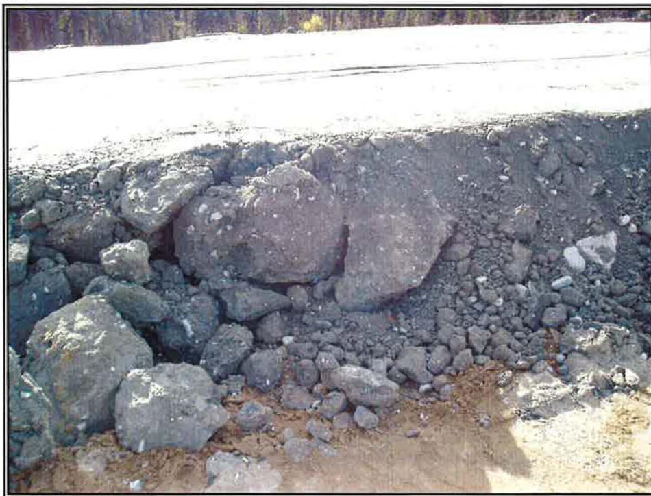
Photo 14: Compacted Till – South Embankment
