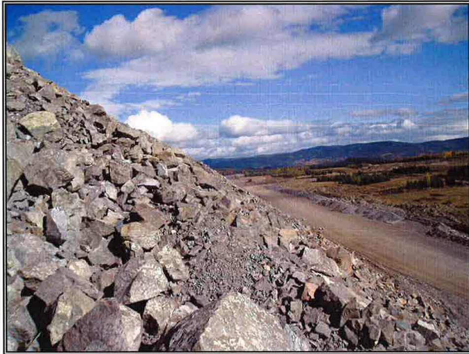
Photo 3: Nature of Main Embankment Rockfill
