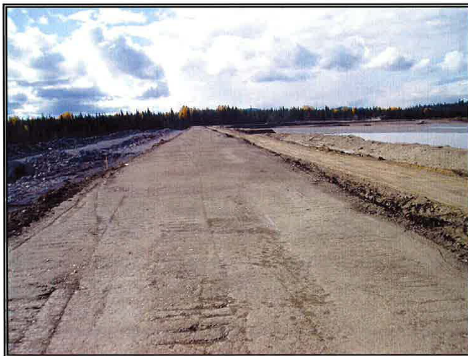
Photo 8: Main Embankment Compacted Core
