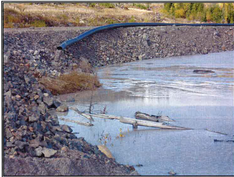
Photo 15: Tailings Overboarding at "Top" of Panel
