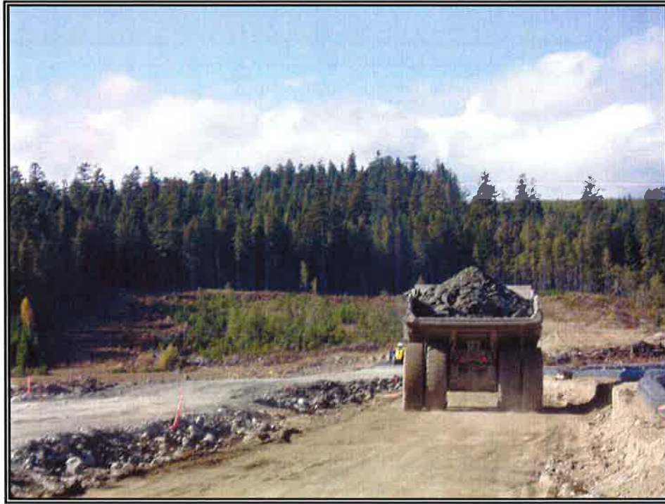
Photo 11: Till Haulage on South Embankment
