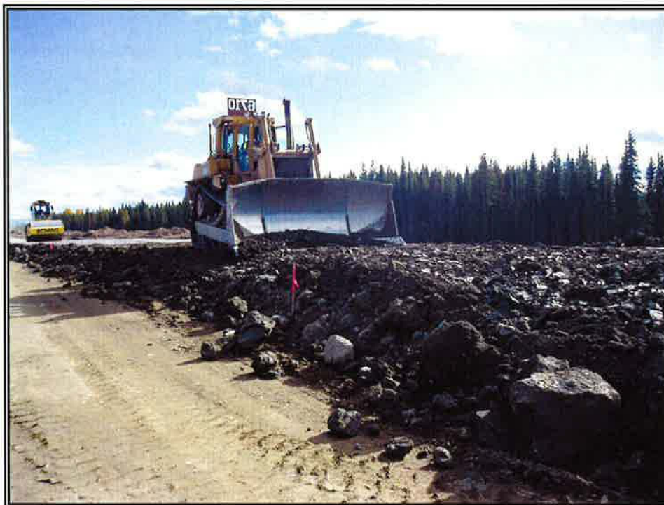
Photo 12: Placement of Till Core – South Embankment
