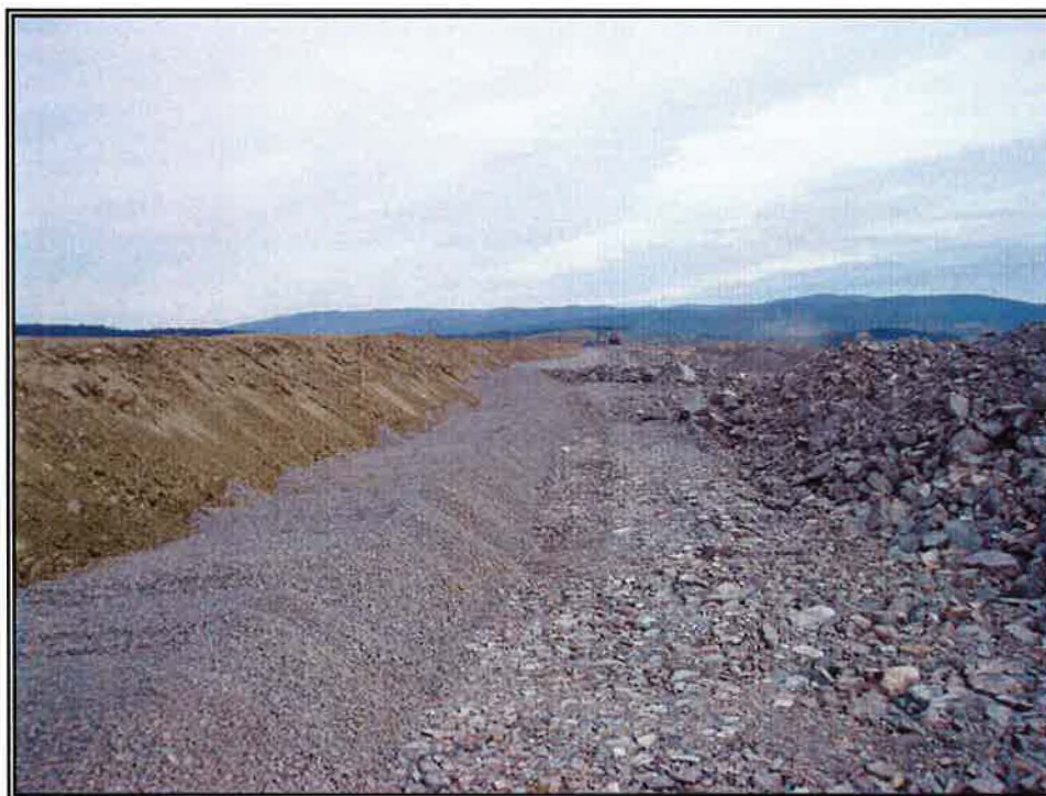
Photo 6: Zones of Main Embankment Dam
