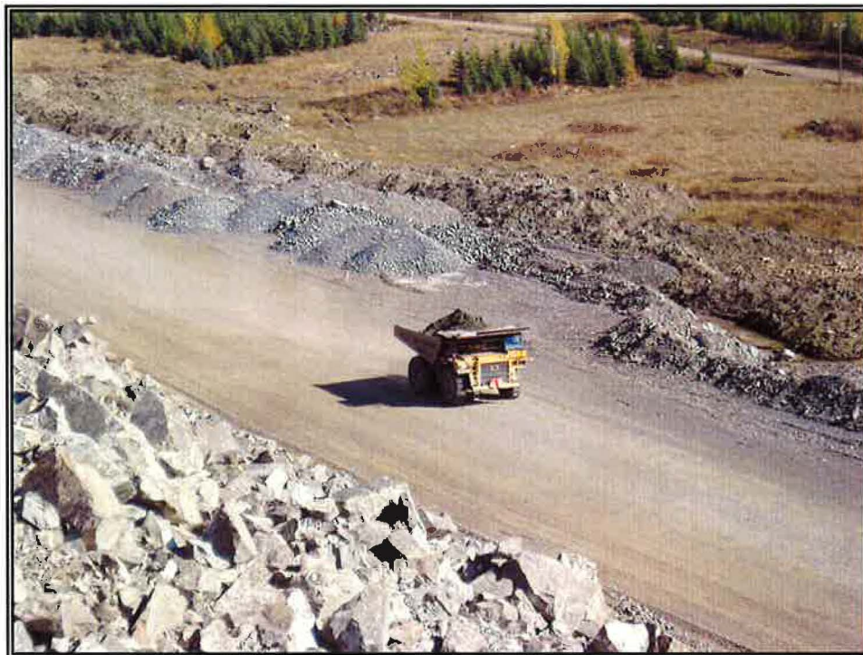
Photo 10: Haulage of Till from Borrow
