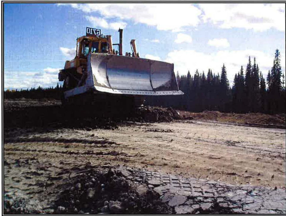
Photo 13: Compacted Till – South Embankment
