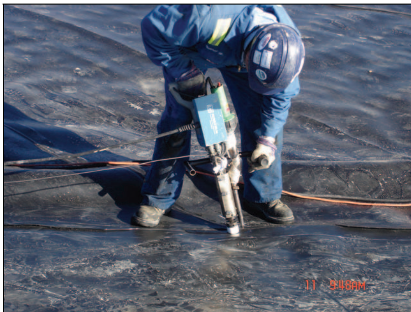
PHOTO 10 – Extruder used to weld two panels together.
