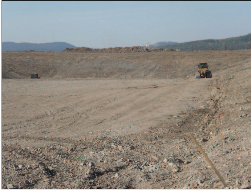
PHOTO 1 – Preparing the open excavation for prepared sub grade
