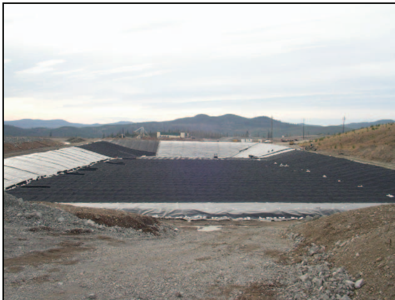
PHOTO 24 – Geonet placed on the floor area.
