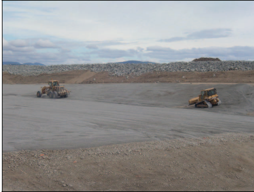
PHOTO 3 – Placement of Zone F – prepared sub grade
