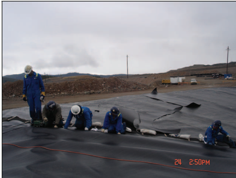
PHOTO 25 – Wedge welding a corner seam.
