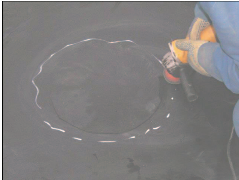
PHOTO 20 – Preparing the surface of a patch for extruder.
