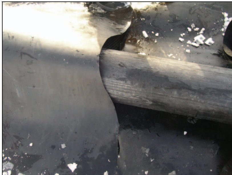
PHOTO 34 – Placement of “skirt” around exit area of the LCRS riser pipe.
