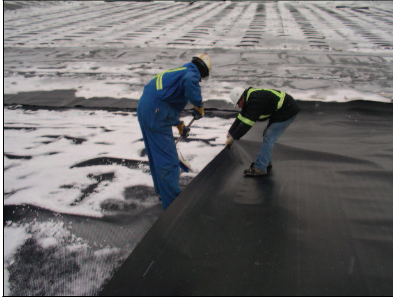
PHOTO 29 – Snow and ice removal from Geonet
