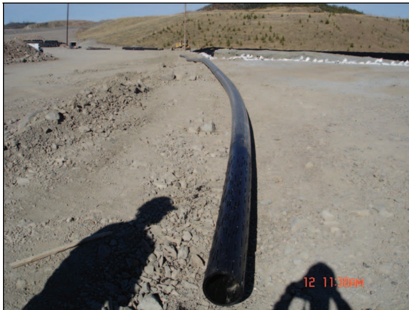
PHOTO 16 – Slotted 200 mm PVC riser pipe
