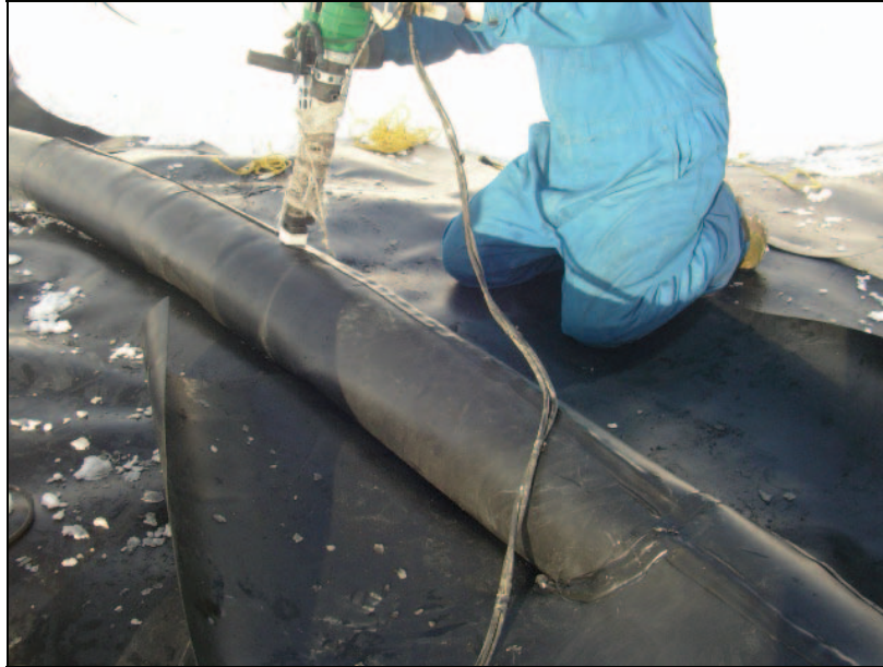
PHOTO 35 – Extruding the LCRS riser pipe “skirt”
