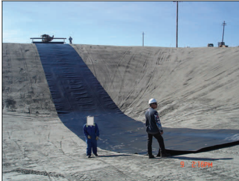
PHOTO 7 – First panel of HDPE liner placed in sump area
