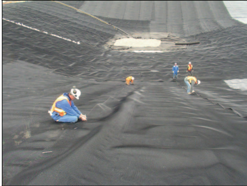
PHOTO 21 – Ties used to hold the Geonet together
