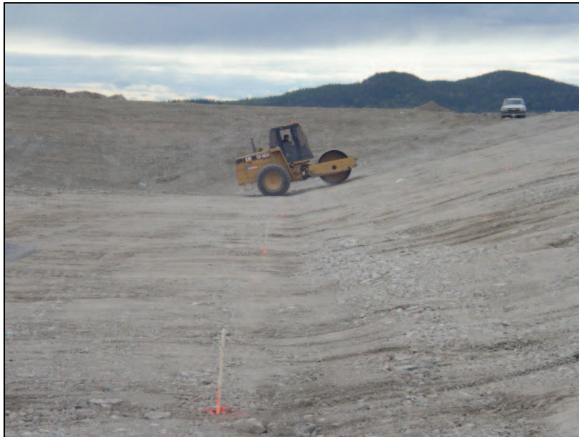
PHOTO 2 – Compacted open excavation
