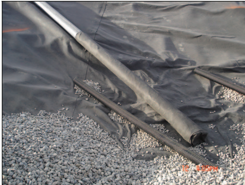
PHOTO 17 – Geotextile wrapped around the end of 200 mm PVC riser pipe.
