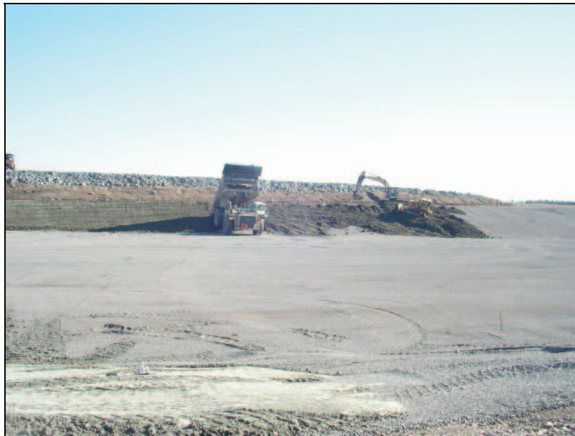
PHOTO 4 – Placement of Zone S on the side slopes
