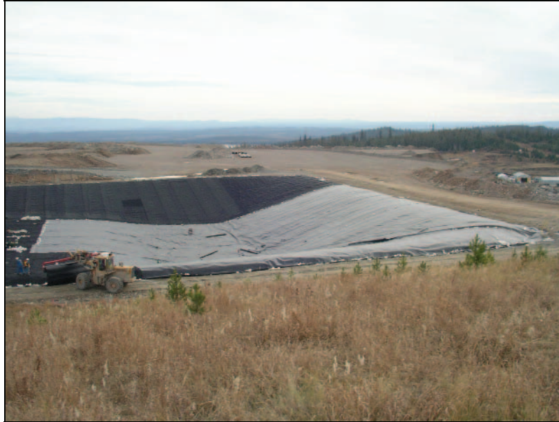
PHOTO 23 – Placement of the second HDPE liner in the sump area.
