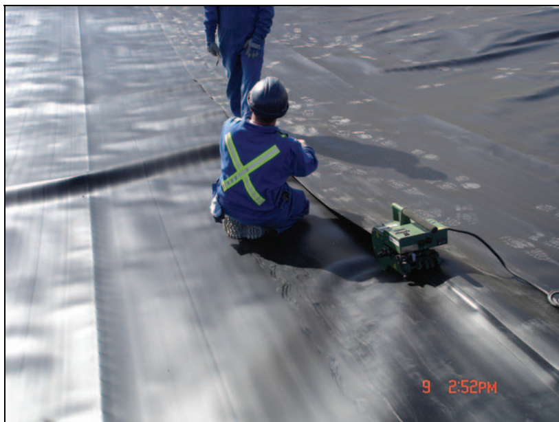
PHOTO 8 – Wedge welding two panels together
