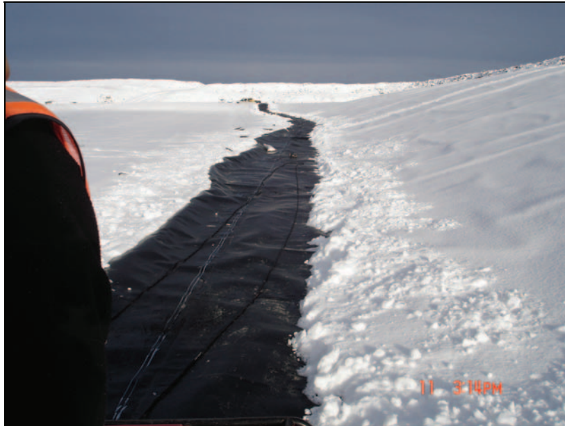
PHOTO 33 – Snow removal to finish welding the tie in seam
