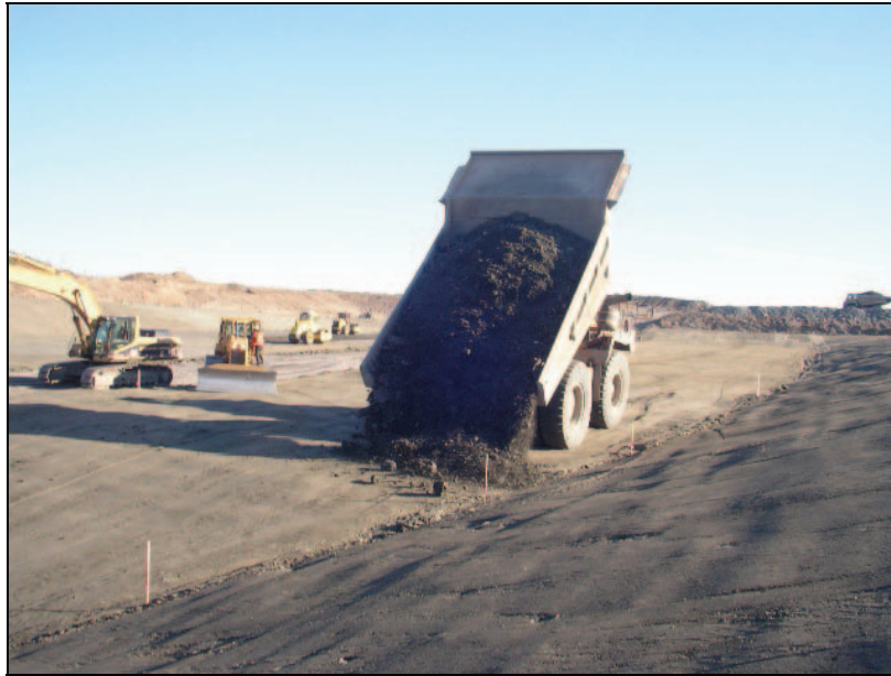
PHOTO 5 – Placement of second layer of Zone S
