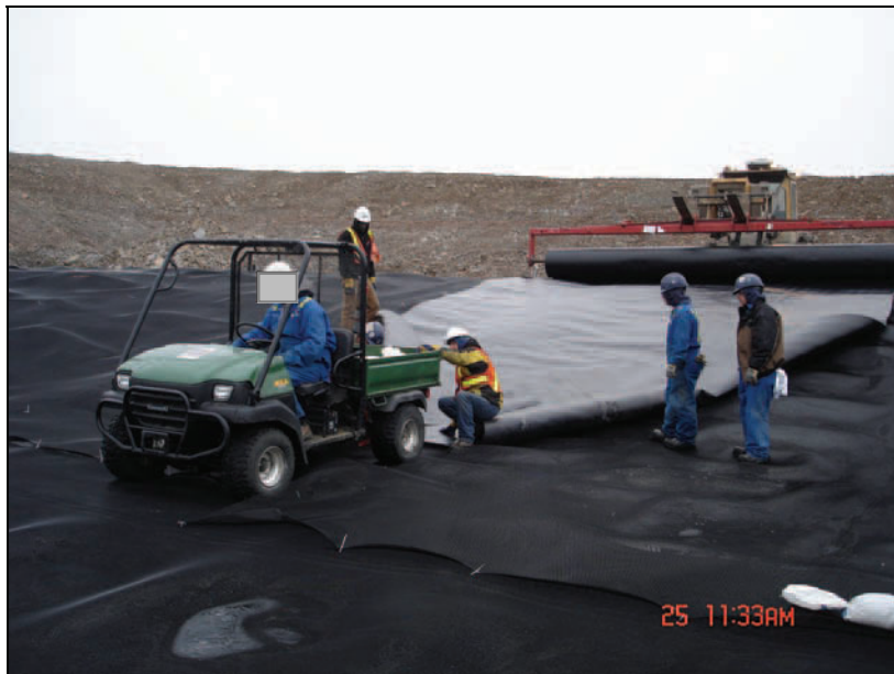
PHOTO 26 – Mule used to pull panels along the floor area.
