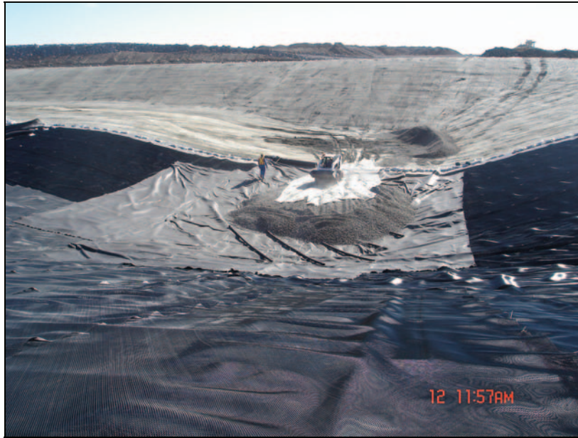
PHOTO 15 – Placement of geotextile, CPT pipe, and LCRS drain rock
