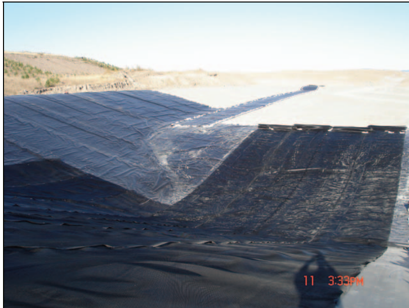
PHOTO 14 – Geonet placed in the sump area
