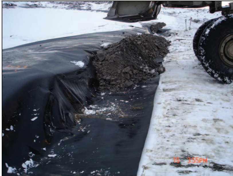
PHOTO 37 – Placement excavated trench material back into the trench.
