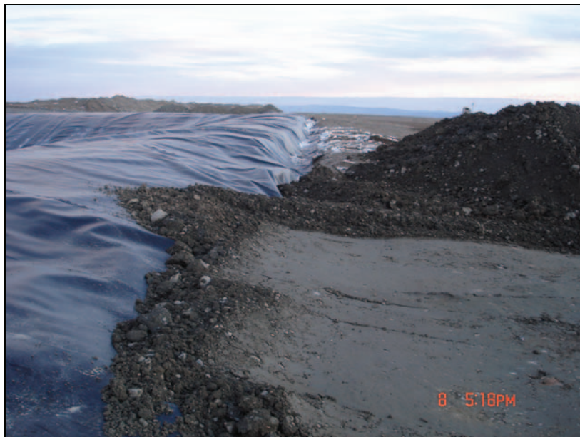
PHOTO 38 – Placement of Zone S material into the trench.
