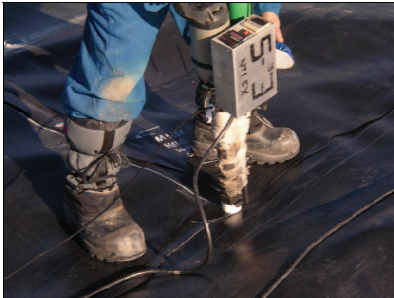
PHOTO 30 – Extruding a tie in seam.
