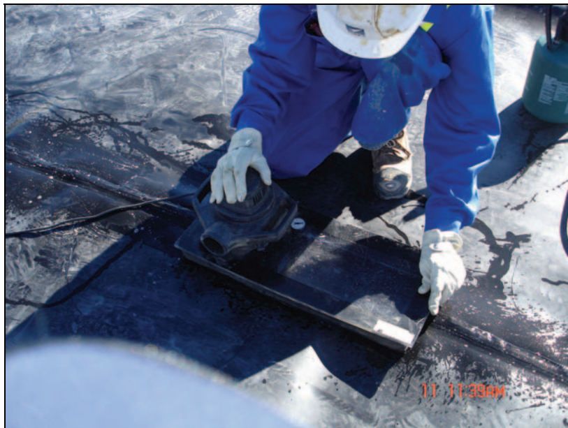
PHOTO 12 – Vacuum test on extruded seam
