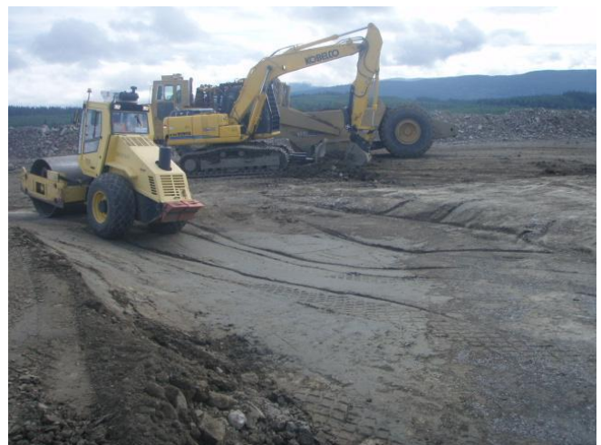
**Excavated then packed area on corner 2
