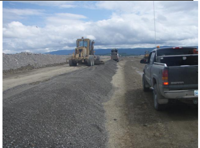
Laying filter around 18+00
