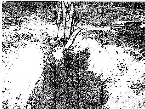
Photo 1: Test pit conducted in existing diversion trench near the south abutment.
