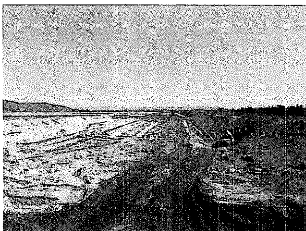
Photo 14: Looking southeast at the sand cell construction on the South embankment.
