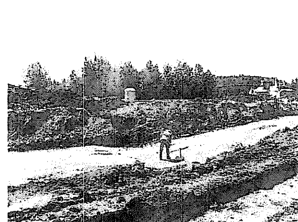
Photo 6: Native till density testing at Perimeter abutment.
