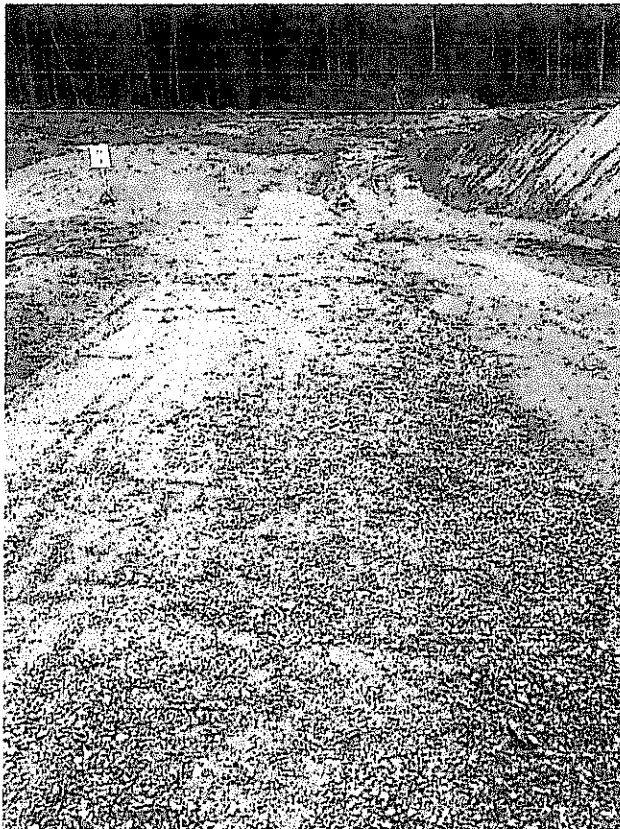
Figure(s) 3: The blue marker indicates where the T/F contact is supposed to be at the given elevation. As we approach 4-corner, material must be added - whereas material must be removed as we distance ourselves from 4-corner.
