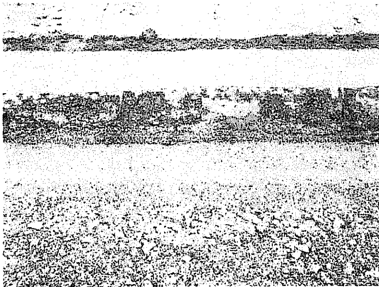
Figure 1: Shallow slope of till resulted in a slight over-lap of the filter layer
