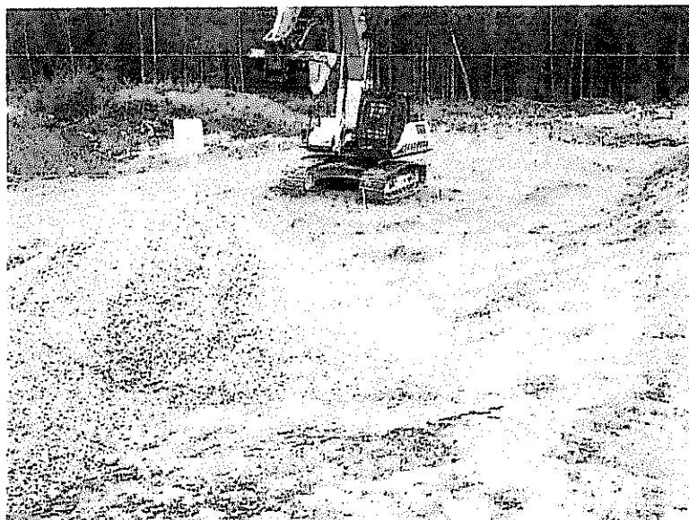
Figure 2: Placement of filter by 4-corner within the outlined bounds
