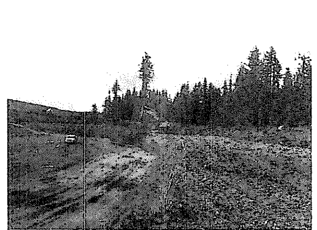
Photo 21: Borrow pit development along the north pit extents.
