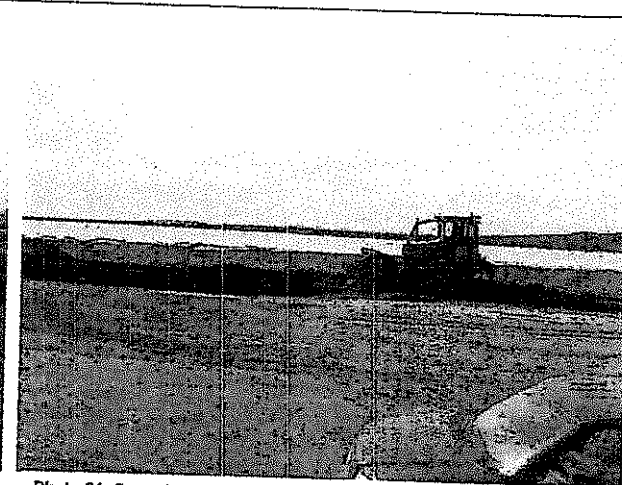
Photo 21: Spreading Zone S material along the perimeter embankment.
