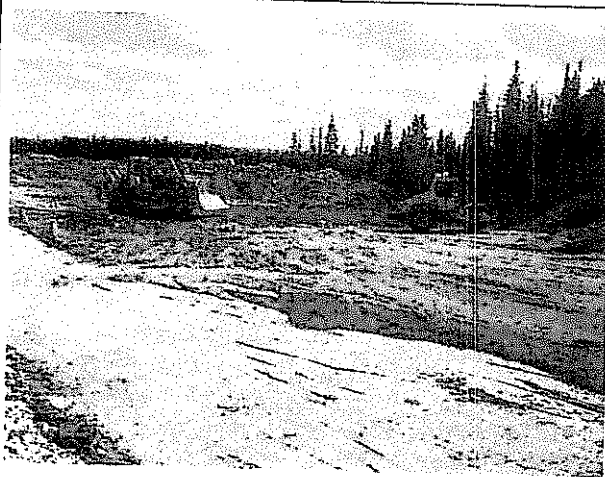
Photo 7: Placement of drainage blanket at the south embankment
