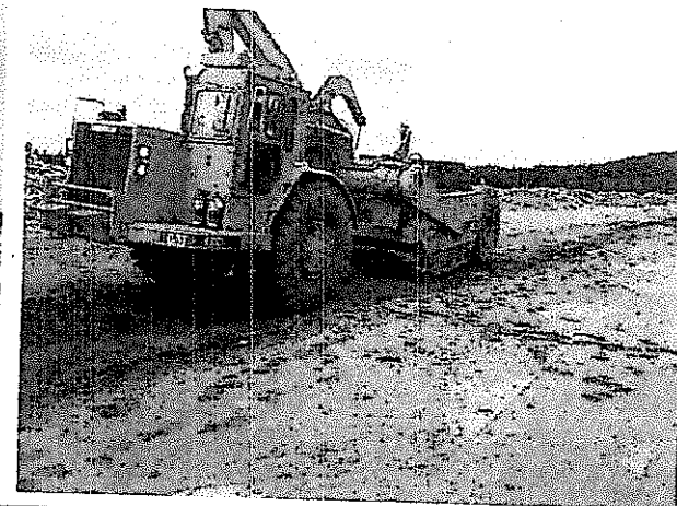
Photo 24: Removing trimmed Zone S material.
