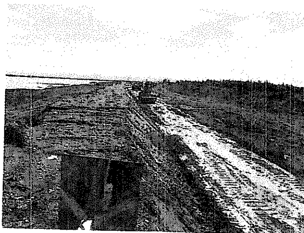
Photo 5: Proof rolling, compacting the exposed core for Zone S placement.
