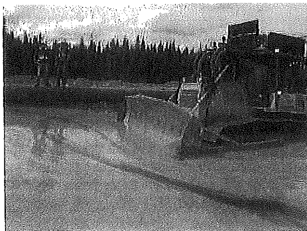
Photo 9 – Cell construction – slimes
