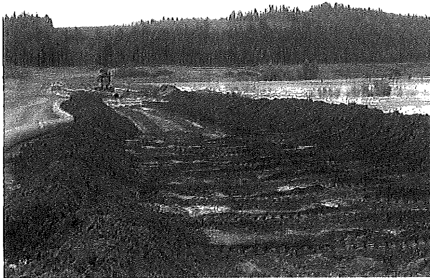
Photo 15 – Bottom of newly prepared cell partially smoothed
