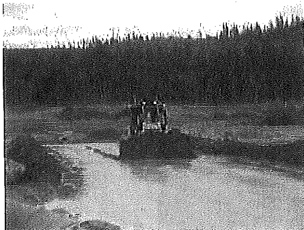
Photo 8 – Cell construction – pushing sand downstream
