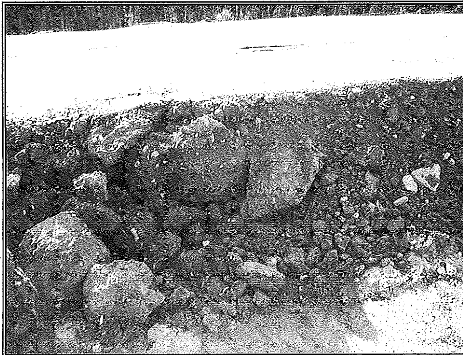
Photo 14: Compacted Till – South Embankment
