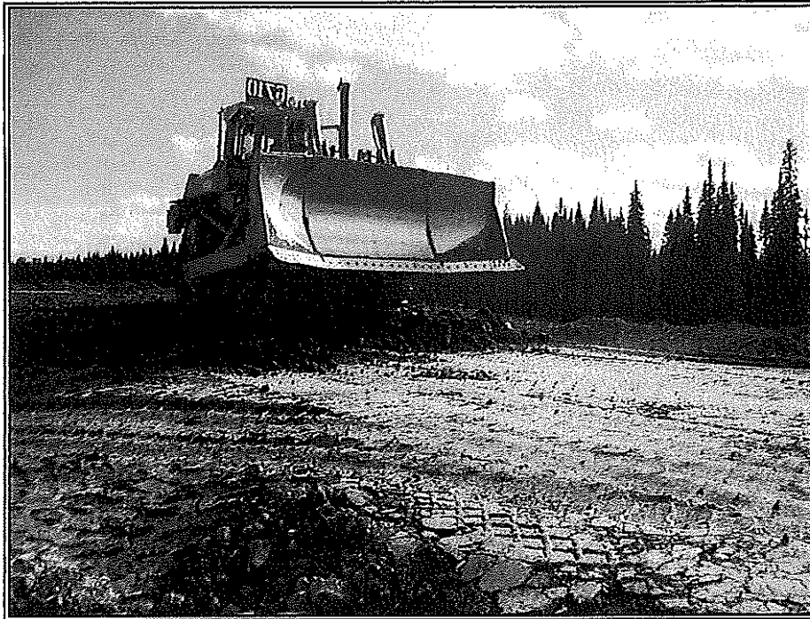
Photo 13: Compacted Till – South Embankment
