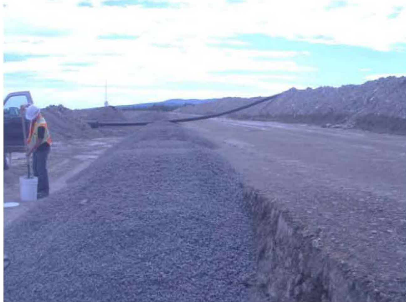
Figure 1: Filter placed near to the ME pipe.
