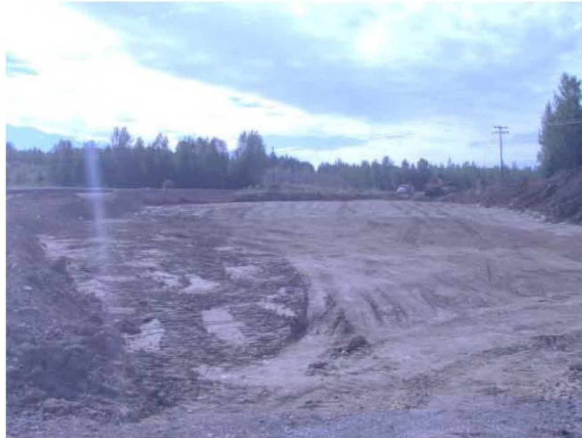
Figure 3: Tie-in preparations by corner-5.
