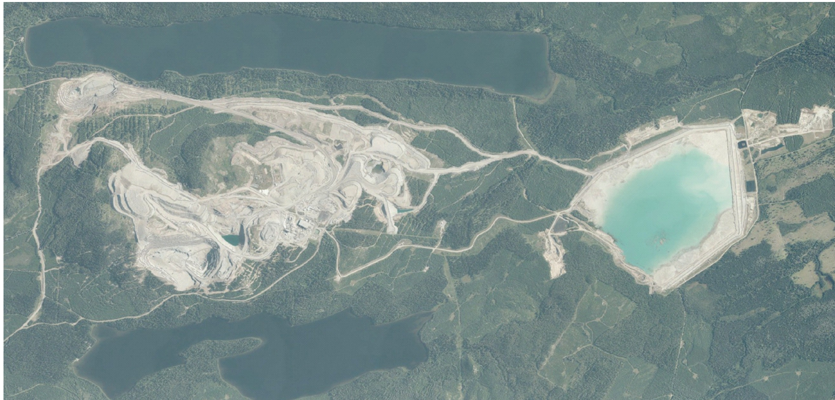
Figure 1.1: Aerial View of Mount Polley Mine Site: 2012
