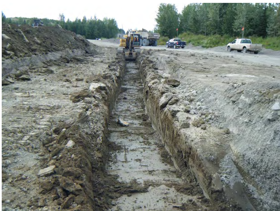
Photo 3: Filter trench excavated along the perimeter abutment to tie into the existing trench.
