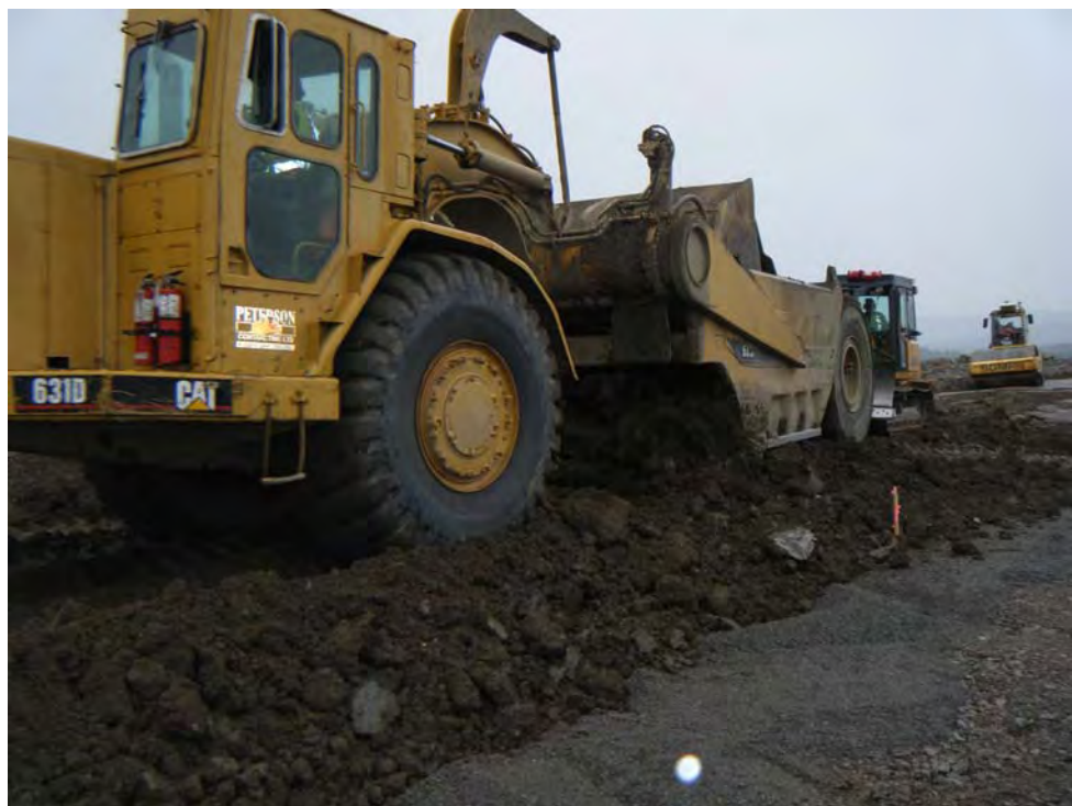
Photo 20: Placement of Zone S on the south embankment.
