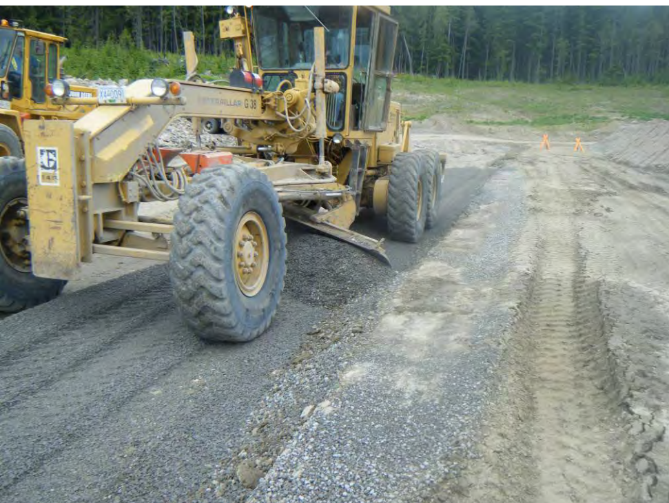
Photo 27: Shaping of Zone F material along the south embankment.
