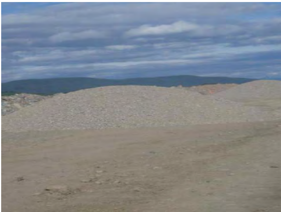
Photo 31: Crushed Zone T material stock pile. This material was utilized for the majority of Zone T placement for the 2011 construction.
