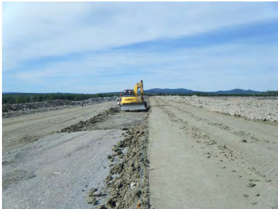
Photo 23: Shaping downstream toe of Zone S along the main embankment, and exposing previously placed Zone F.
