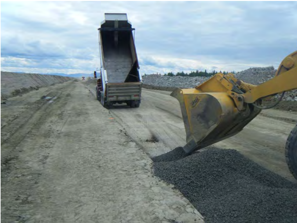
Photo 26: Placement of Zone F material along the south embankment.
