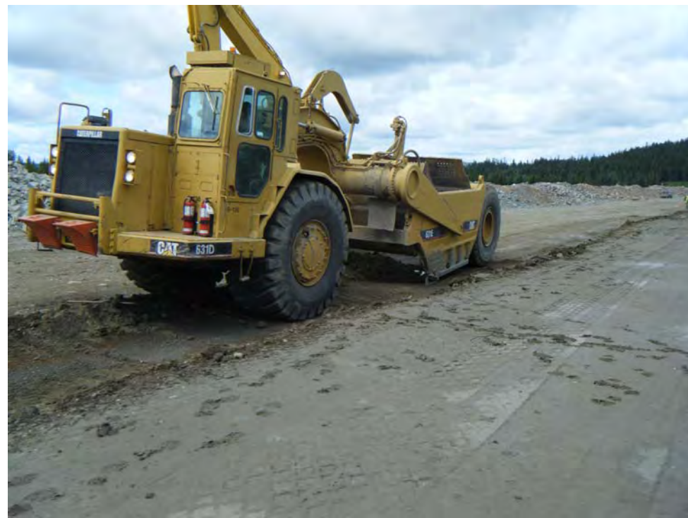
Photo 24: Removing trimmed Zone S material.
