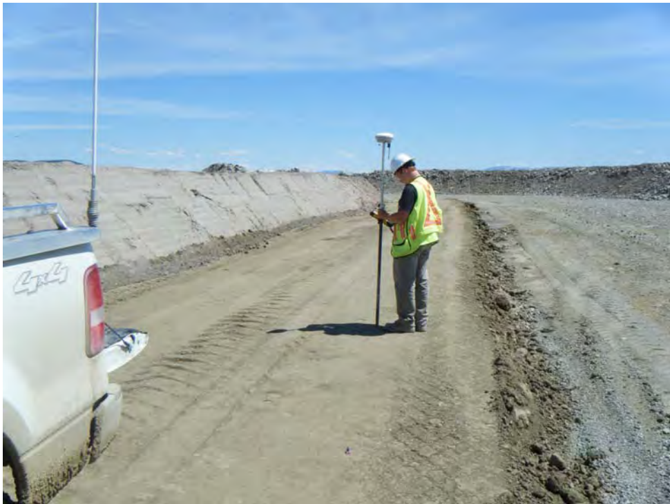
Photo 34: Surveying of compaction test location.
