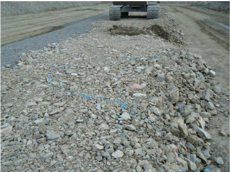
Photo 29: Poorly sorted Zone T material, with areas identified to be removed (south embankment).
