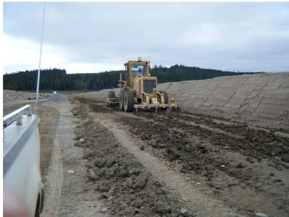
Photo 19: Looking west along the south embankment during scarification of previously placed Zone S material.
