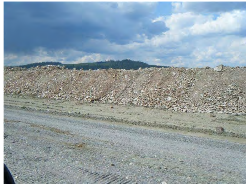
Photo 12: Zone U comprised of NAG rockfill along the Main Embankment.
