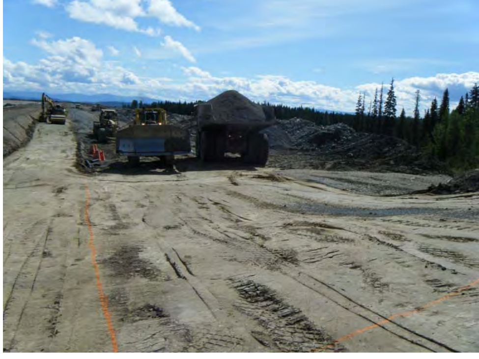
Photo 6: Compacted and proof rolled abutment detail at the south abutment.
