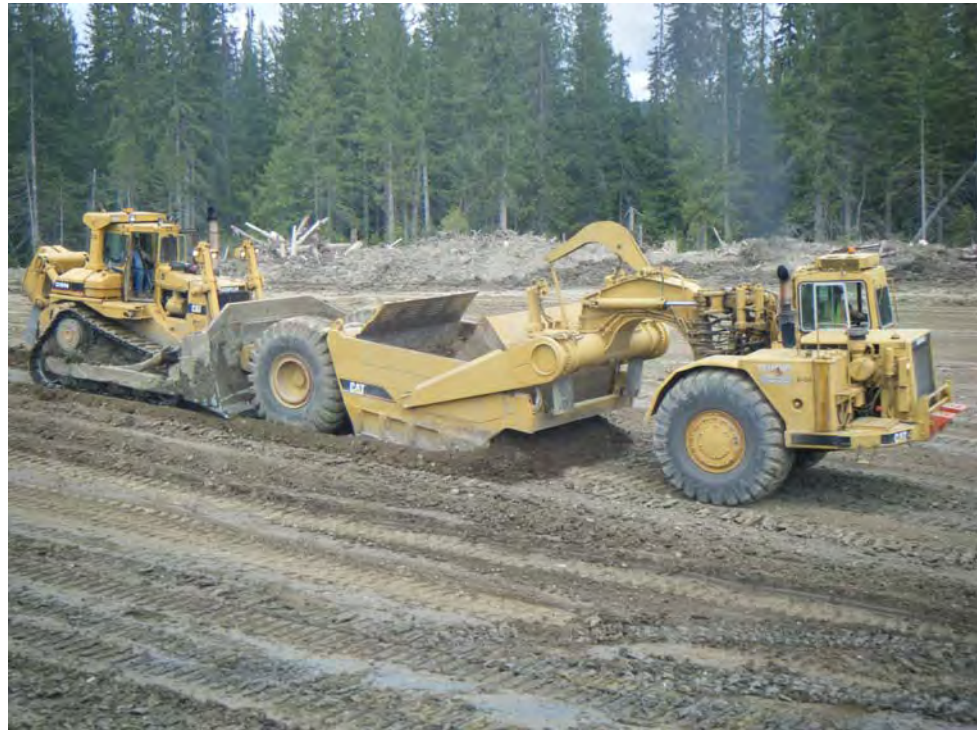
Photo 25: Loading of Zone S material at the perimeter borrow pit.
