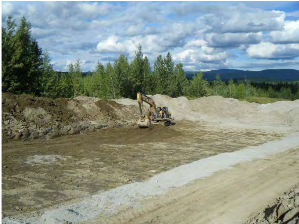
Photo 9: Removing previously placed material at the perimeter embankment to expose competent native till.
