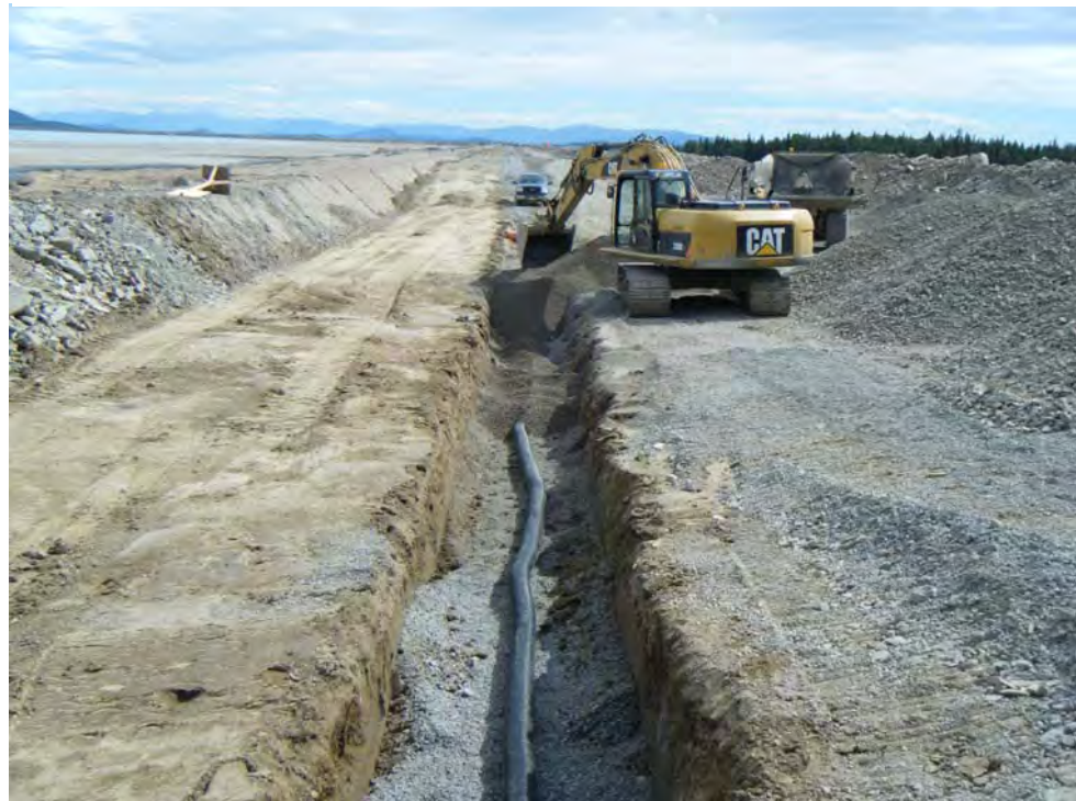
Photo 4: Filter Trench being backfilled along the south embankment. Note the corrugated pipe placed to tie into existing drainage channel
