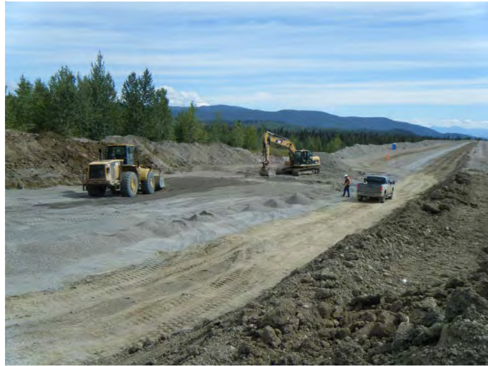
Photo 11: Placement of drainage blanket at the perimeter abutment.
