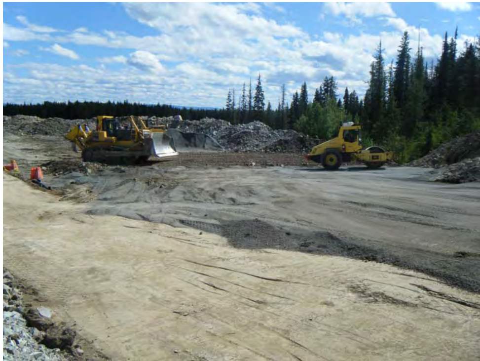
Photo 7: Placement of drainage blanket at the south embankment
