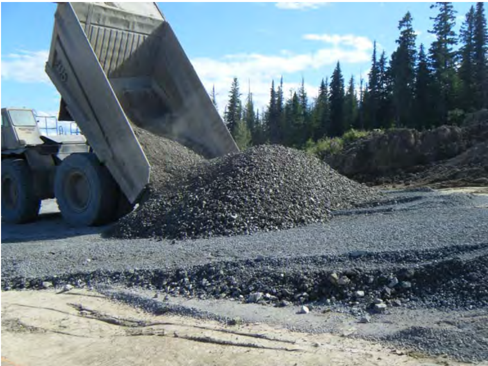
Photo 8: Placement of Zone T material over the drainage blanket at the south abutment.
