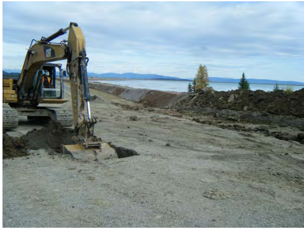
Photo 2: Test pit conducted at the perimeter abutment.
