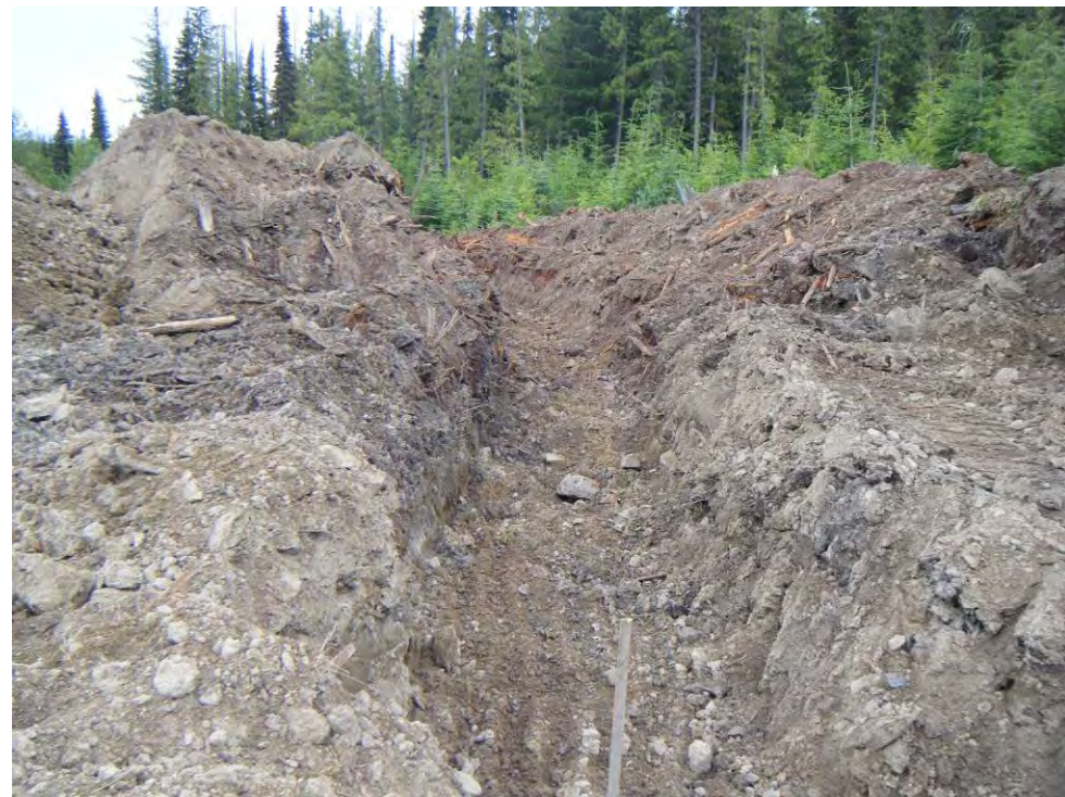
Photo 1: Relocation of the diversion trench near corner 4.
