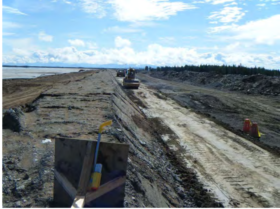
Photo 5: Proof rolling, compacting the exposed core for Zone S placement.
