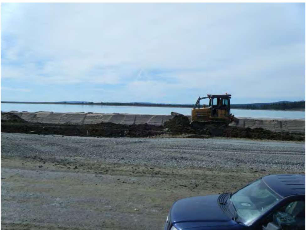
Photo 21: Spreading Zone S material along the perimeter embankment.
