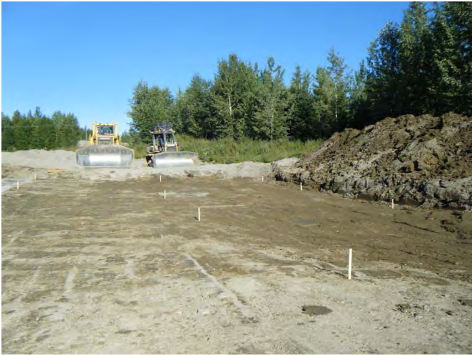
Photo 10: Survey stakes delineating drainage blanket placement area at the perimeter abutment.
