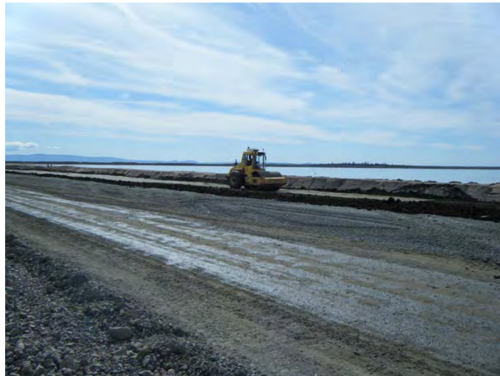
Photo 22: Compaction of Zone S along the perimeter embankment with a 10 ton smooth drum vibratory compactor.
