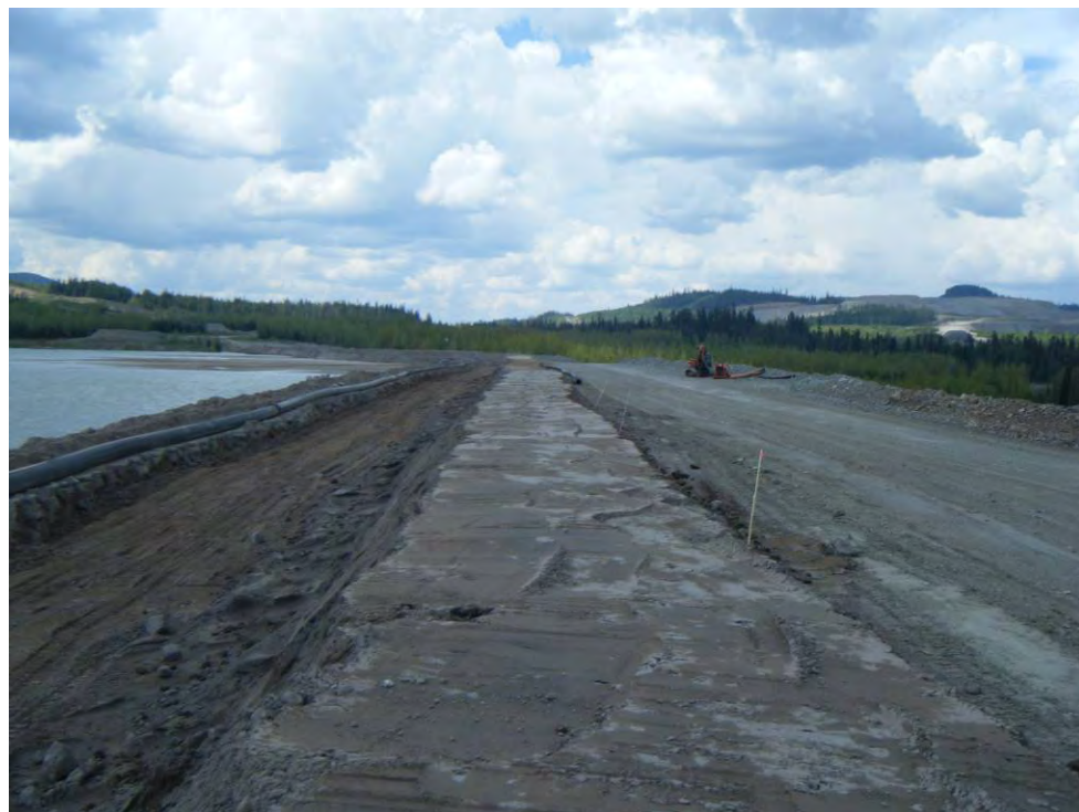
Photo 13: Looking northwest along the perimeter embankment (Zones U, S, F, T and C from left to right).
