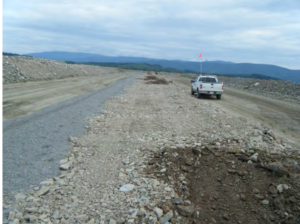
Photo 30: Approved Zone T material (South Embankment). Note the freshly removed unacceptable fill – see Photo 29).
