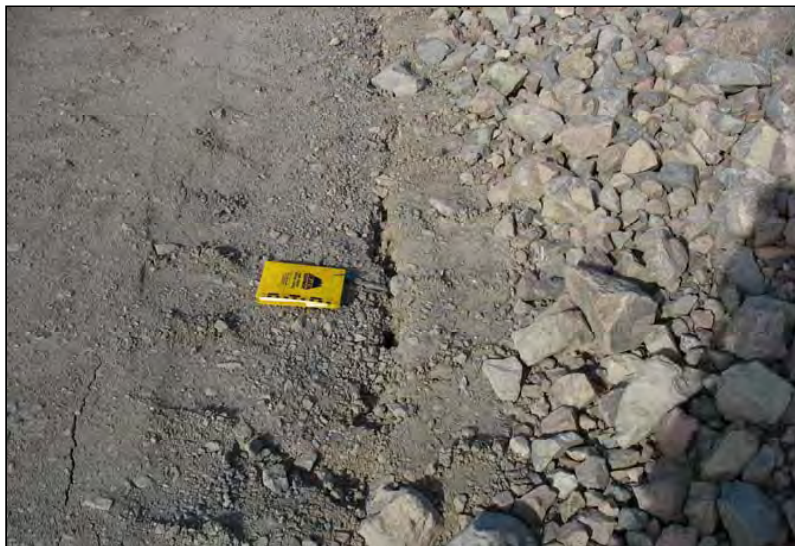
PHOTO 6 – Tension Crack at the Perimeter Embankment.
