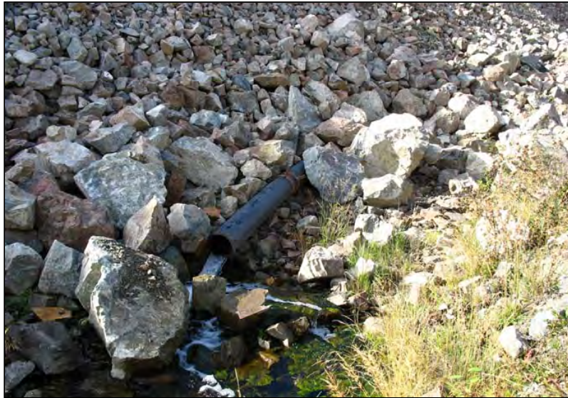
PHOTO 3 – Perimeter Embankment Toe Drain Flow.
