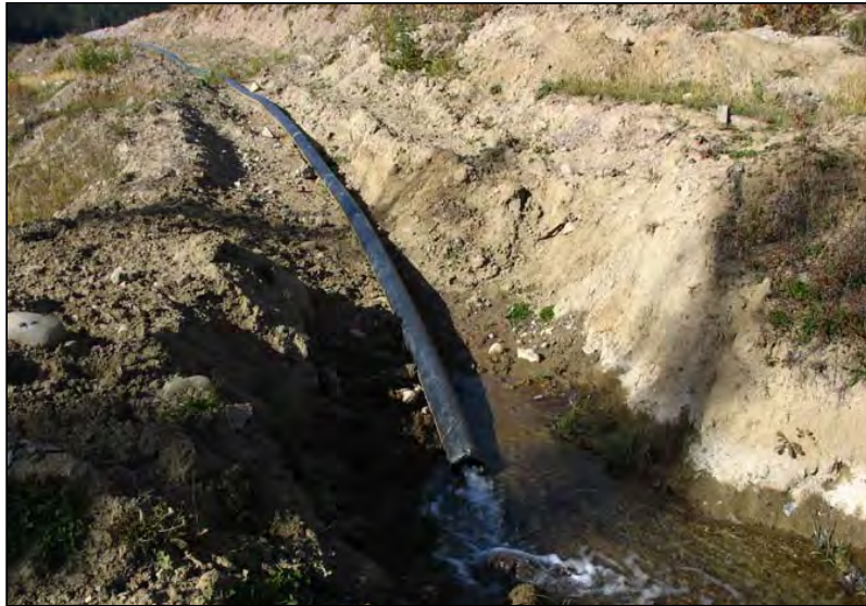
PHOTO 15 – South Embankment Upstream Toe Drain flow.
