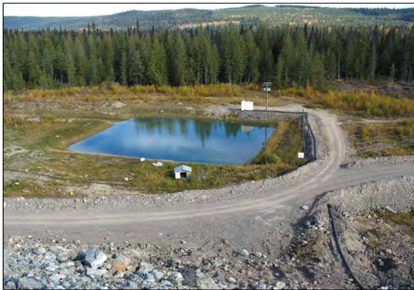
PHOTO 2 – Perimeter Embankment Seepage Collection and Recycle Pond.
