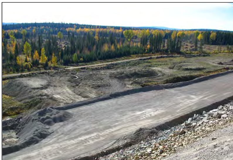
PHOTO 10 – Main Embankment Buttress.
