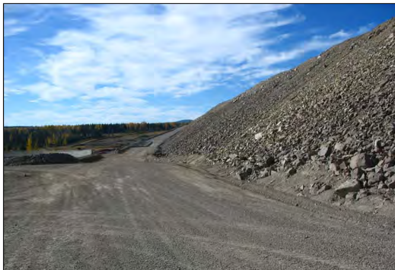
PHOTO 8 – Downstream Slope of Main Embankment.
