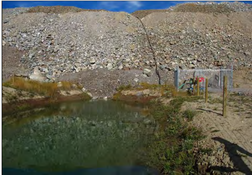
PHOTO 14 – South Embankment Seepage Collection and Recycle Pond.
