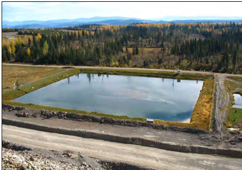
PHOTO 9 – Main Embankment Seepage Collection and Recycle Pond.
